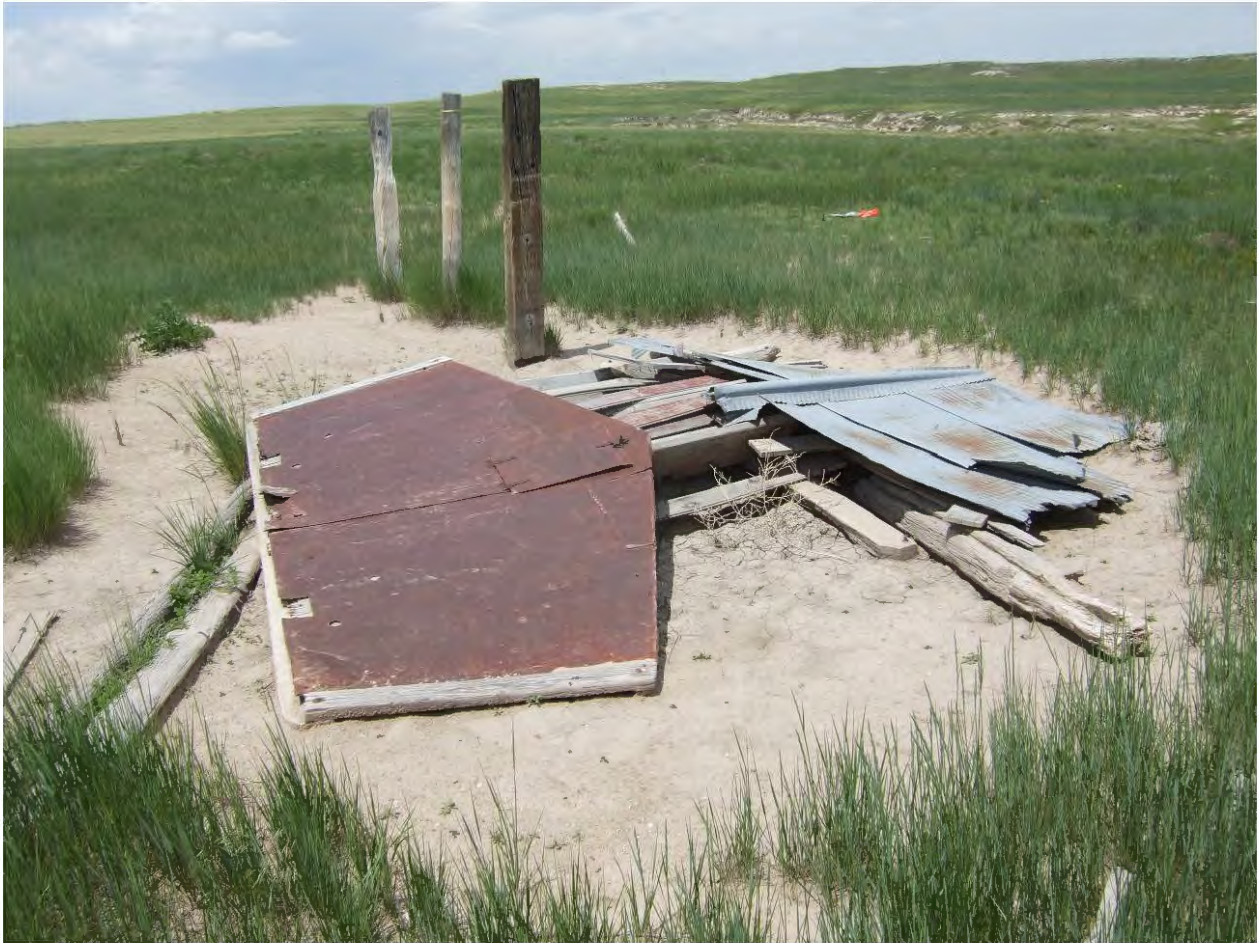
Figure 30. Overview looking west at collapsed shed and standing posts in the 5WL7682 site area.
