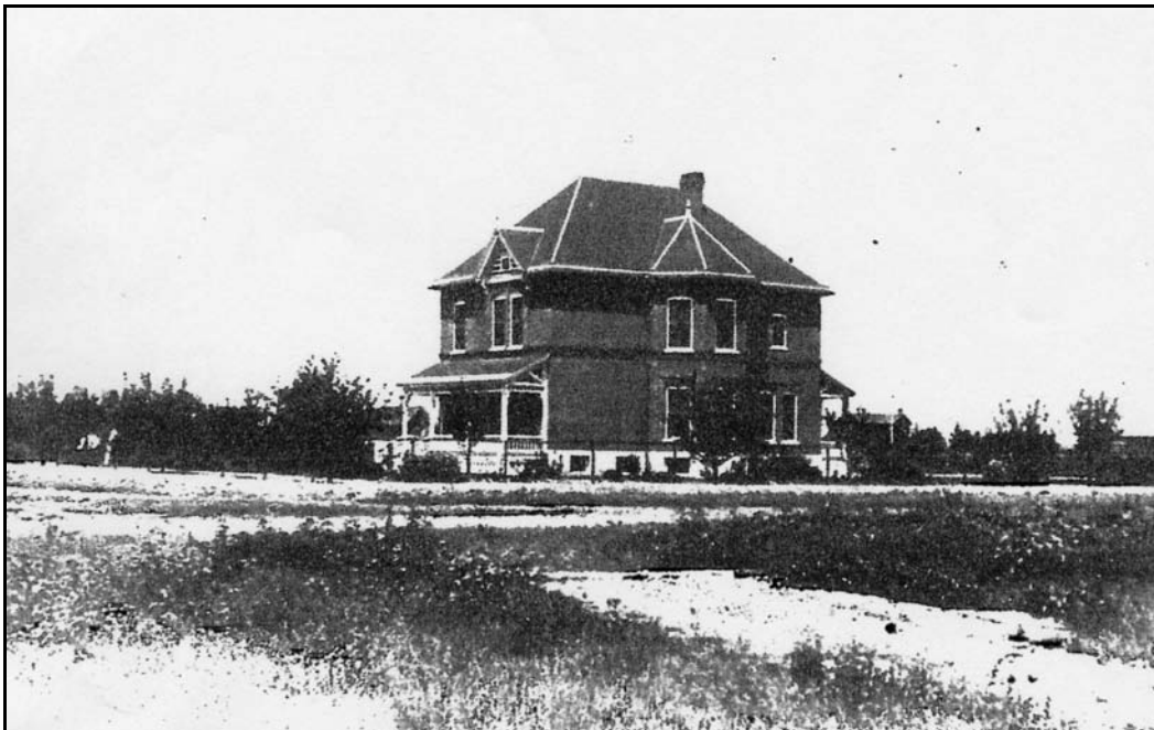
Figure 1. Early, undated, photograph of the A.J. Eaton House (view northeast). SOURCE: Eaton Area Historical Society, photographic collection.
