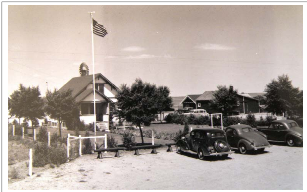
H10. View of the complex (c. 1940) showing growth of trees and shrubs.
