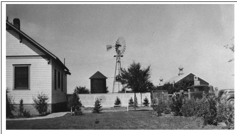
H8. Slightly later (c.1937-1938) photo of the headquarters showing the house/office, granary, and shop/barn. The house has been painted white. The plantings are very young.
