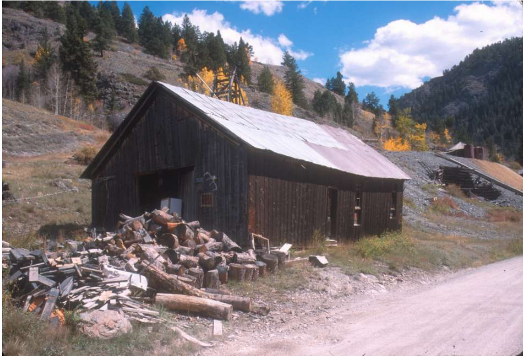
HP 22. Southwestern and northwestern sides of Building 37, looking east-southeast, in 2001.
