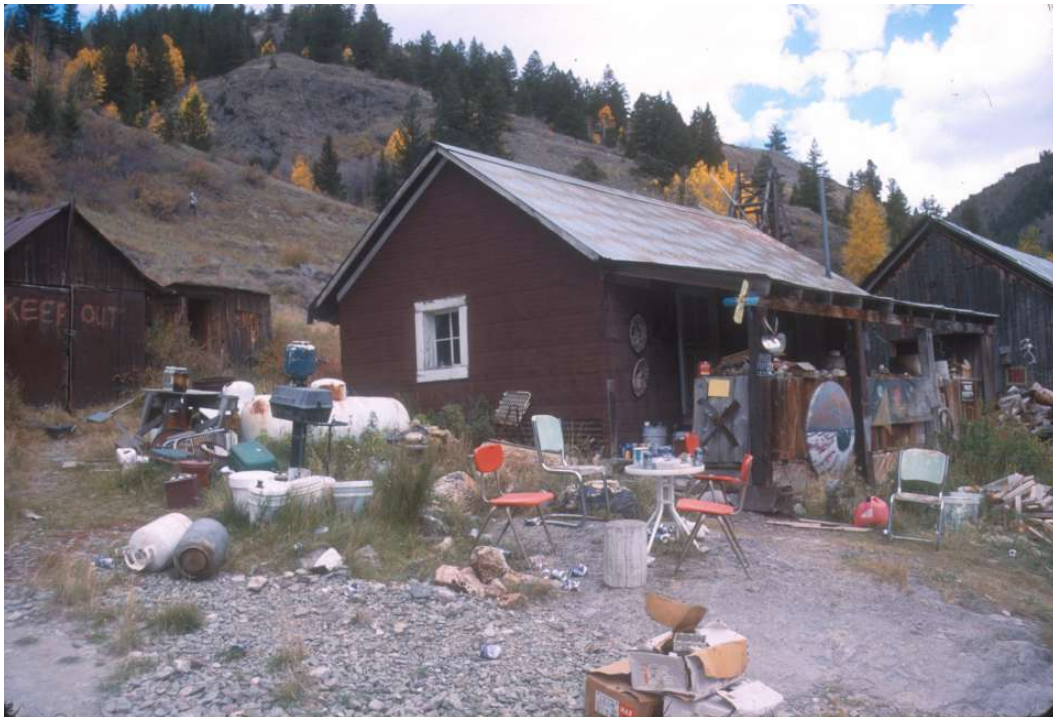
HP 23. 2001 photo of the southwestern and northwestern sides of residence (Building 38), looking east with removed Building 39 to left.
