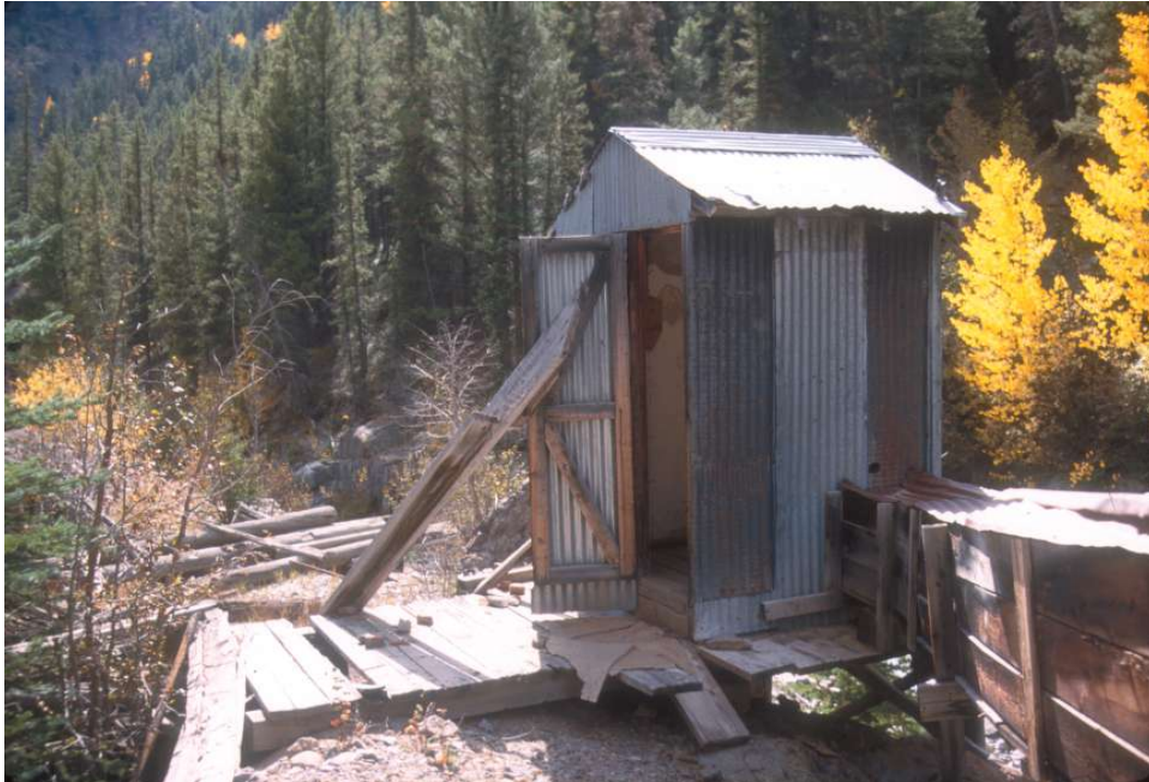
HP 12. 2001 photo of the small corrugated sheet metal shed (Building 13) with wooden boardwalk in front and water pipe in covered box to right. View is to the south. This building is now laying on its front side.
