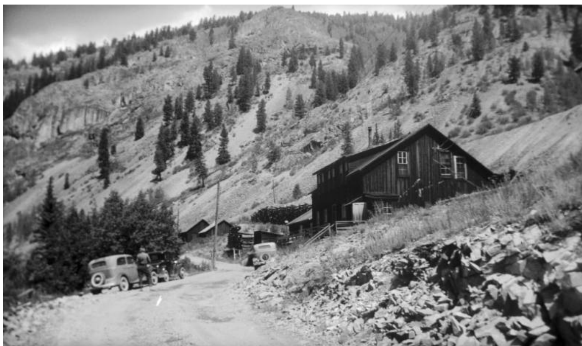
HP 7. Looking northwest at the boarding house (Building 16) with the residence (Building 15) partly visible behind, and Buildings 37 and 38 in the distance. Photo taken in 1942 by Muriel Sibell Wolle. DPL photo X-3467
