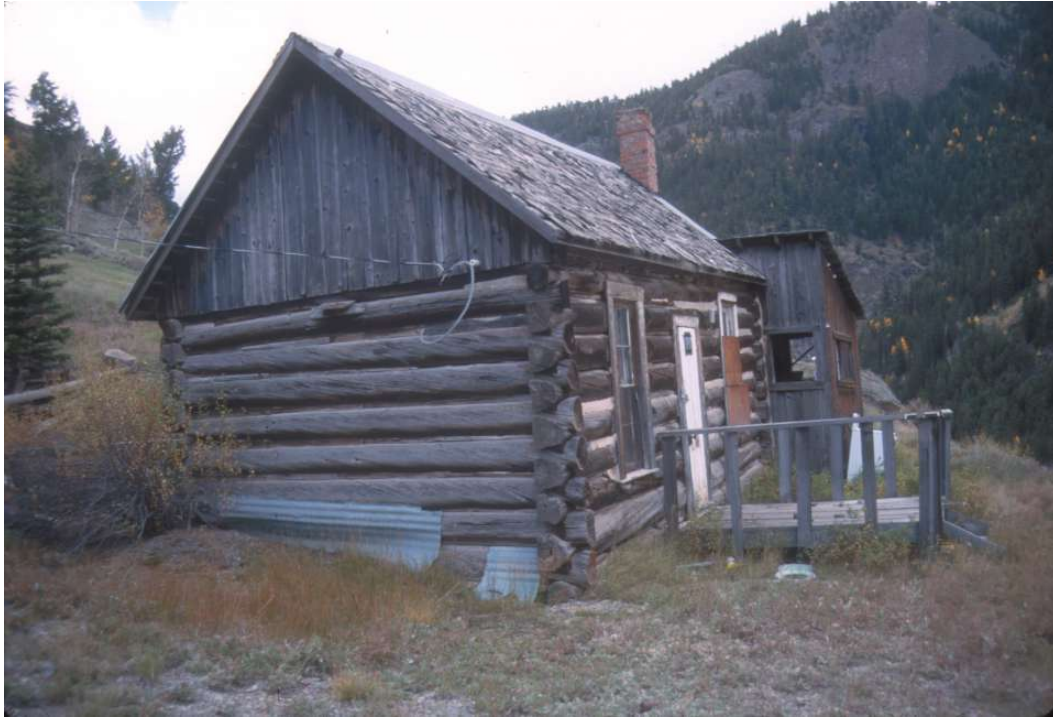
HP 18. Southwestern and northwestern sides of the log cabin residence (Building 17), looking southeast in 2001.
