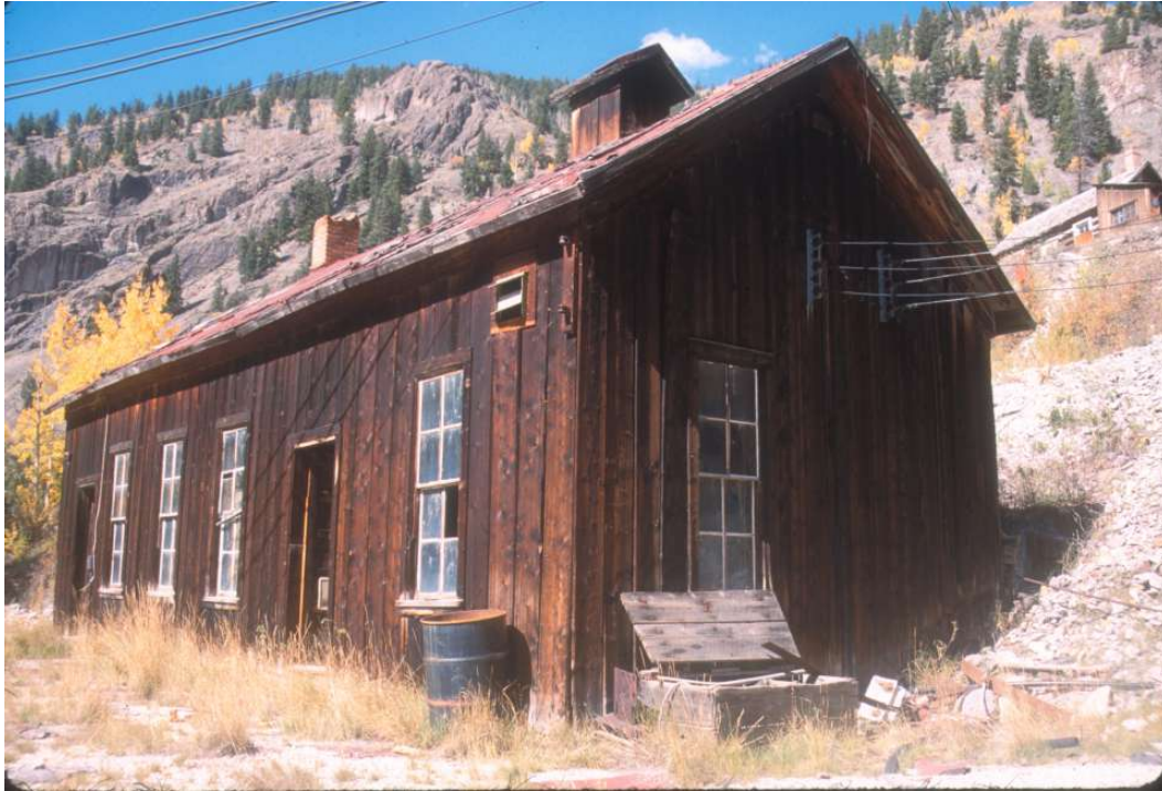
HP 8. 2001 photo of the southeastern and southwestern sides of the assay office (Building 8). View is to the north.
