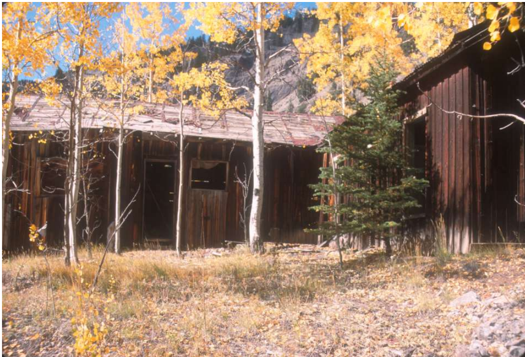
HP 9. 2001 photo of the southeastern side of the southwestern wing and southwestern side of the southeastern wing of the office (Building 9). View is to the northwest.
