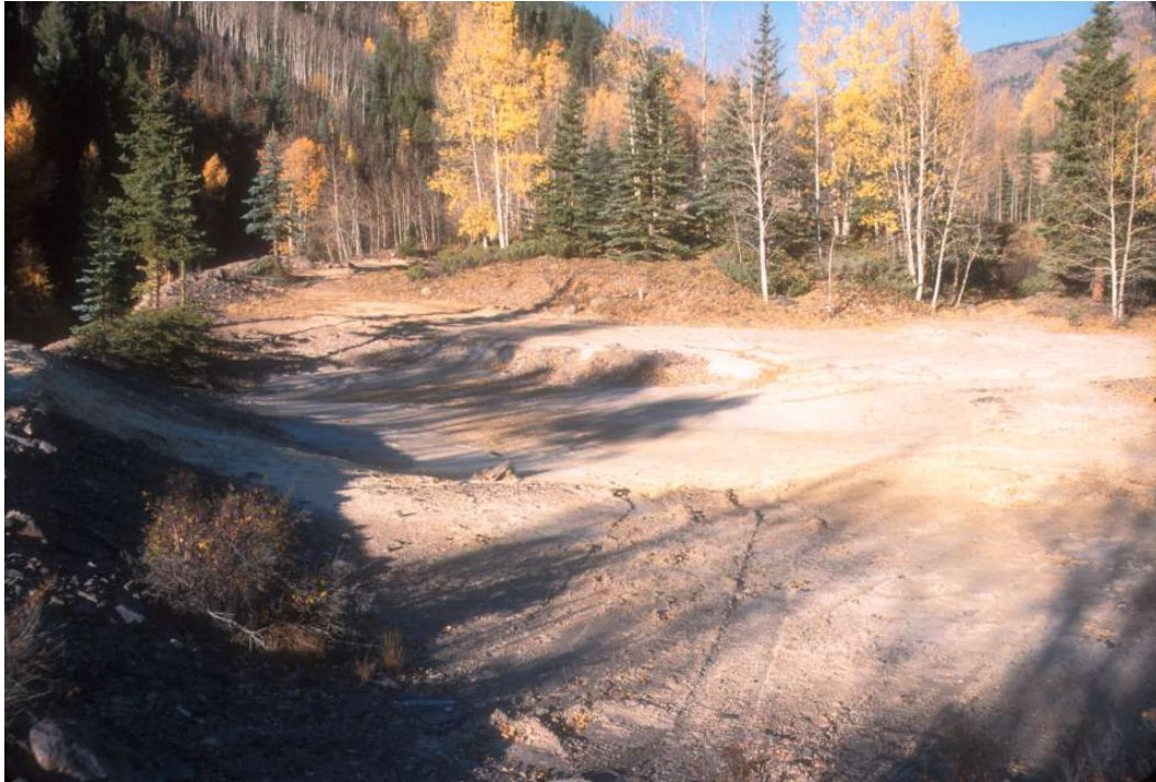
HP 28. Tailings Impoundment 4, looking west in 2001. This area was remediated and revegetated in 2009.
