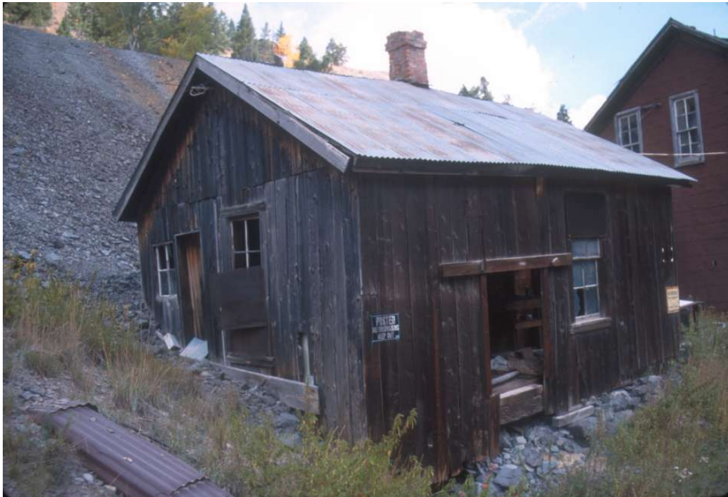
HP 16. 2001 photo of the southwestern and northwestern sides of Building 15, looking east.
