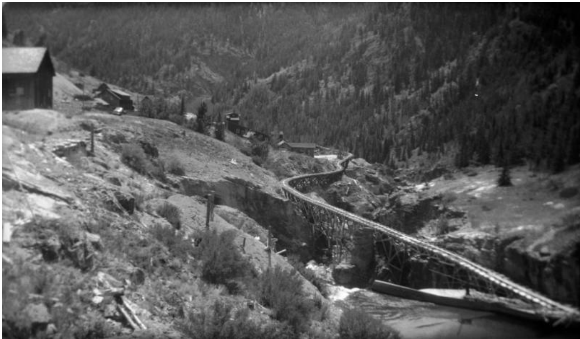
HP 5. The flume (Feature 2) winding southeastward down Henson Creek with the office (Building 9) just above the flume and the mill (Building 6) at center. At the far right is removed Building 36 with the boarding house (Building 16) in the distance. Photo taken in 1942 by Muriel Sibell Wolle. DPL photo X-3474
