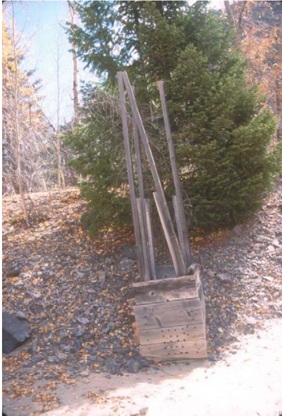
HP 14. Cribbed water drainage box (Feature 4) on east end of Tailings Impoundment 7 as it appeared in 2001, looking east-southeast. This was removed during mill tailings remediation in 2013.
