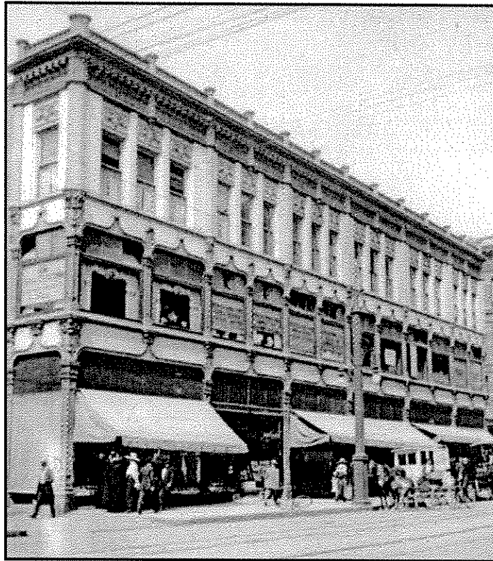
Figure 2. The 16 th Street side of the McClintock Building is shown here in about 1913. SOURCE: Denver Public Library, Western History and Genealogy Department, photographic collection, image X-18751.
