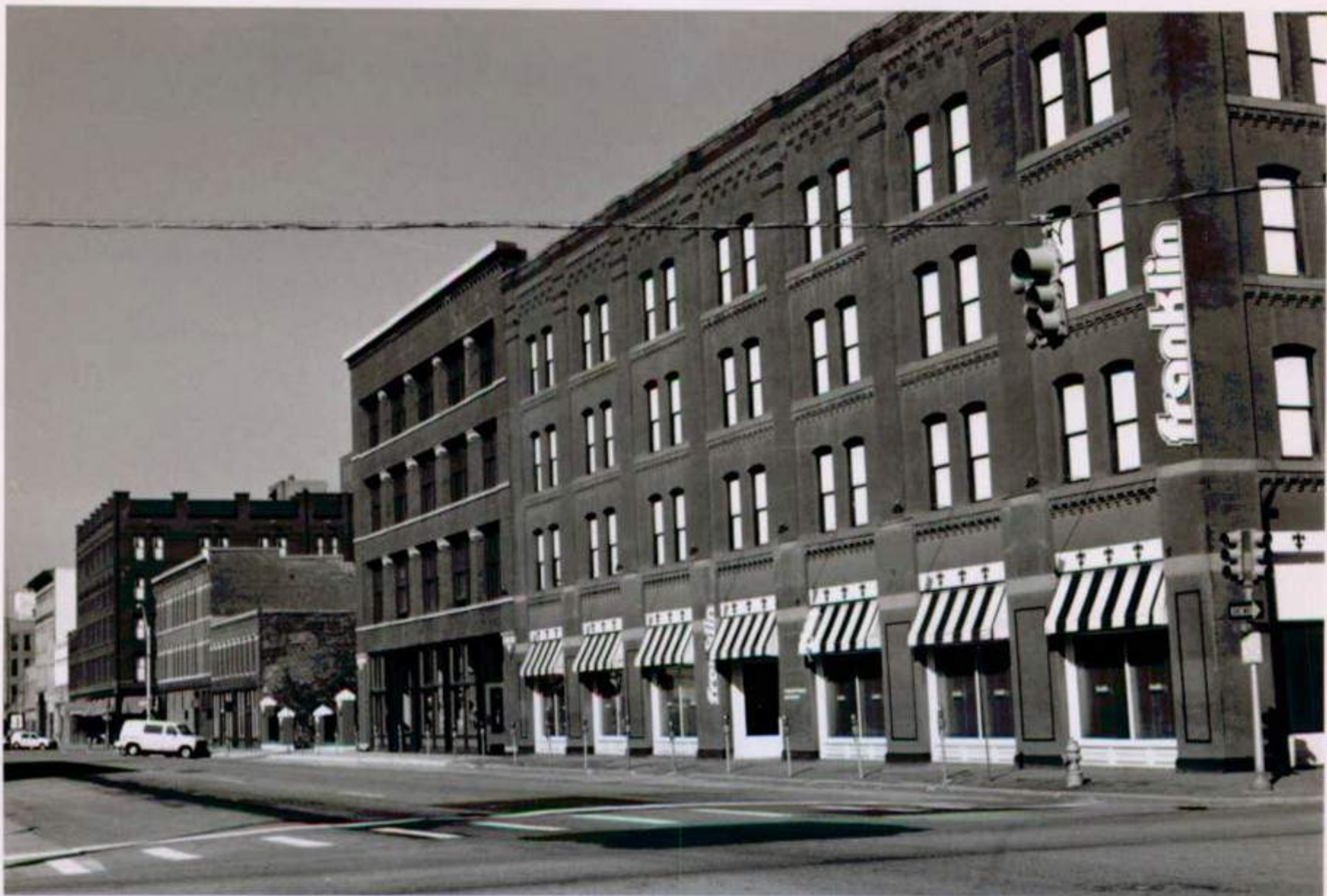
Lower Downtown Historic District #17 Denver, Colorado
