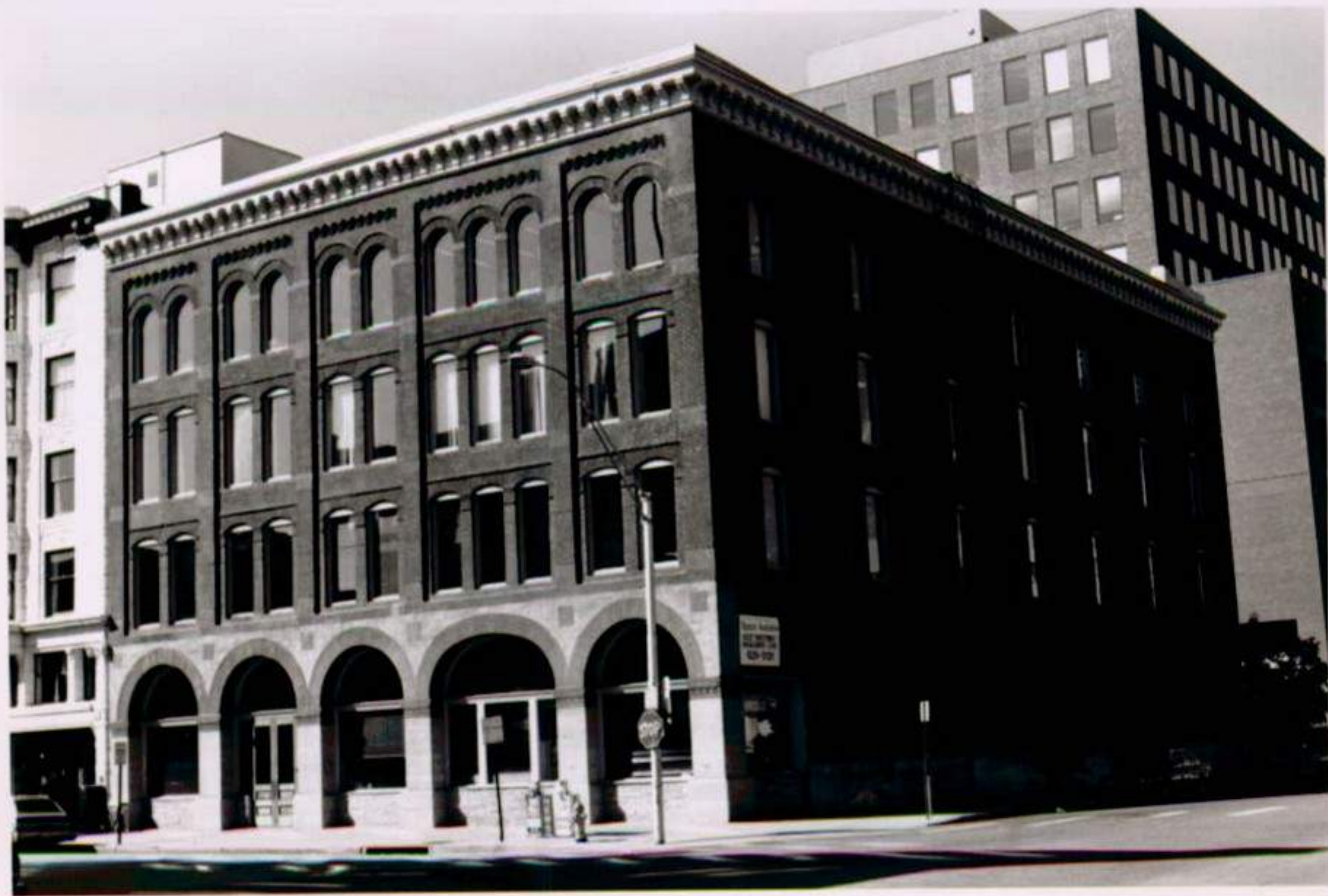
Lower Downtown Historic District #5 Denver, Colorado
