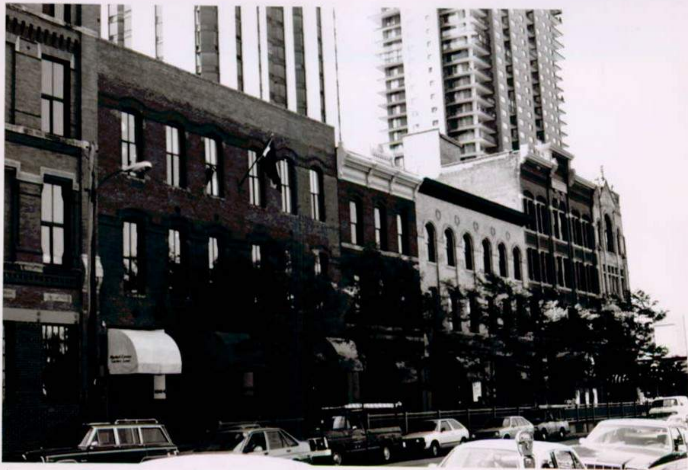
Lower Downtown Historic District #36 Denver, Colorado
