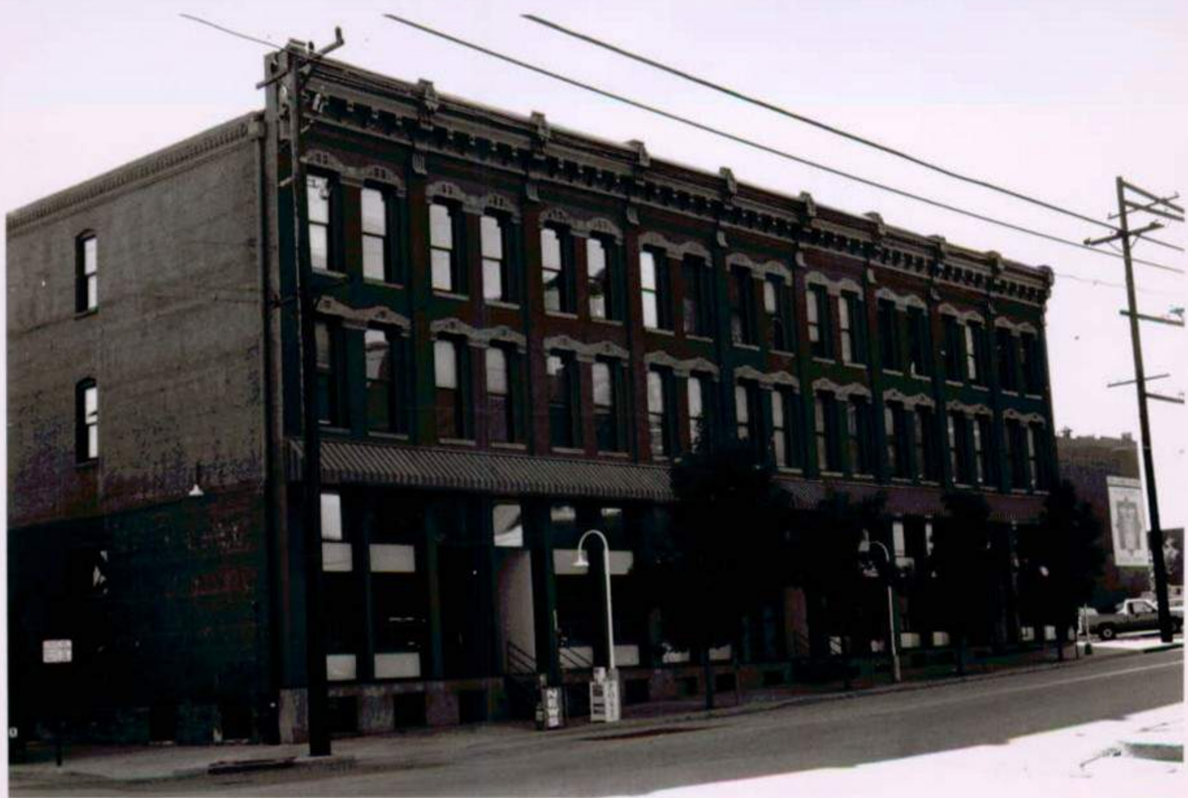
Lower Downtown Historic District #20 Denver, Colorado
