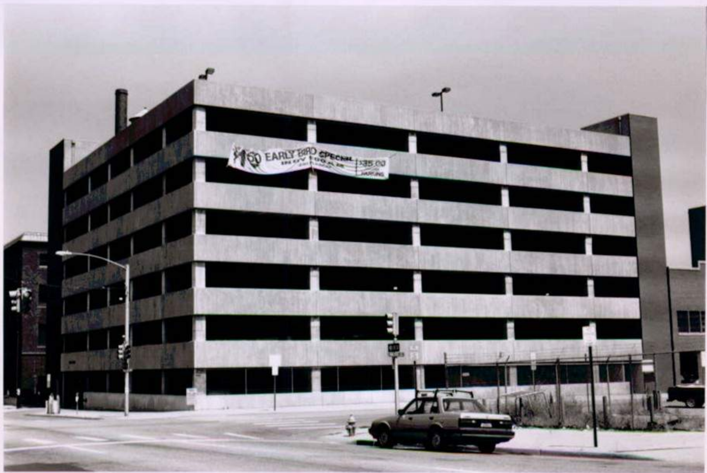
Lower Downtown Historic District #18 Denver, Colorado
