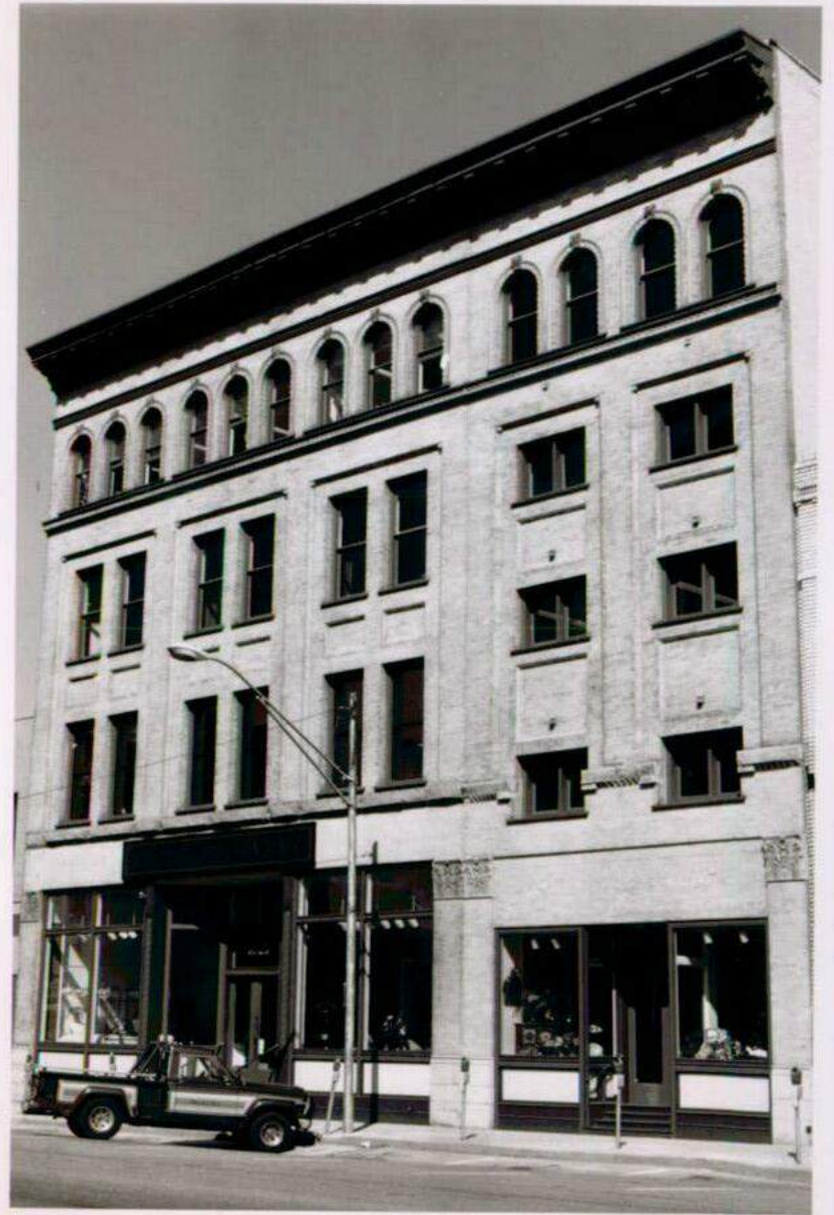
Lower Downtown Historic District #15 Denver, Colorado
