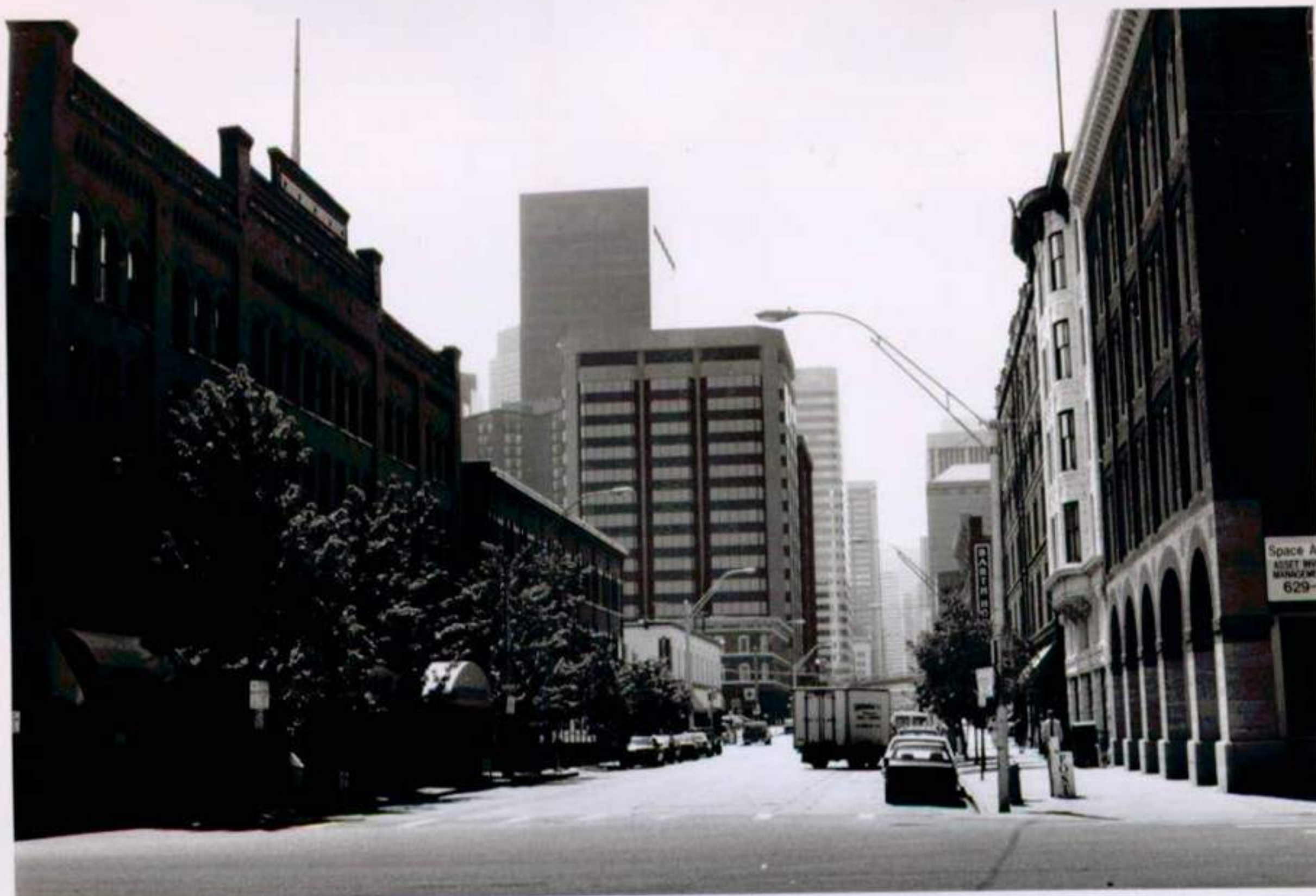
Lower Downtown Historic District #4 Denver, Colorado
