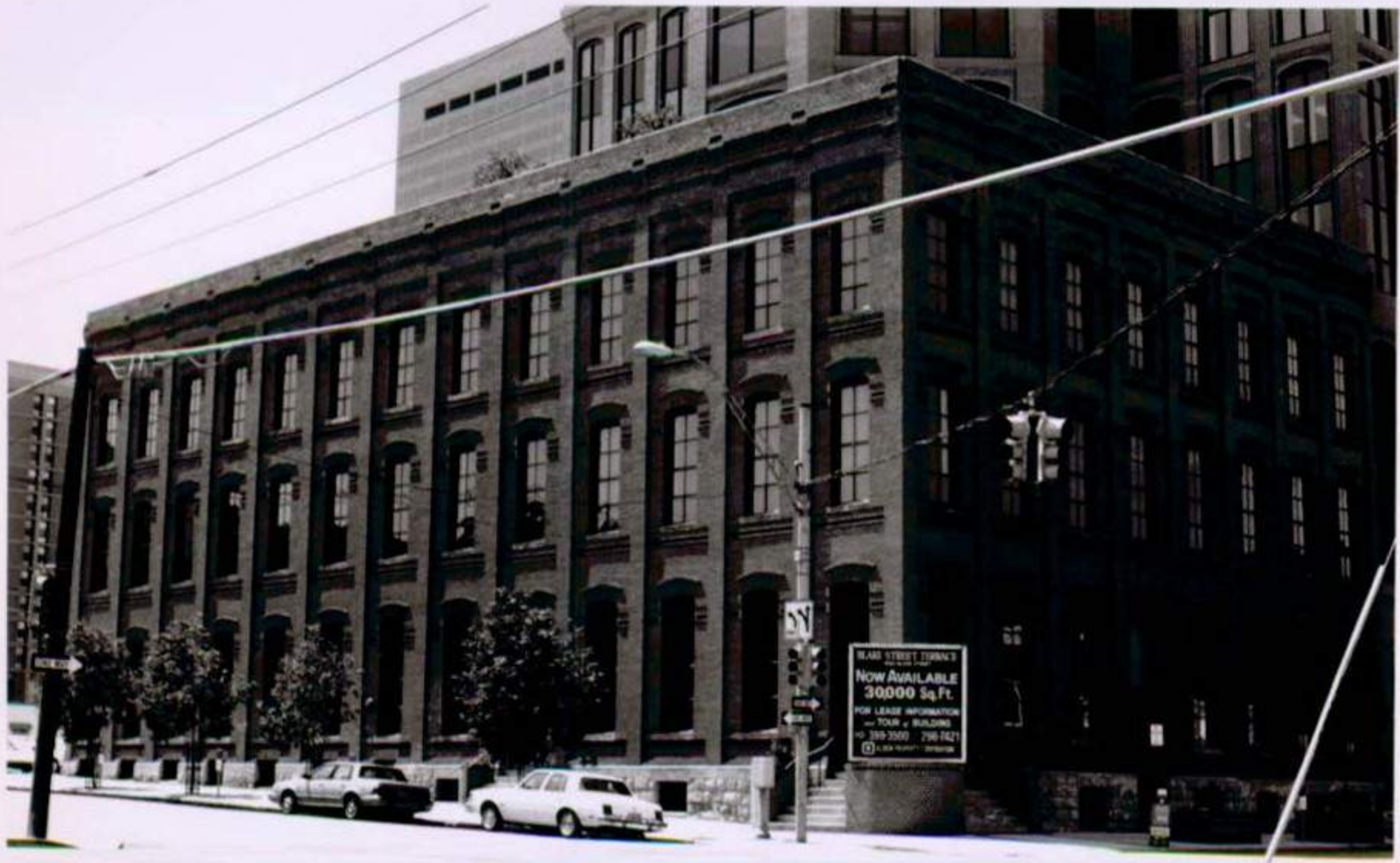
Lower Downtown Historic District #28 Denver, Colorado
