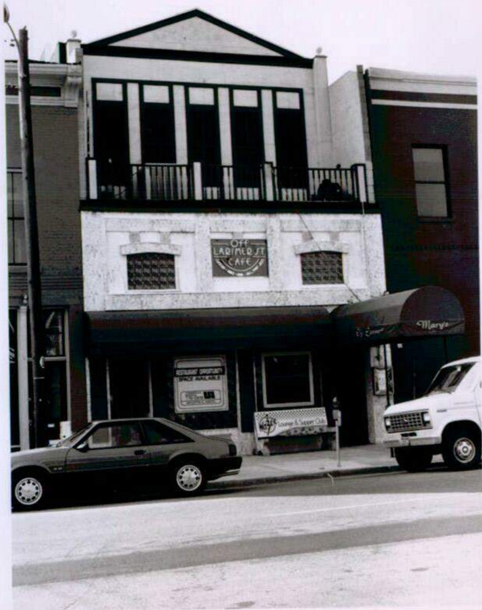
Lower Downtown Historic District #32 Denver, Colorado
