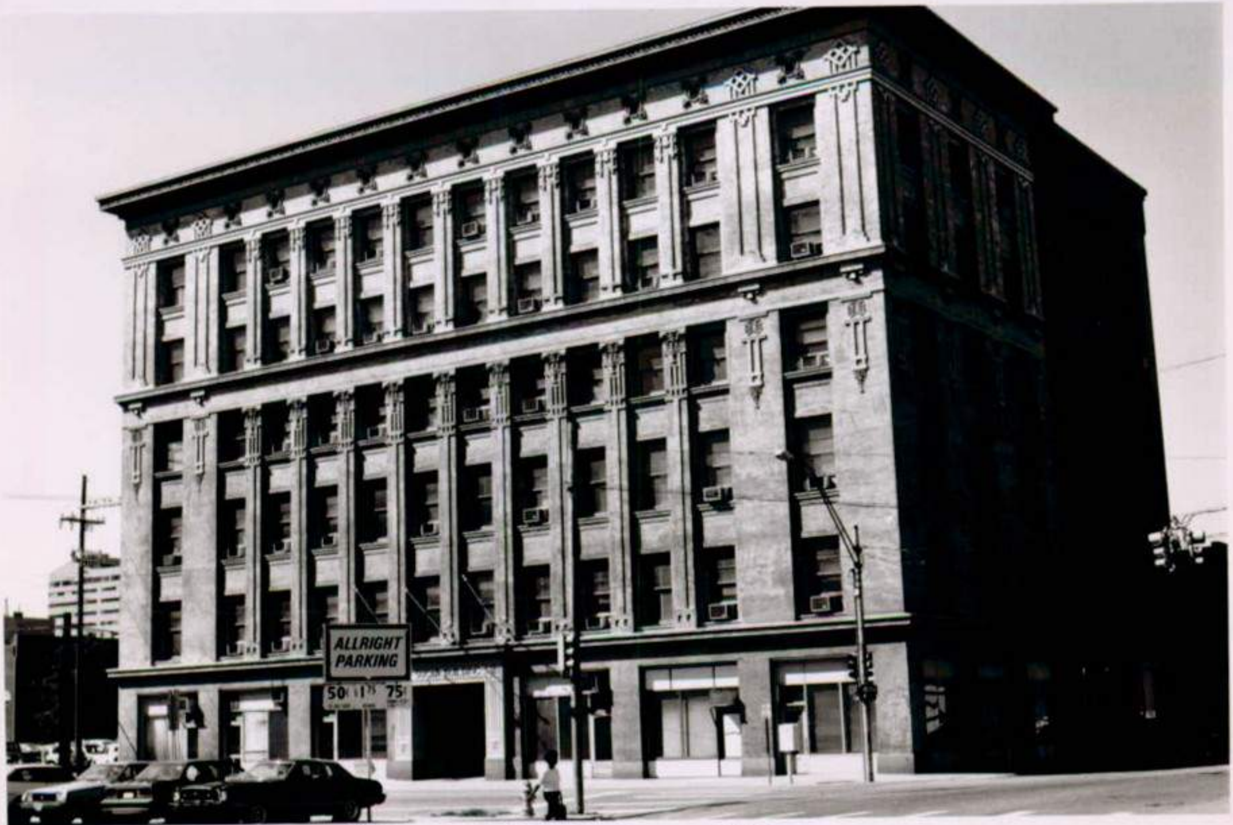
Lower Downtown Historic District #12 Denver, Colorado
