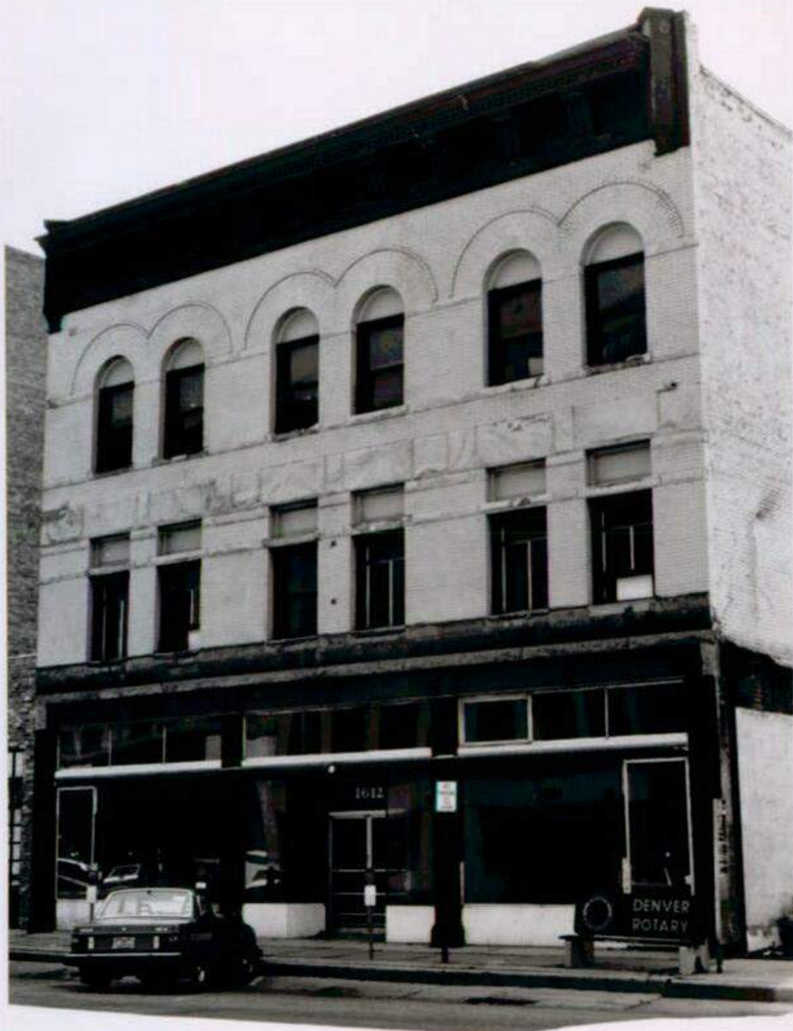
Lower Downtown Historic District #14 Denver, Colorado
