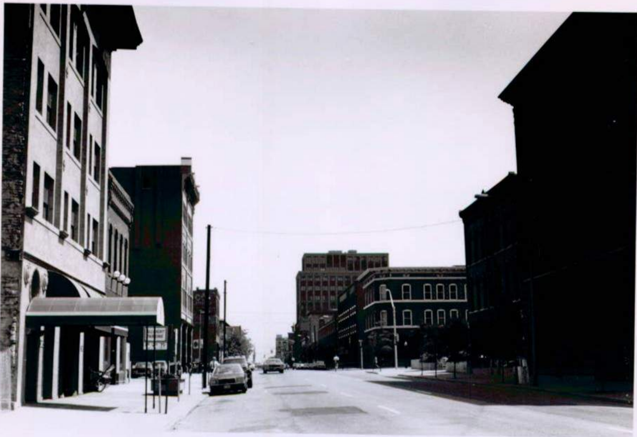
Lower Downtown Historic District #24 Denver, Colorado
