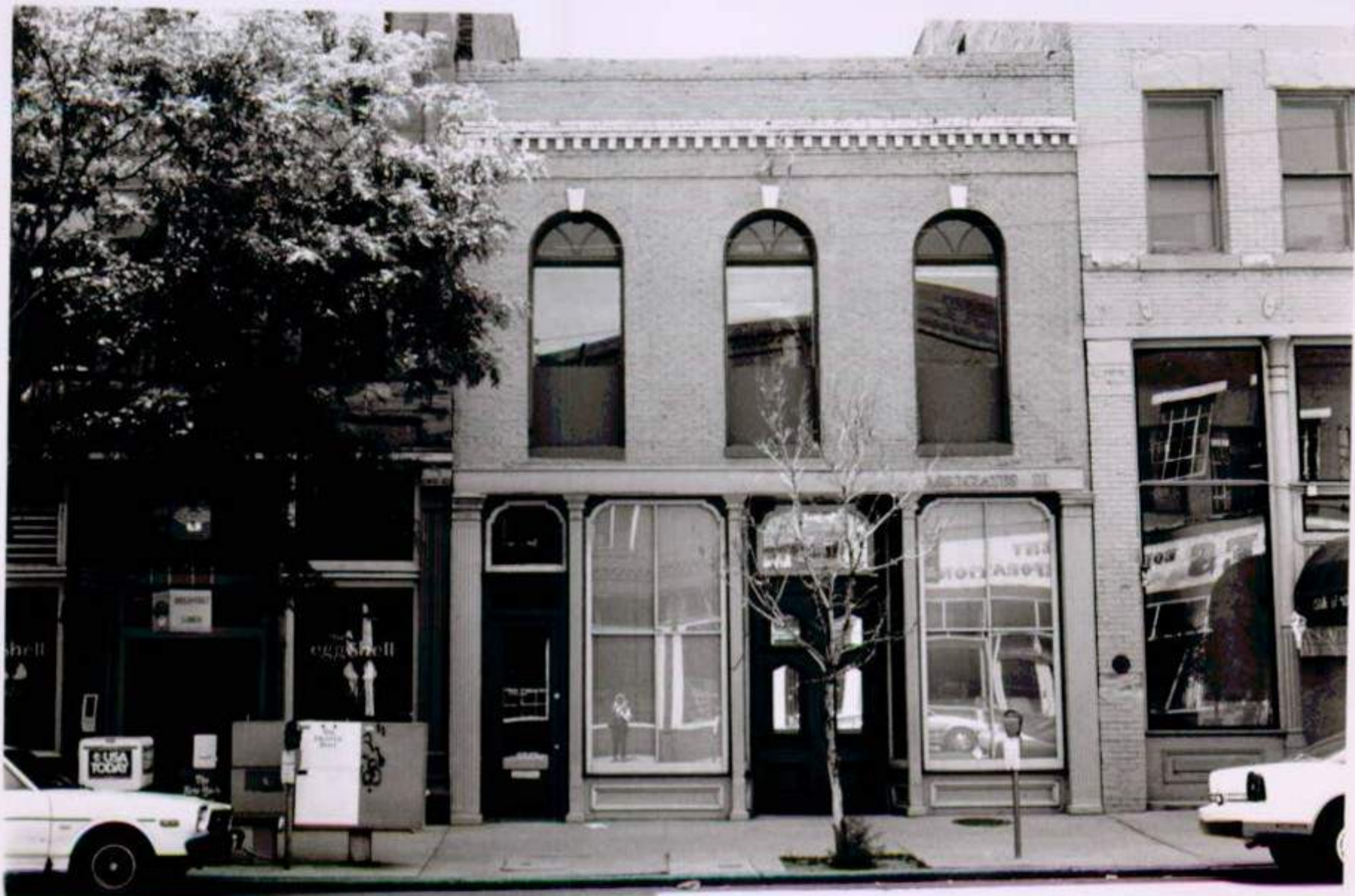
Lower Downtown Historic District #22 Denver, Colorado
