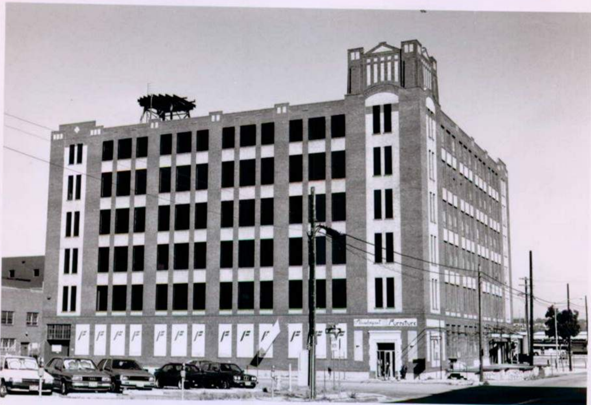
Lower Downtown Historic District #19 Denver, Colorado
