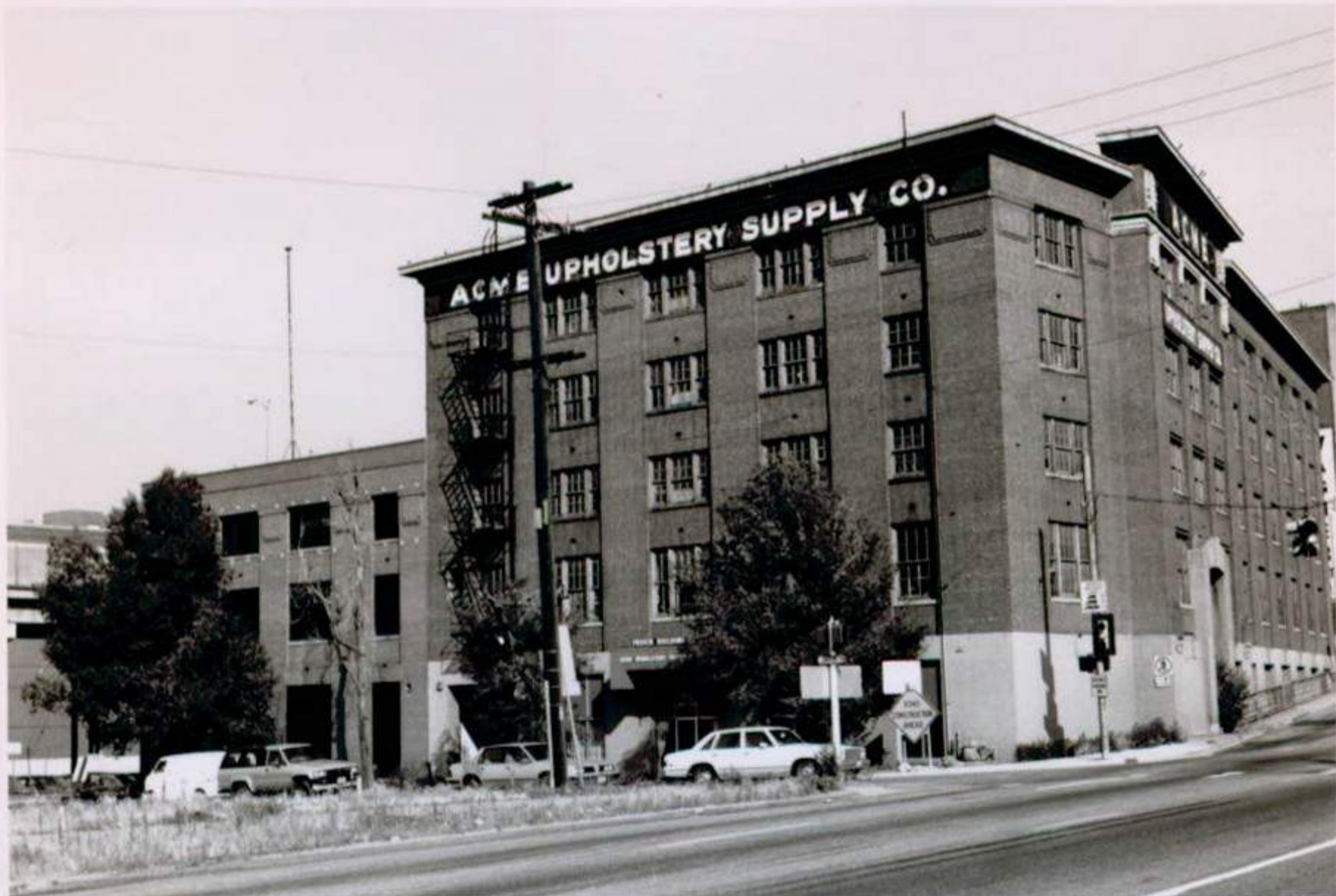
Lower Downtown Historic District #9 Denver, Colorado
