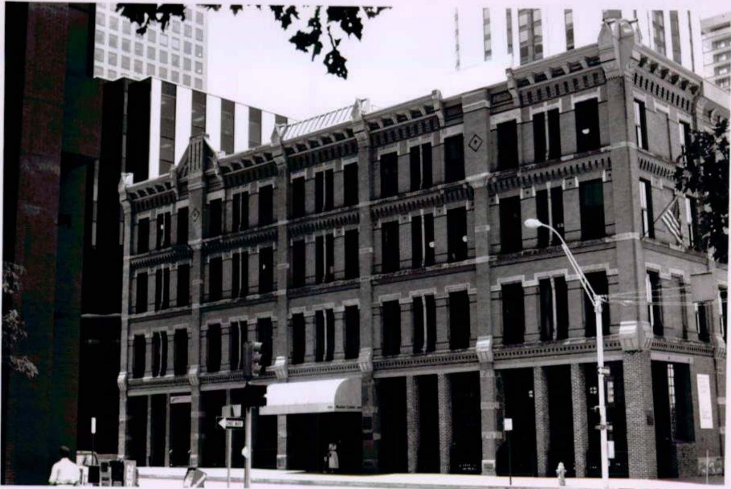
Lower Downtown Historic District #38 Denver, Colorado
