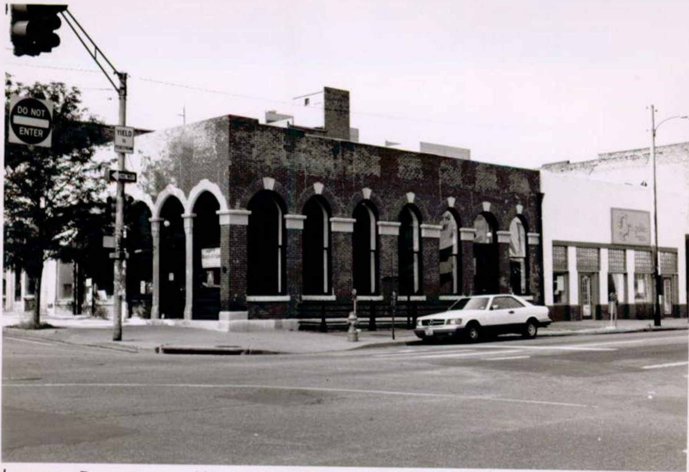
Lower Downtown Historic District #33 Denver, Colorado
