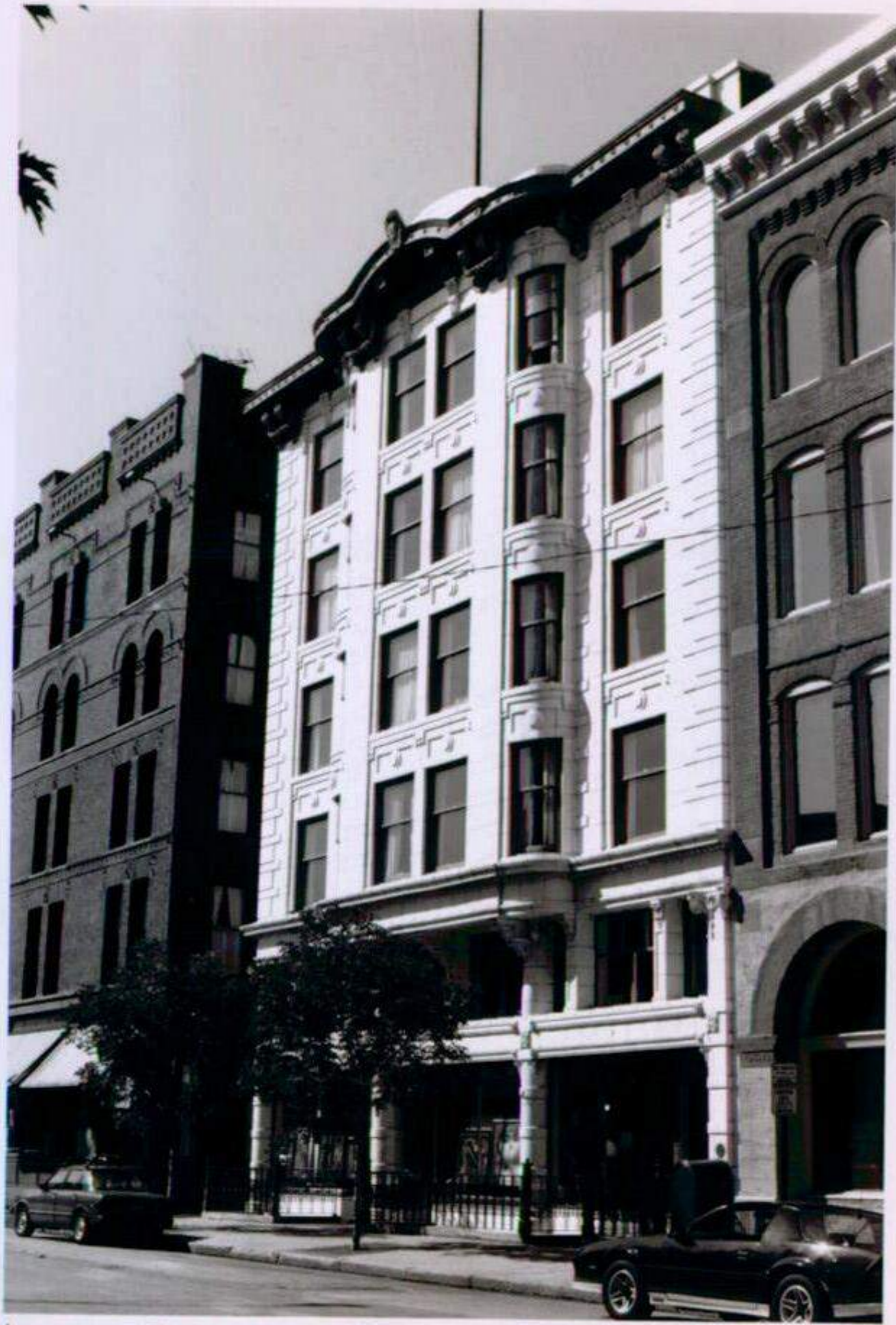
Lower Downtown Historic District #7 Denver, Colorado
