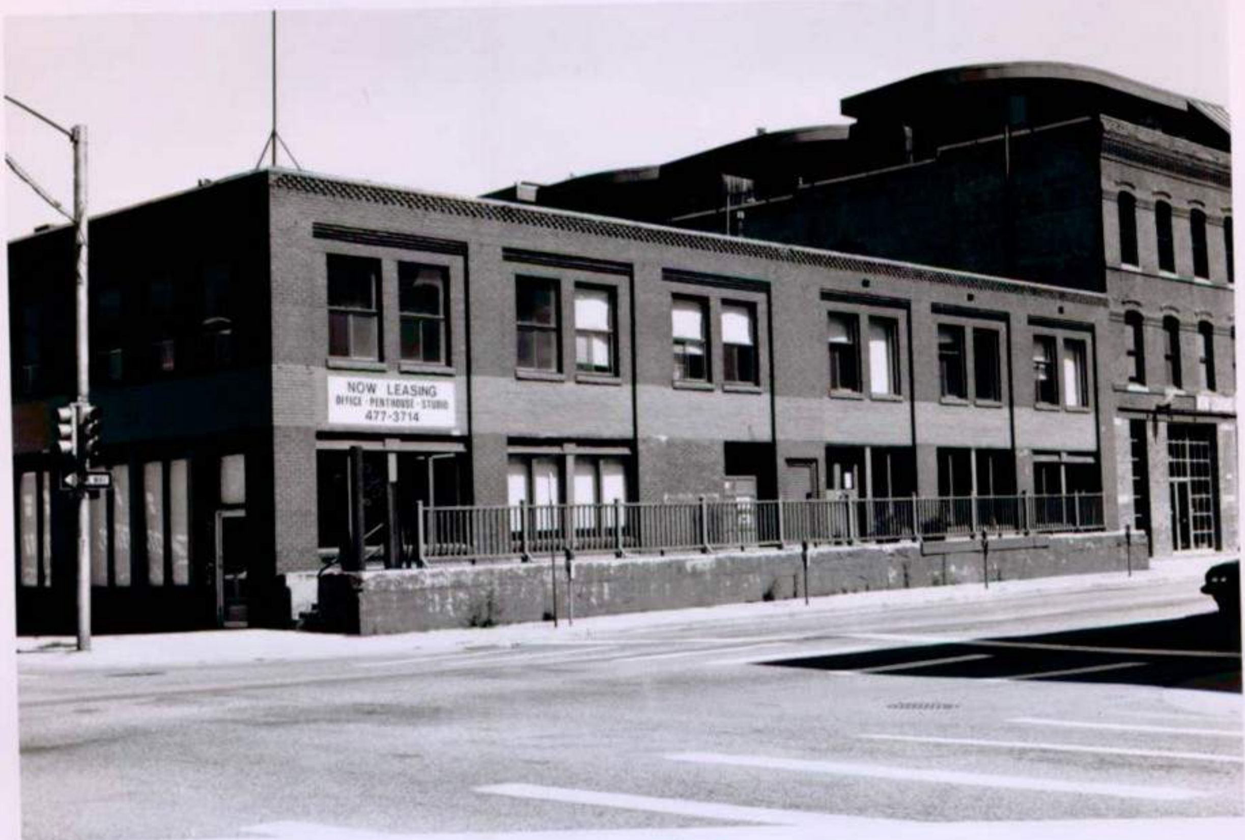
Lower Downtown Historic District #27 Denver, Colorado
