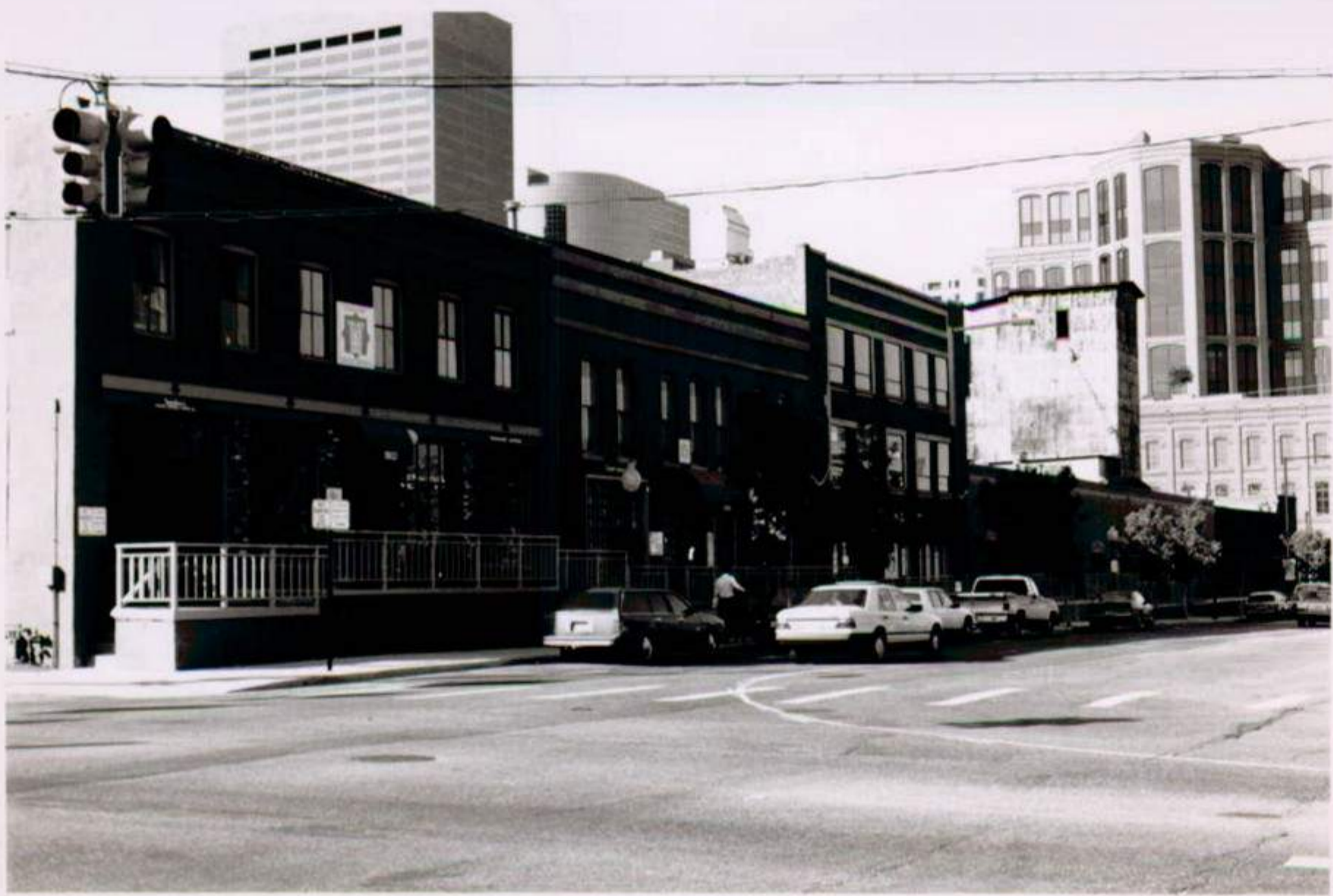
Lower Downtown Historic District #30 Denver, Colorado
