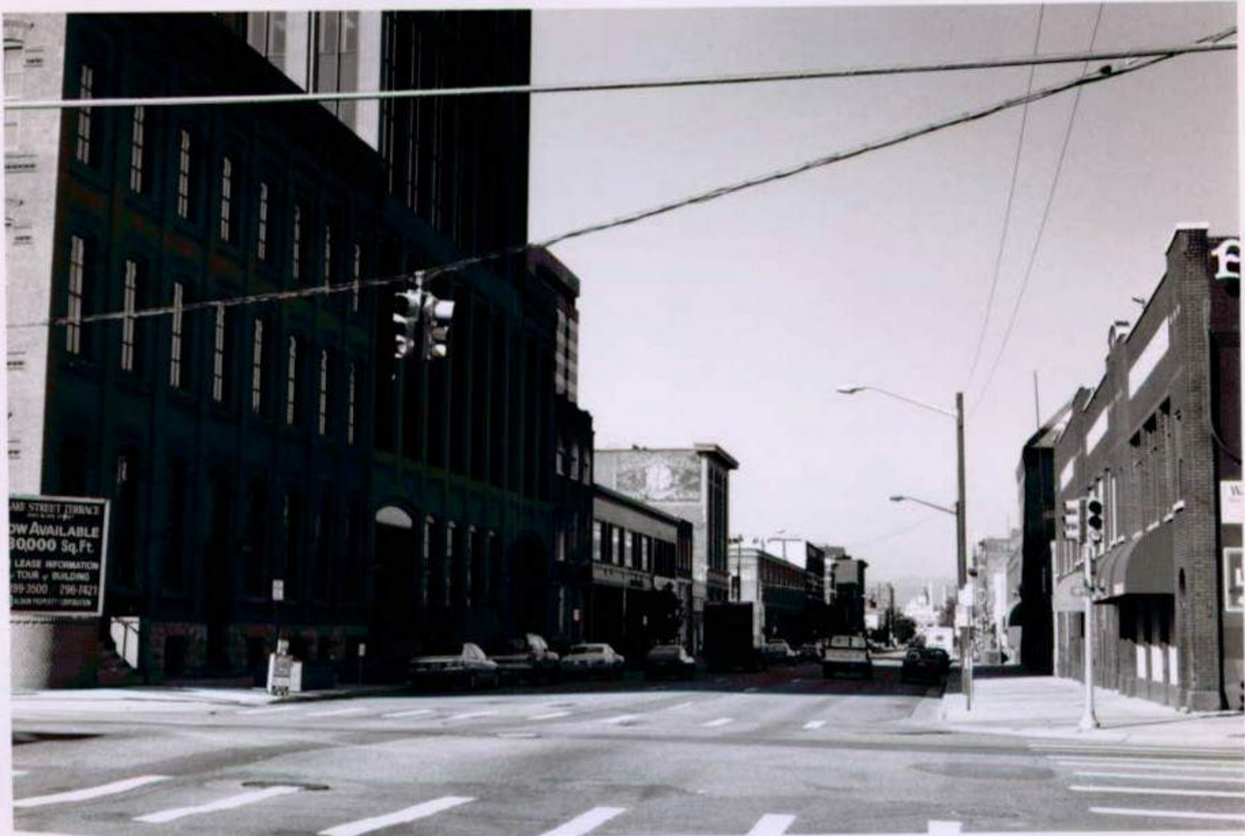
Lower Downtown Historic District #29 Denver, Colorado
