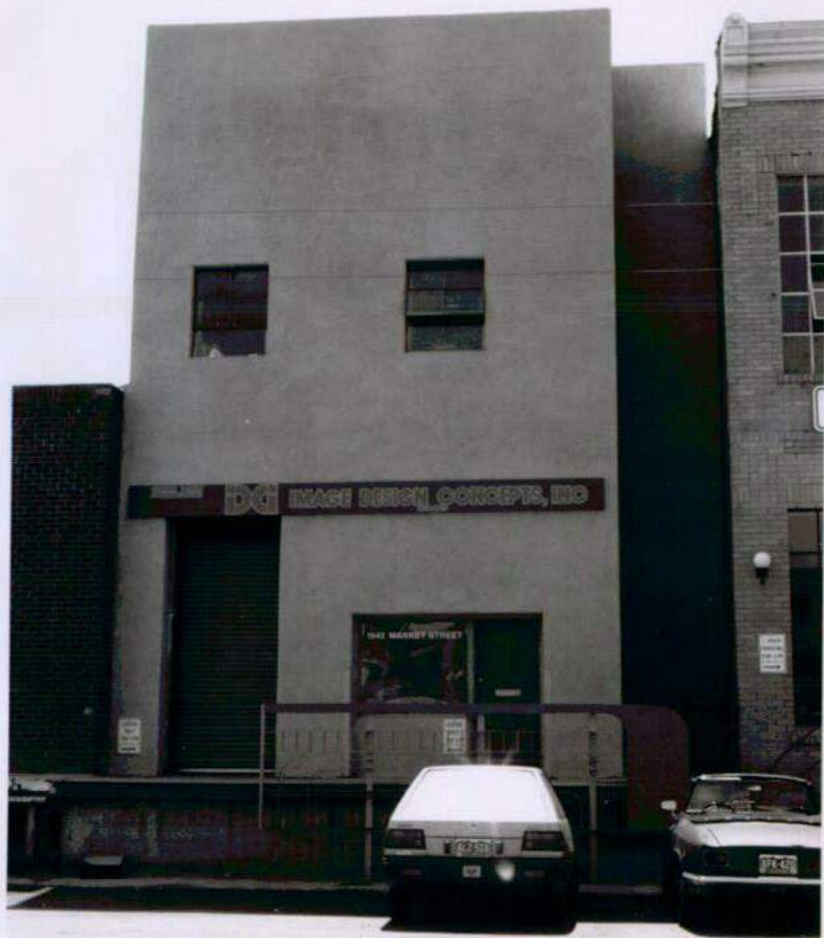
Lower Downtown Historic District #39 Denver, Colorado
