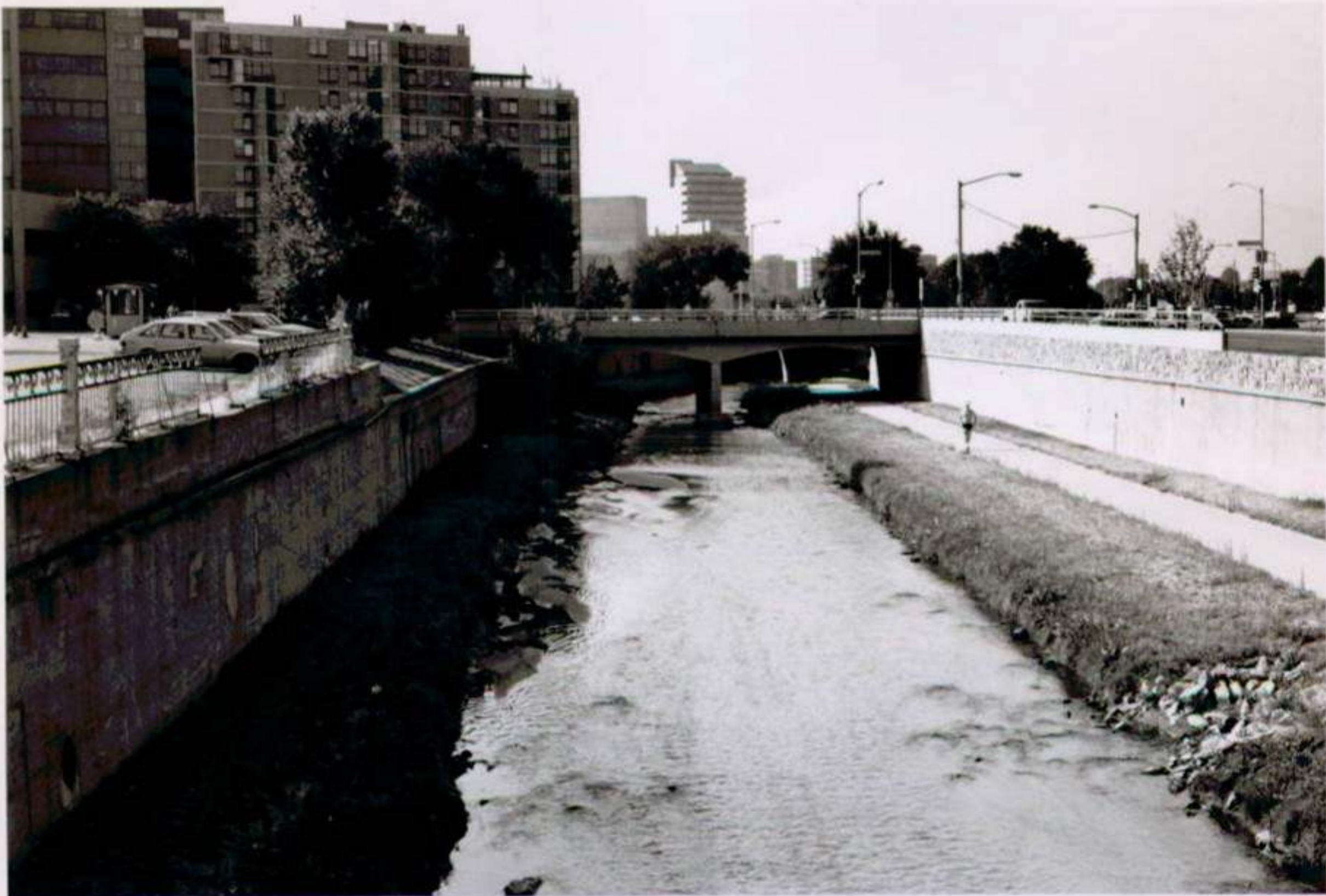
Lower Downtown Historic District #31 Denver, Colorado
