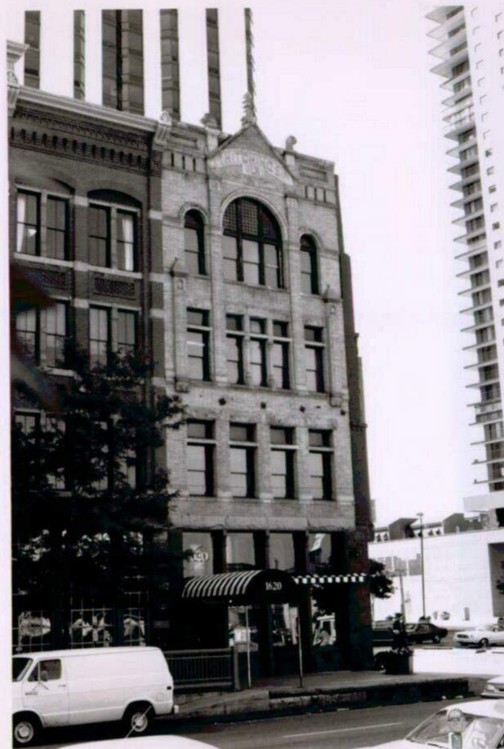
Lower Downtown Historic District #35 Denver, Colorado
