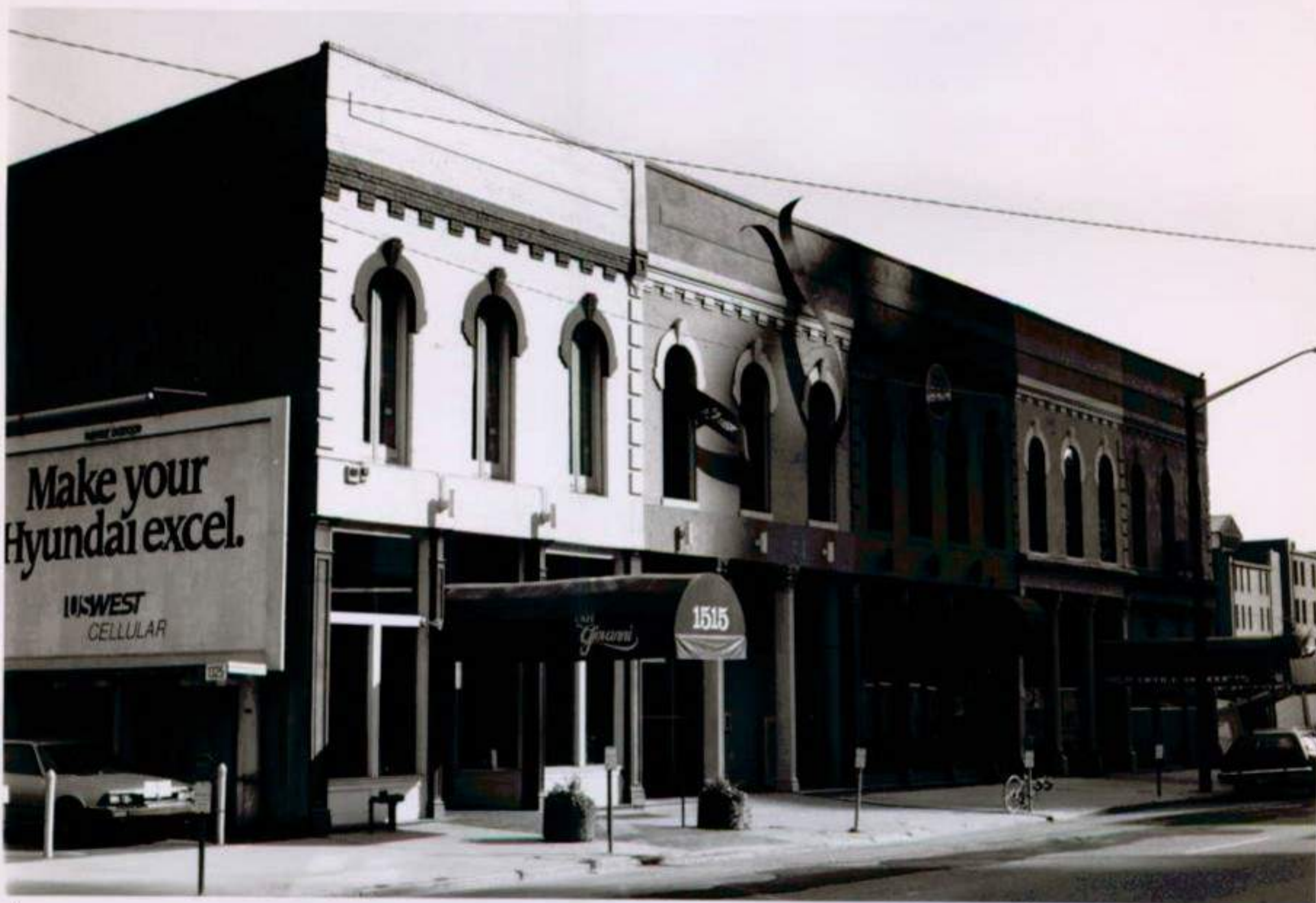
Lower Downtown Historic District #34 Denver, Colorado
