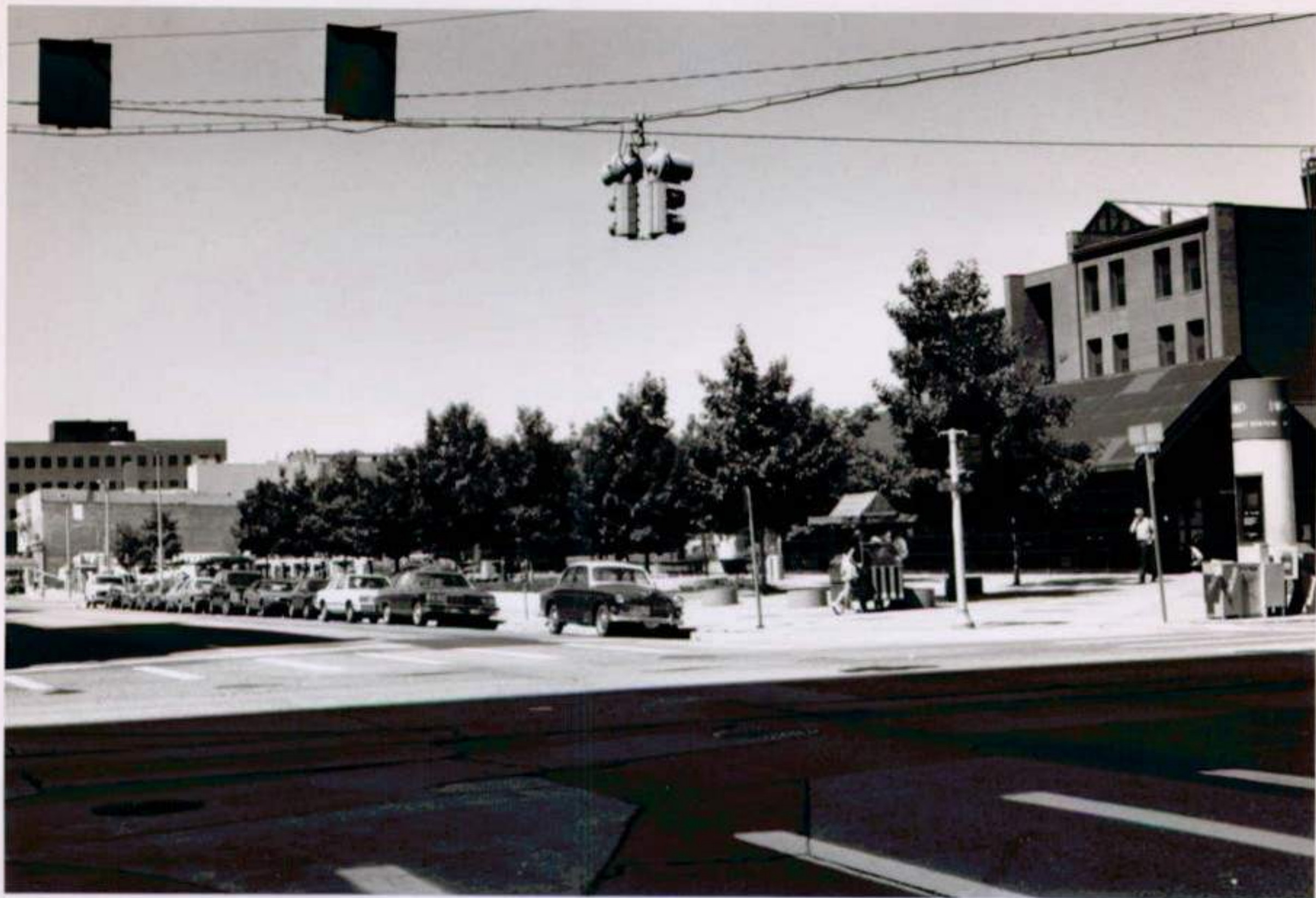
Lower Downtown Historic District #37 Denver, Colorado
