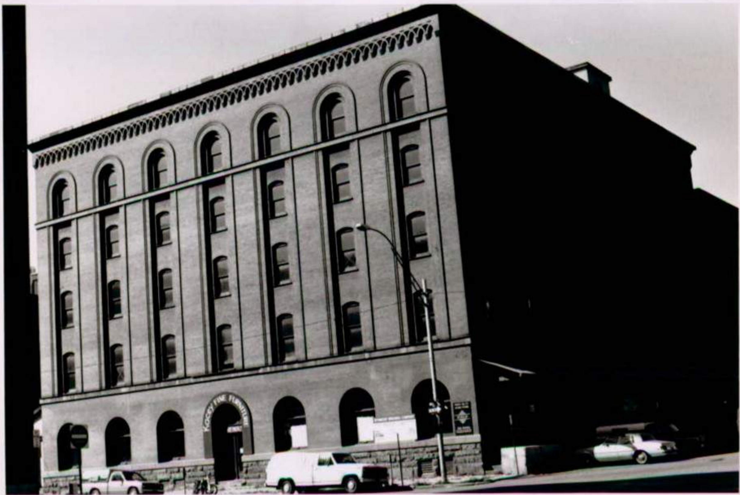
Lower Downtown Historic District #8 Denver, Colorado
