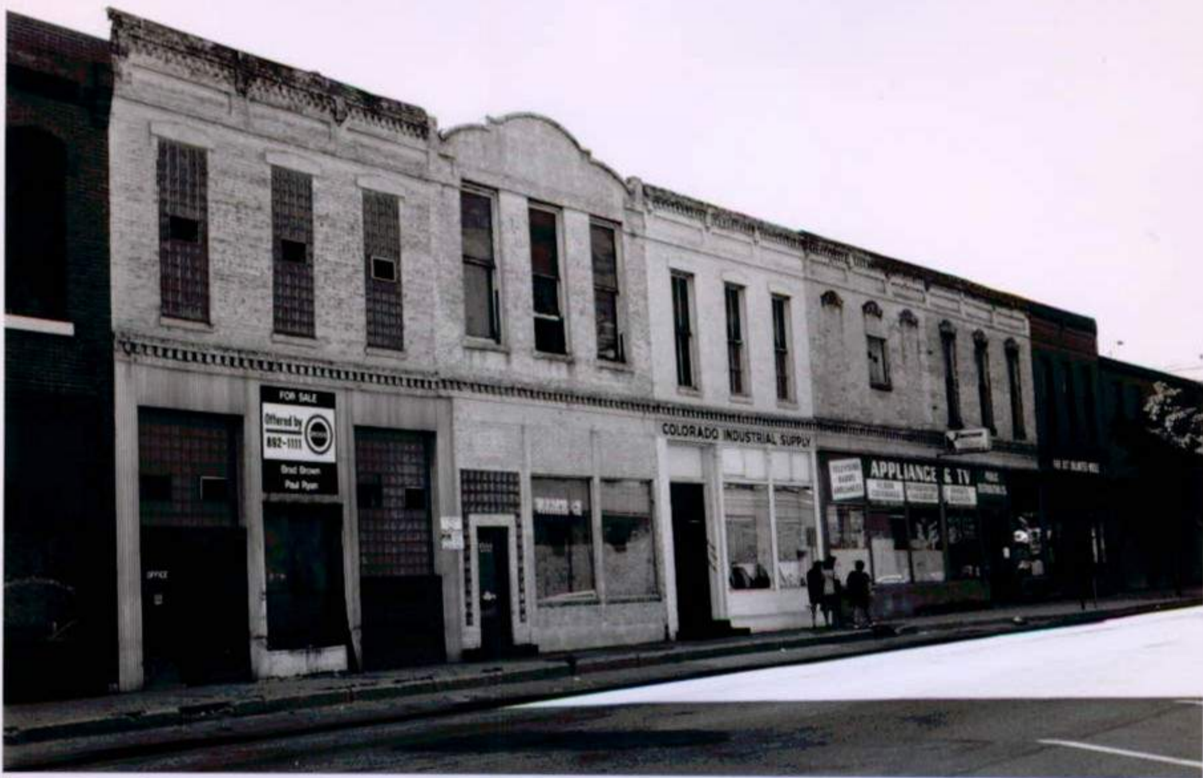
Lower Downtown Historic District #11 Denver, Colorado
