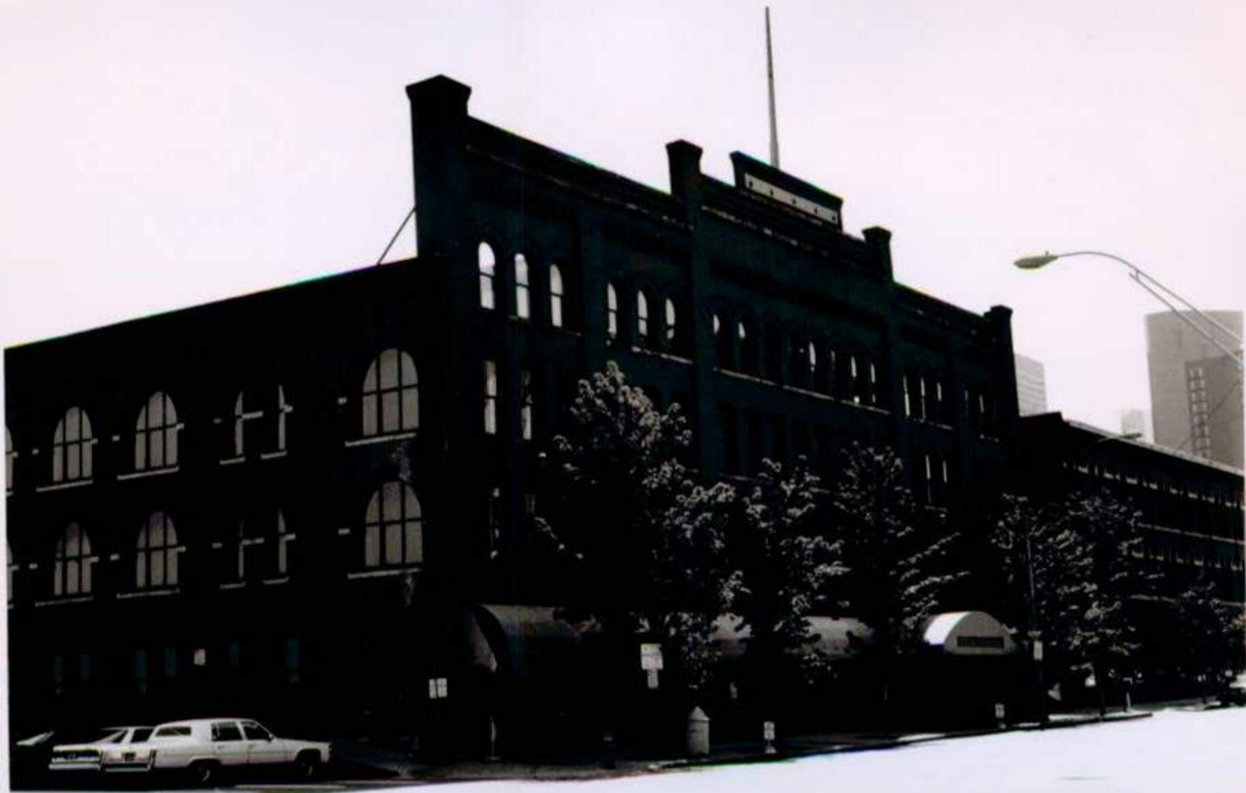
Lower Downtown Historic District #6 Denver, Colorado
