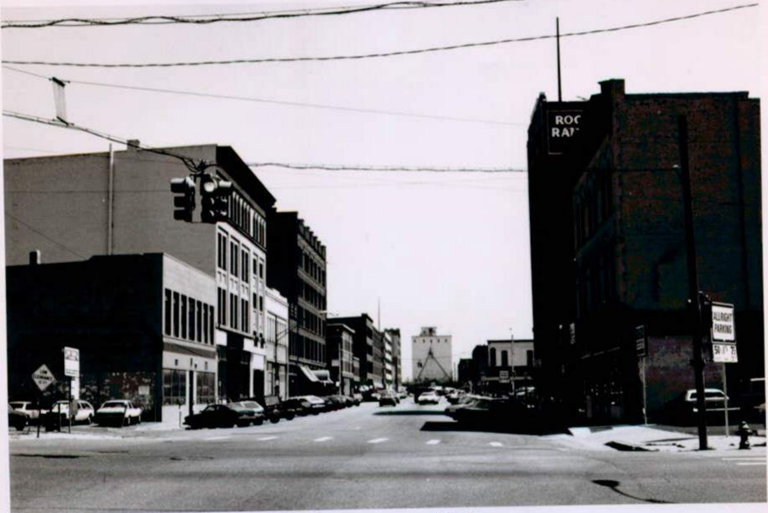
Lower Downtown Historic District #13 Denver, Colorado
