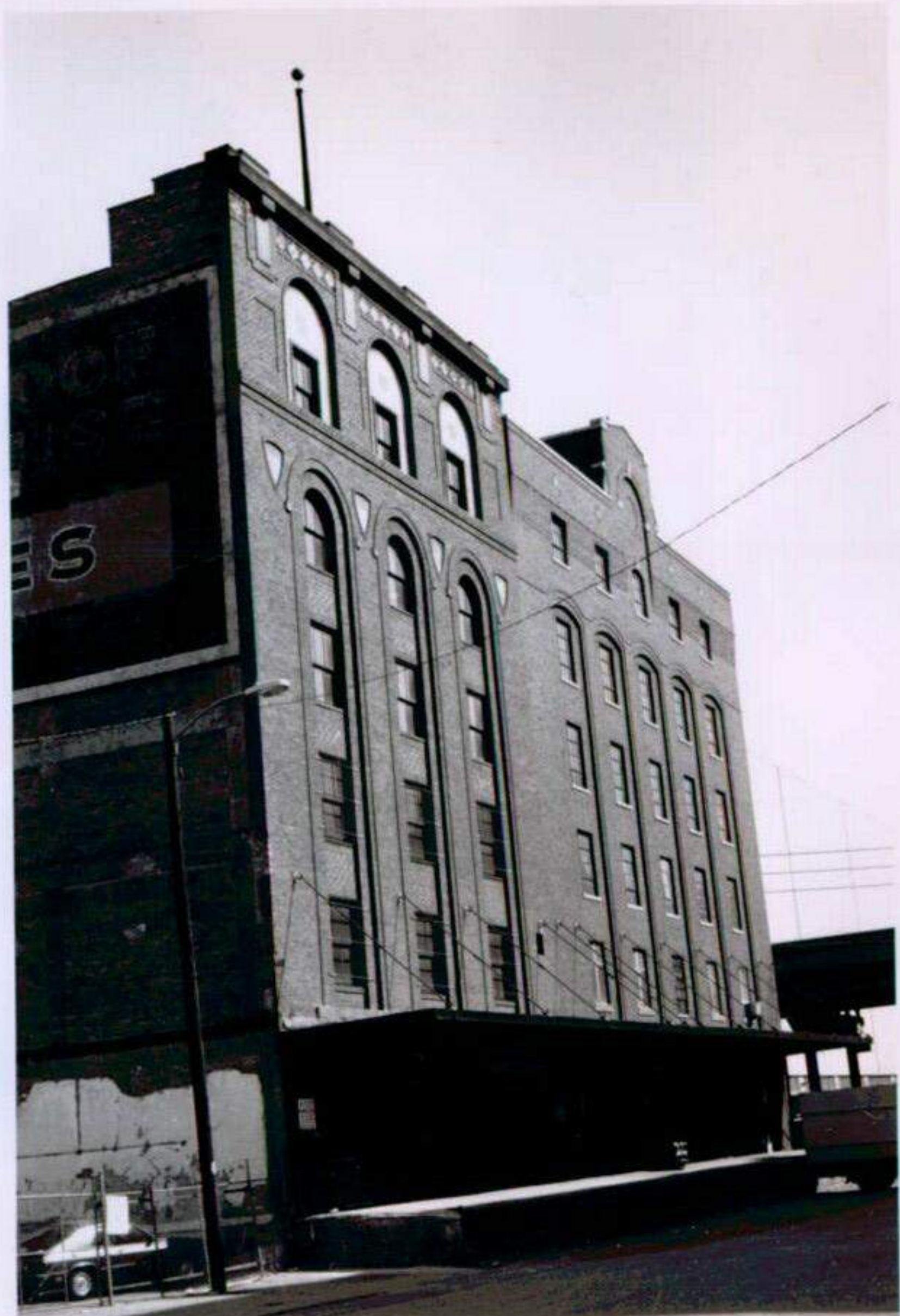
Lower Downtown Historic District #1 Denver, Colorado
