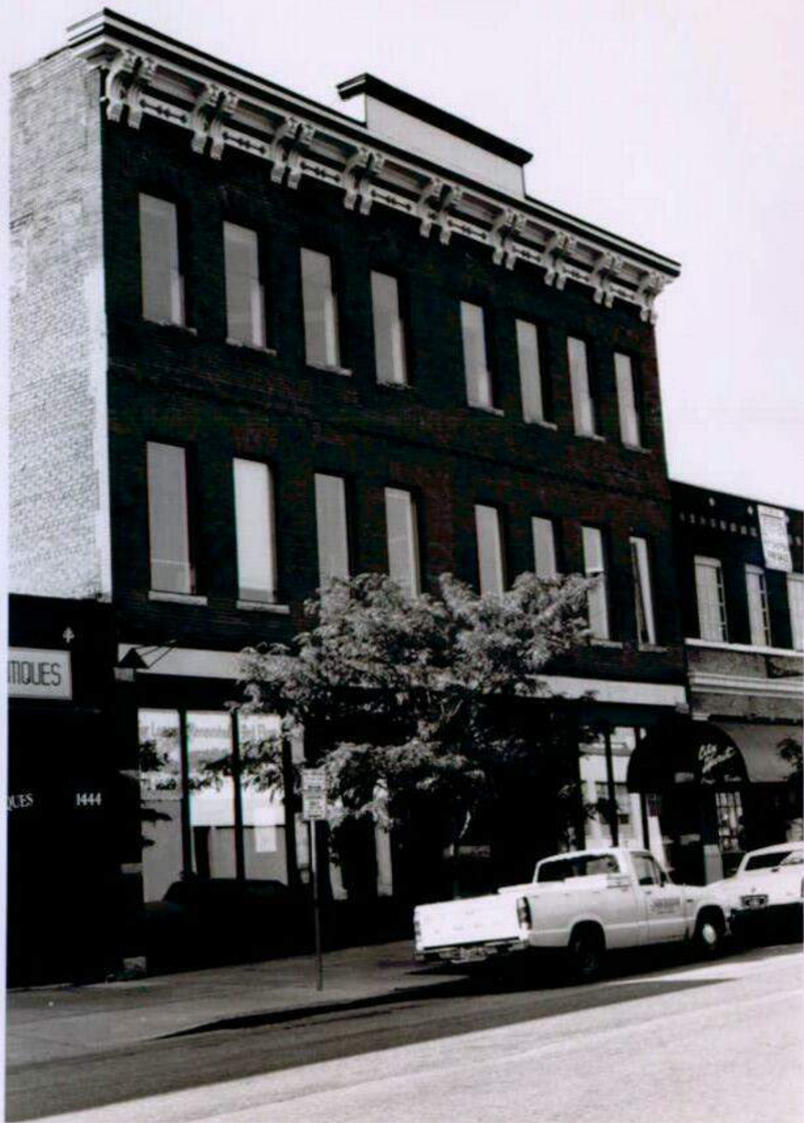
Lower Downtown Historic District #21 Denver, Colorado
