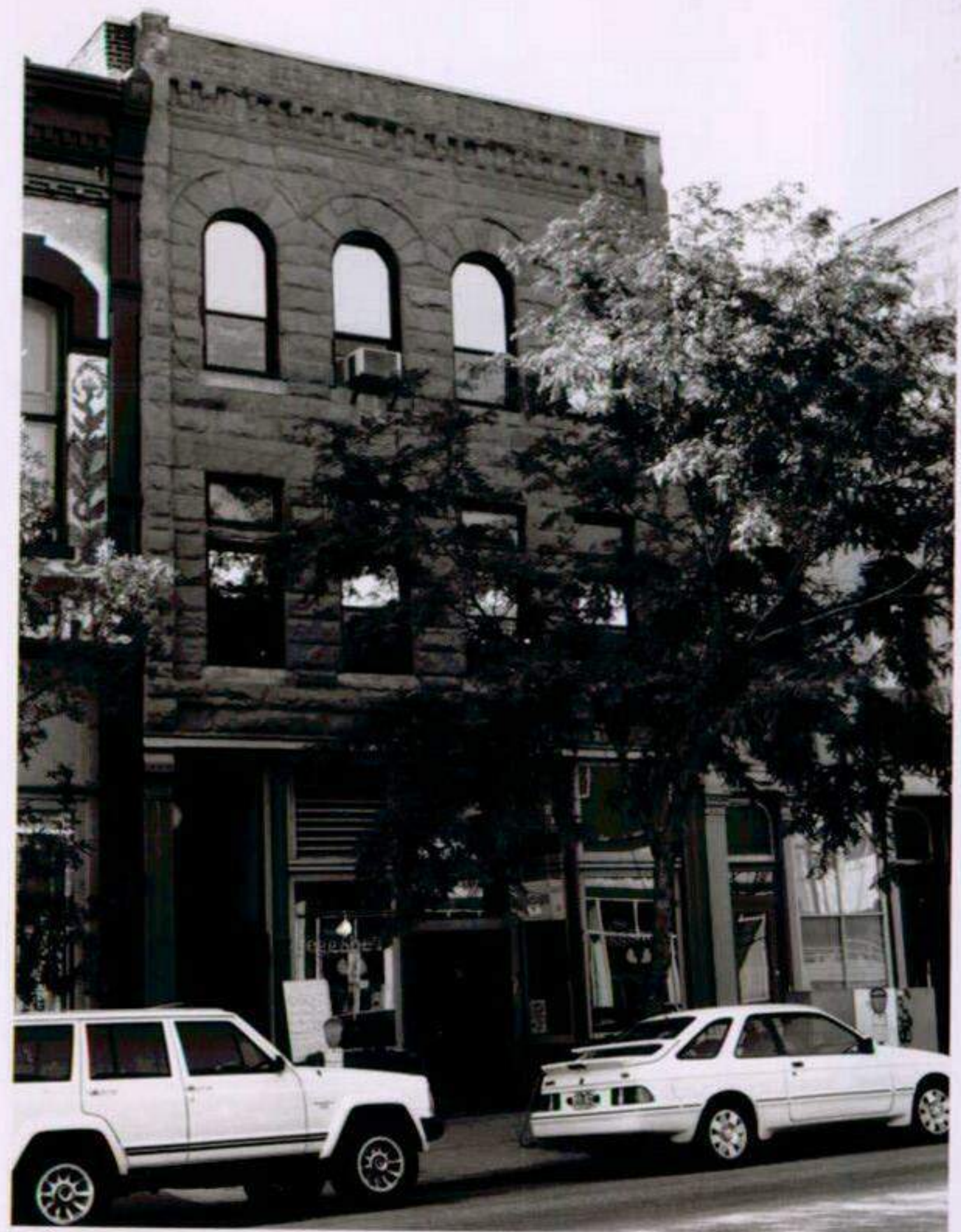
Lower Downtown Historic District #23 Denver, Colorado
