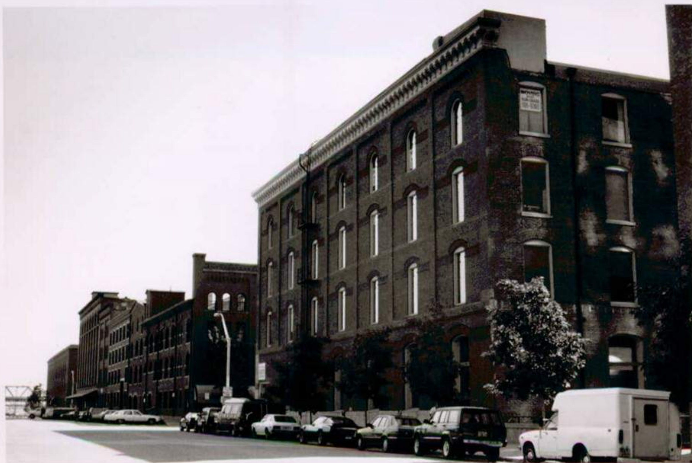
Lower Downtown Historic District #2 Denver, Colorado
