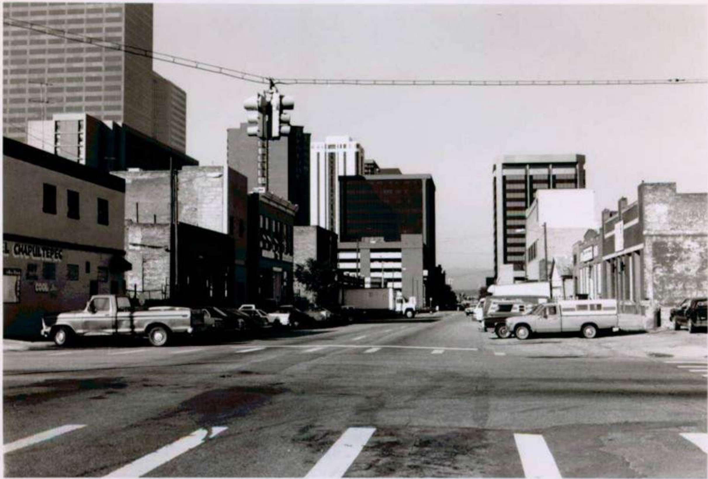
Lower Downtown Historic District #40 Denver, Colorado
