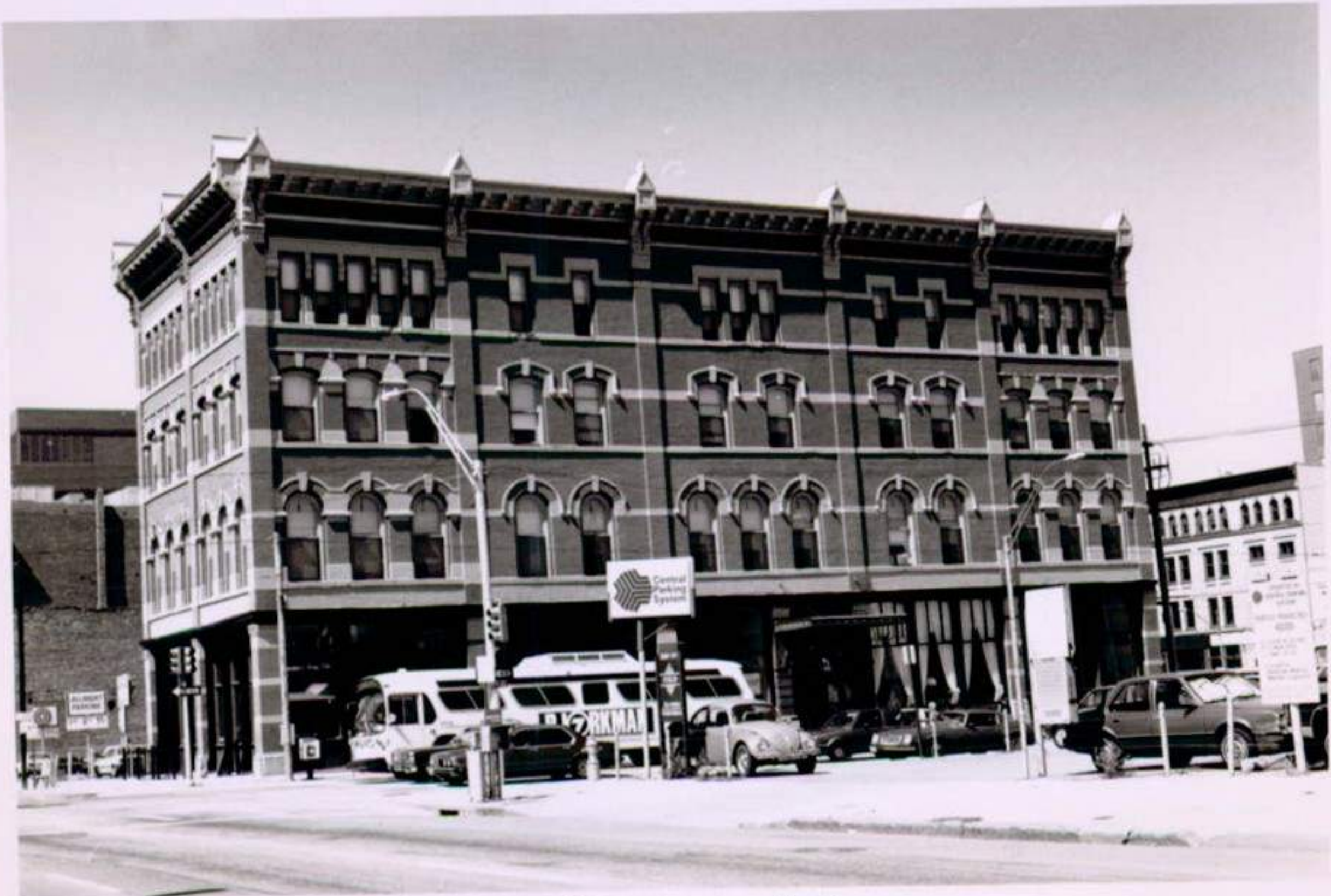
Lower Downtown Historic District #26 Denver, Colorado
