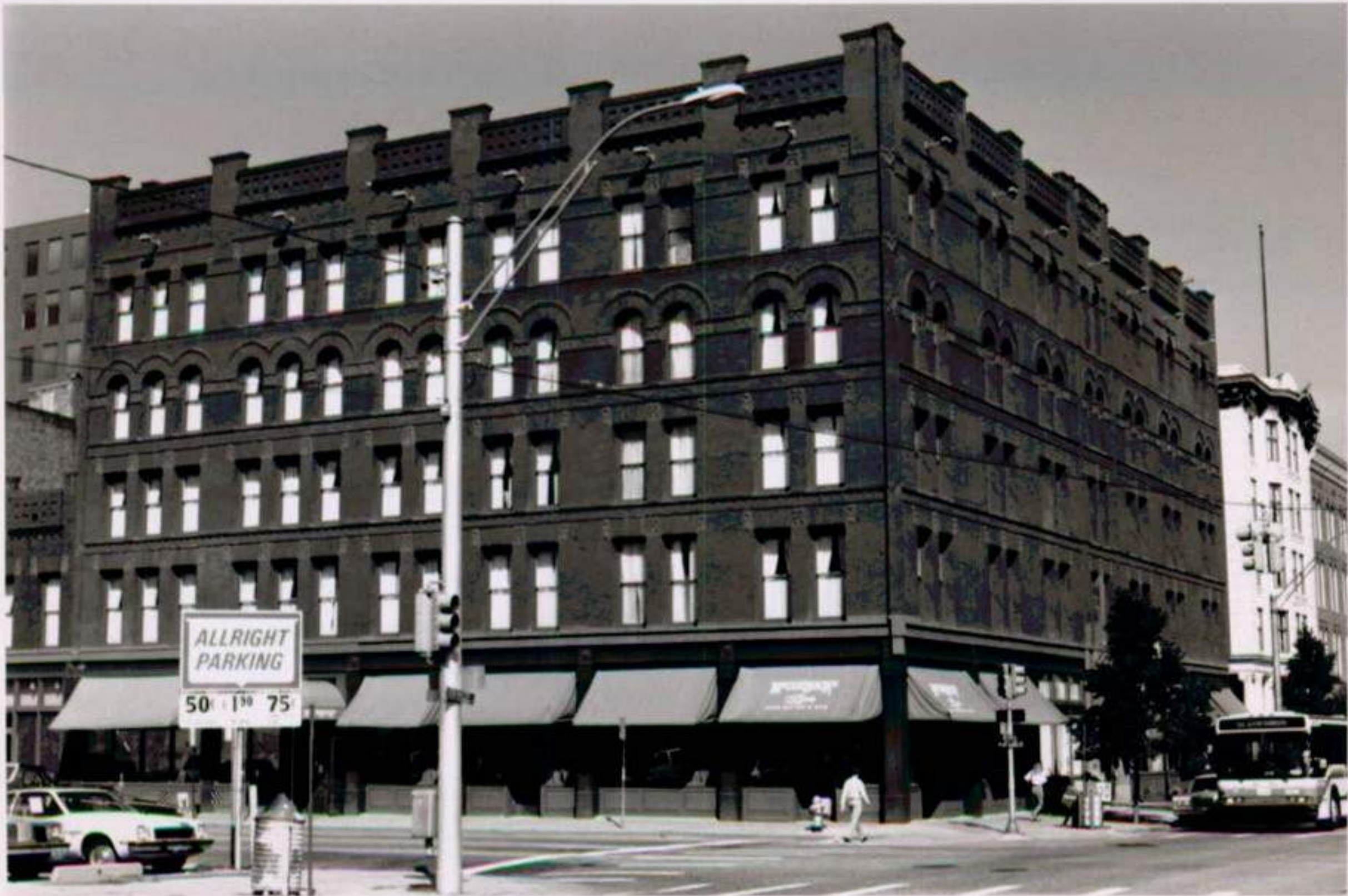
Lower Downtown Historic District #16 Denver, Colorado
