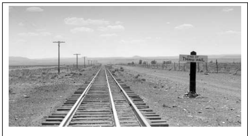
Figure 9. The end of the three-rail track comes just west of Antonito, marking the end of standard gauge operation on the San Juan Extension. Photographer: Otto Perry, June 21, 1943. Source: Western History / Genealogy Department, Denver Public Library.
