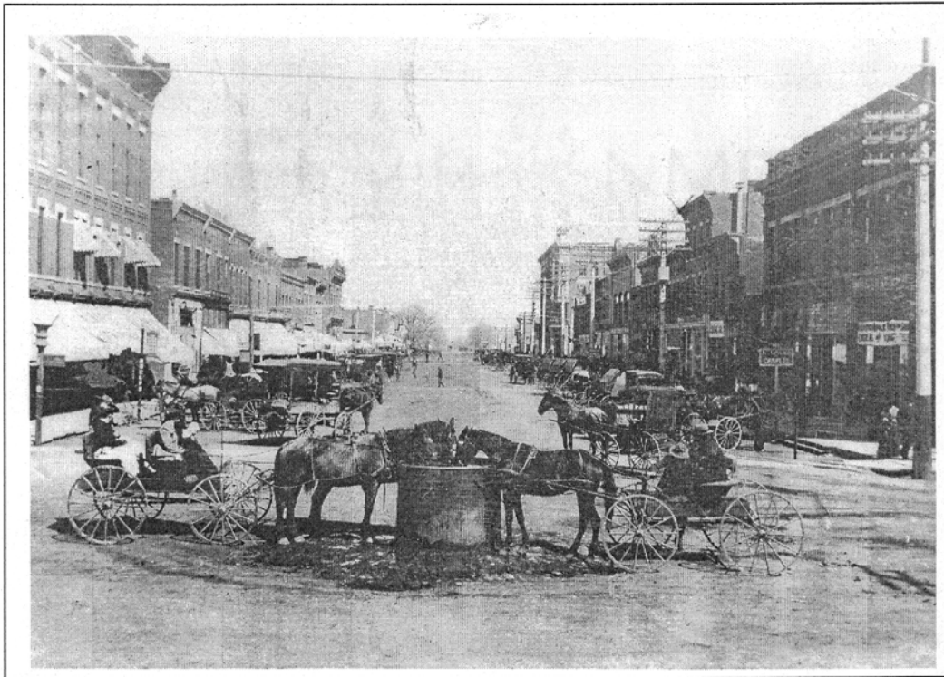
Photo H3: COGM 1976_143_0007 Intersection of 8 th St & 9 th Ave-Horses at Water Tank.jpg View of 8 th Street looking east from 9 th Avenue. Photo Courtesy of City of Greeley Museums Permanent Collection, #1976.143.0007.
