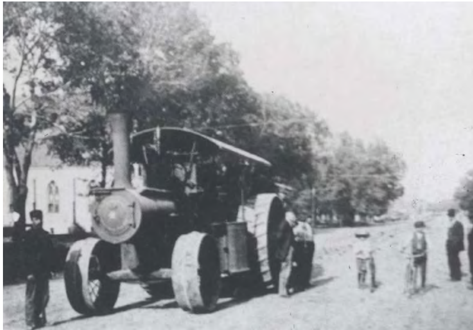
Figure 134. Grading the roadway for construction of the D&I streetcar lines, 1907. 626
