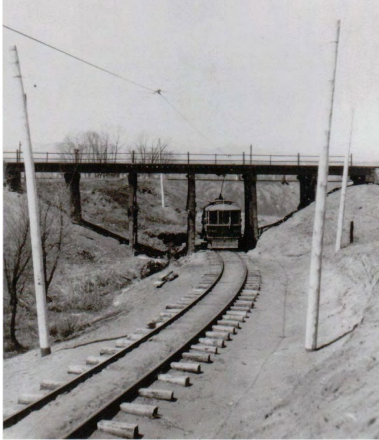
Figure 164. D&SP streetcar in Slaughterhouse Gulch, c.1910. Note the poles carrying the electric lines installed at an angle outward to keep the electric lines taught. 710 (Image from the Collection of the Littleton Museum. May not be reproduced in any form without permission of the Littleton Museum.)
