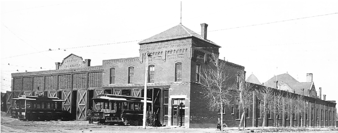
Figure 75. East Division car barn at East 35 th Avenue and Gilpin Street, built by the Metropolitan Railway in 1892. 380
