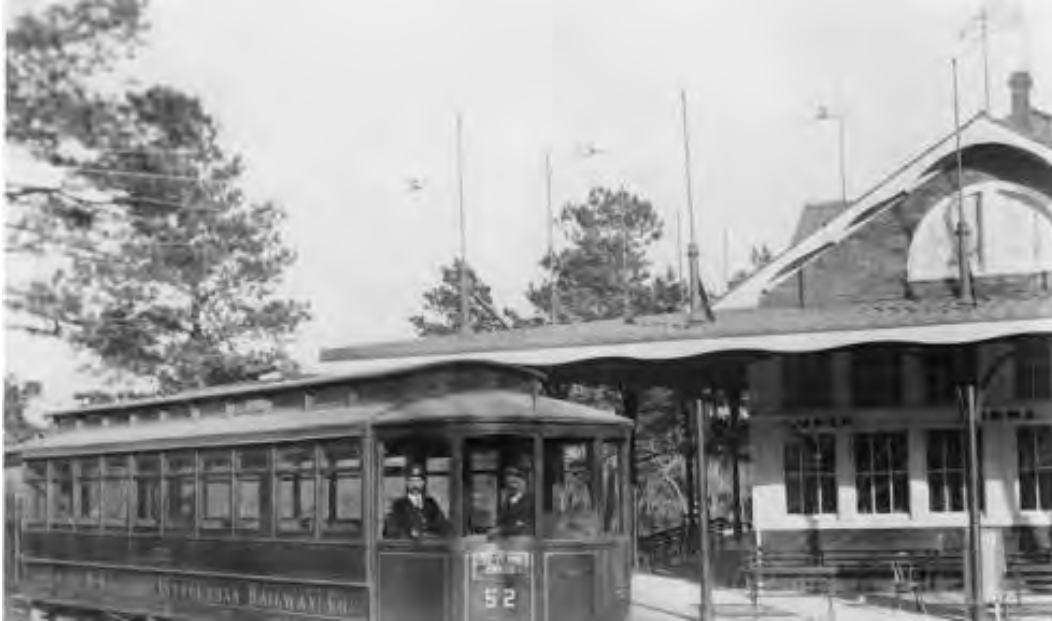
Figure 36. Streetcar and car pavilion at Stratton Park, c.1901-1910. 225
