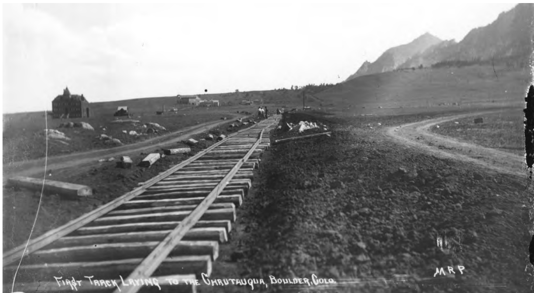
Figure 22. Laying track on the BR&U route to Chautauqua Park in 1899. 187
