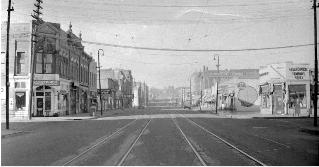
Figure 172. Streetcar tracks on Union Avenue looking north from D Street, 1938. 743
