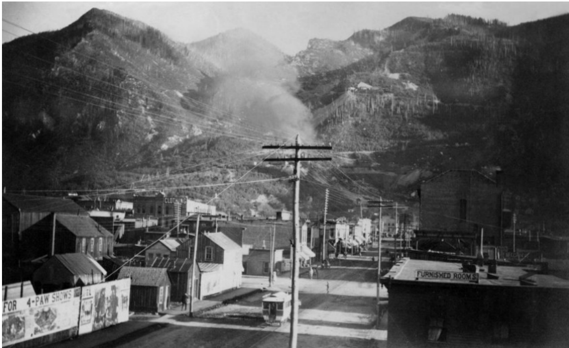
Figure 19. View of an ACR horsecar on Main Street, looking west from Mill Street, 1892. 176
