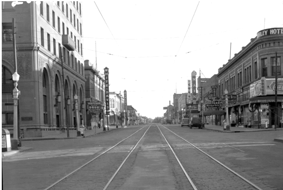
Figure 171. Streetcar tracks on Main Street looking north from 5 th Street, 1938. 742
