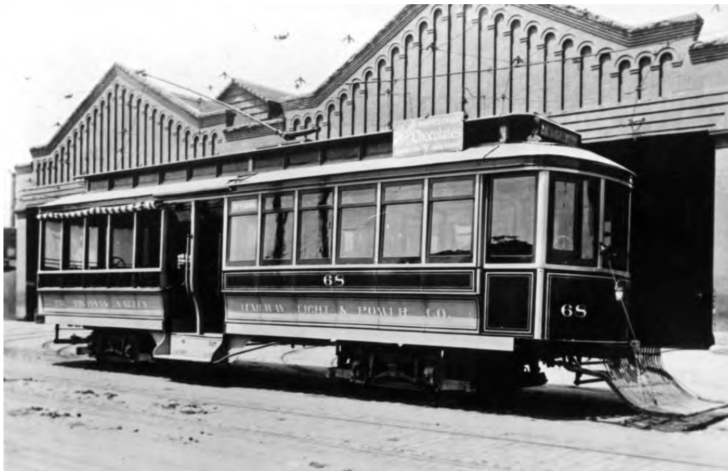
Figure 168. Streetcar parked in front of the 1890 car barn constructed by the PCR, c.1920
