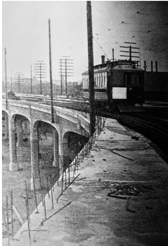
Figure 66. The Colfax-Larimer Viaduct under construction. 341
