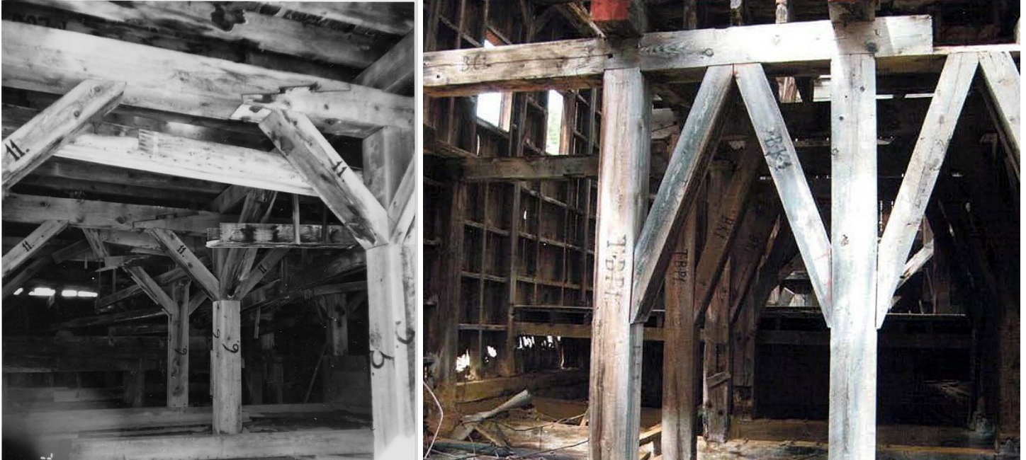
Figure 7: Frisco Mill interior, structural timbers with historic markings. Left photo taken 1997; right photo taken 2011. (Source: 1997 survey form completed by Susan Medville and 2011 survey form completed by James Herron, on file with History Colorado)
