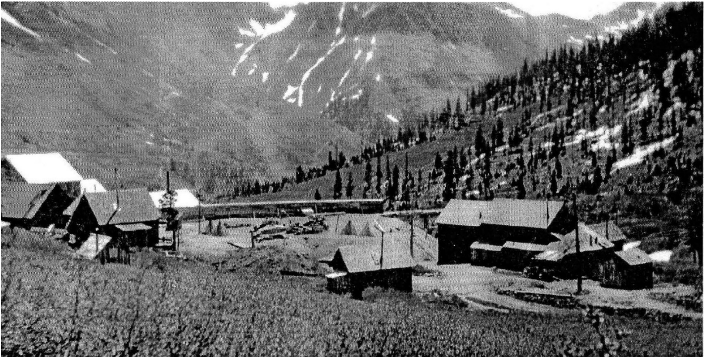
Figure 2: Bagley Tunnel Surface Plant ca. 1922. (Source: Gregg and Jean Harlow)
