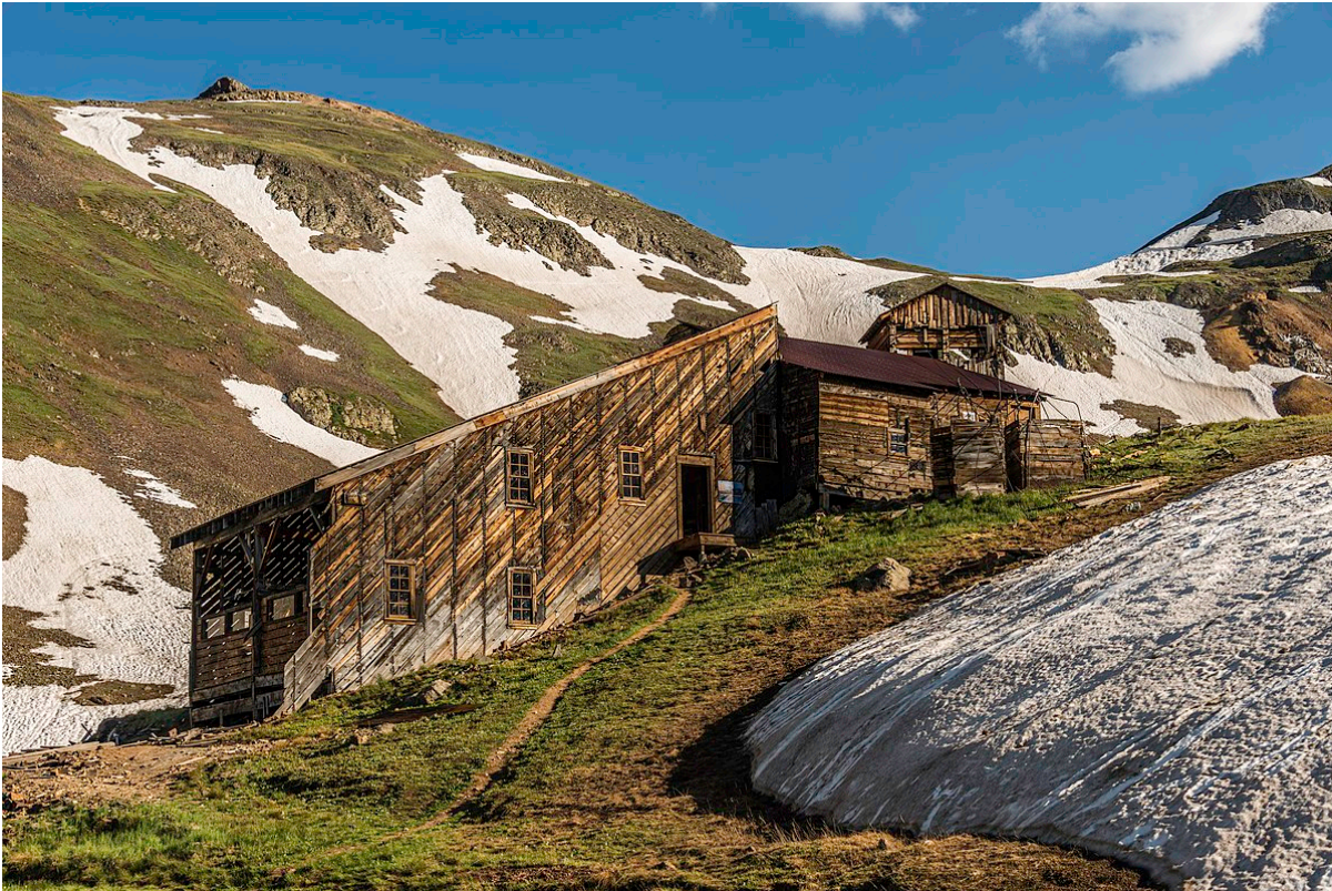
Figure 6: The Sound Democrat Mill in northern San Juan County exemplifies the traditional shed-roof mill design typically employed in the 1900s. (Wikimedia Commons)
