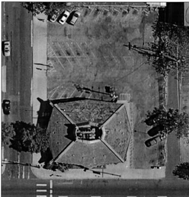
Figure H3. This view from the air vividly shows the unusual roof configuration of the White Spot at East Colfax Avenue and Pearl Street. SOURCE: GoogleEarth, 2007.
