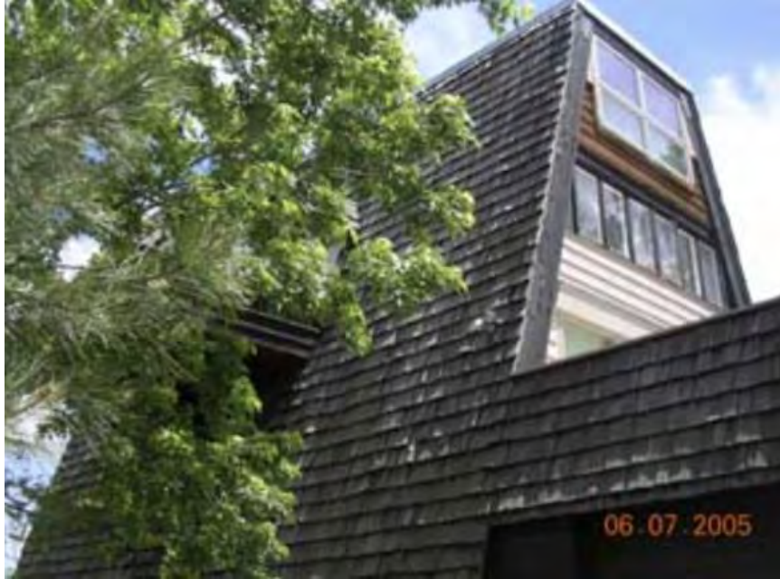
Figure 101. Example of a flat-top or clipped A-frame at 1900 Kohler Drive, Boulder. 201
