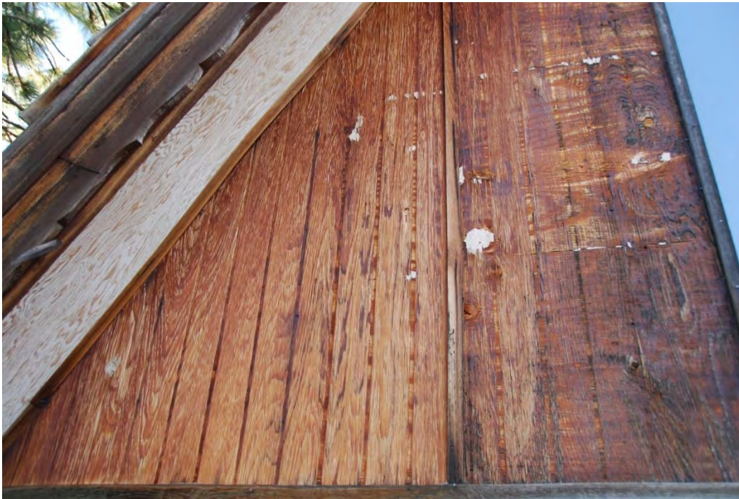
Figure 43. Exterior detail of the Beal A-frame showing the unpainted siding panels that give the effect of board and batten siding.
