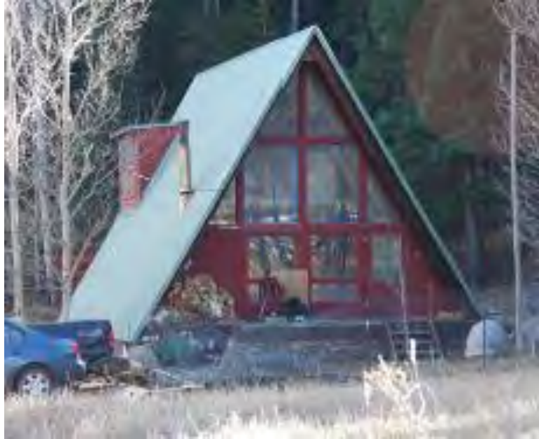
Figure 5. This Boulder County A-frame (71 Beaver Creek) represents the characteristics of the mountain type of A-frame vacation home.
