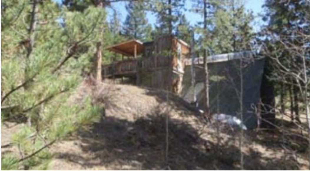
Figure 20. 71 Stinky Gulch Road, Nederland, showing how the A-frame home nestles into the topography. This A-frame is not yet attributed to an architect or kit supplier. 113
