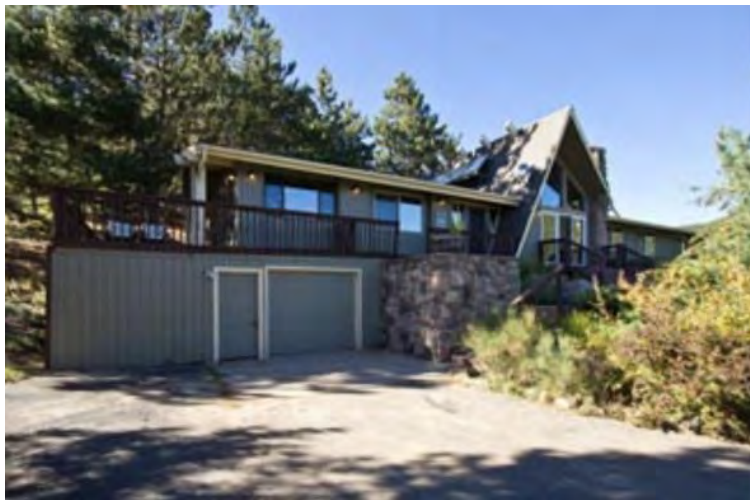
Figure 74. 324 Granite Drive, Unincorporated. This example features a steeply pitched roofline in the center of the building, above the entryway. Because the A-frame structure is only executed all the way to the ground on one side, this is not considered an A-frame. 191
