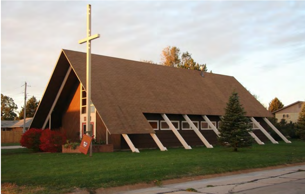
Figure 12. c.1970 A-frame church in Cozad, Nebraska. Note the use of side walls to maximize usable interior space.
