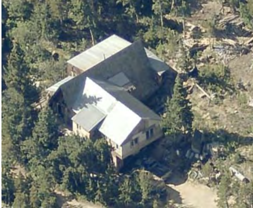
Figure 69. 0 B&M Street, Ward. This property is not considered an A-frame. While the original A-frame form is visible within the roofline of the building, multiple large additions have nearly encapsulated the A-frame form. 186
