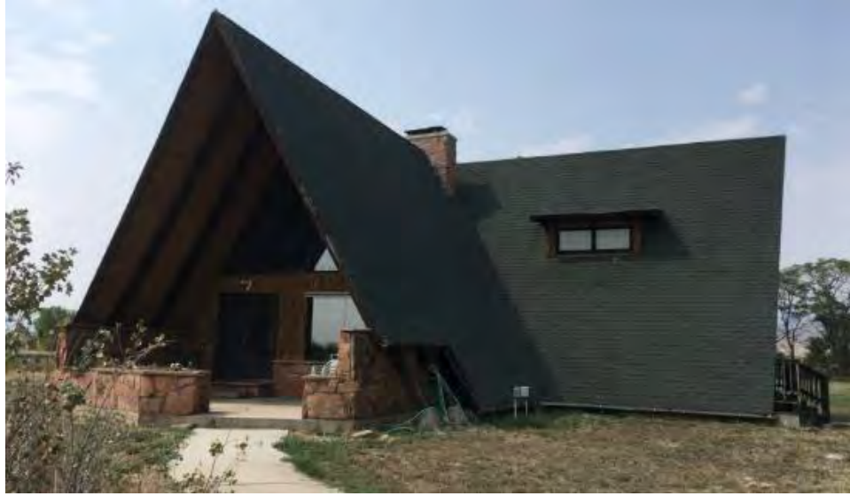
Figure 102. Example of a double A-frame at 12191 61 st Street, Unincorporated. 202
