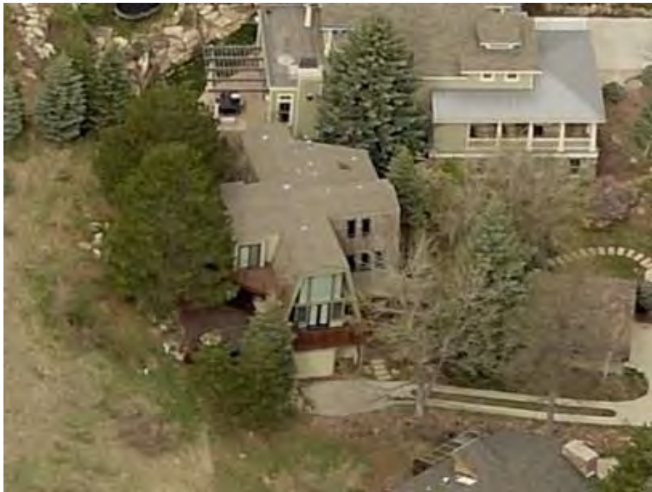
Figures 54 through 56. Examples of larger, architect designed A-frames within the West Highland Park Subdivision in Boulder. Clockwise from top left: 1900 Kohler Drive, 1920 Kohler Drive, 1960 Kohler Drive. 171
