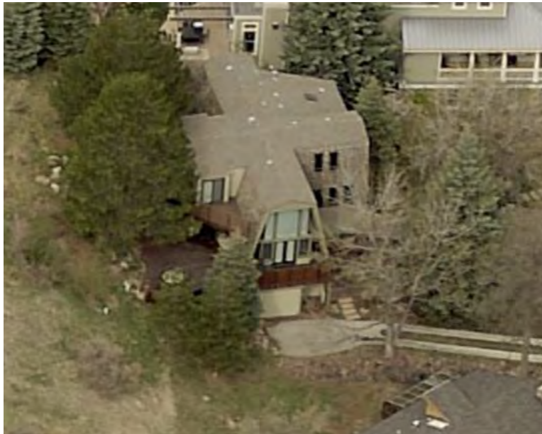
Figure 100. Example of gambrel roof A-frame at 1960 Kohler Drive, Boulder. The large, non-A-frame additions to the rear of the property compromise the integrity of the gambrel roof A-frame portion. 200
