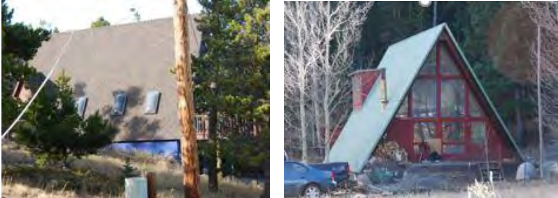
Figures 80 and 81. Examples of skylights and dormer windows. Left: 490 Camp Eden Road, Unincorporated. Right: 71 Beaver Creek Drive, Unincorporated.
