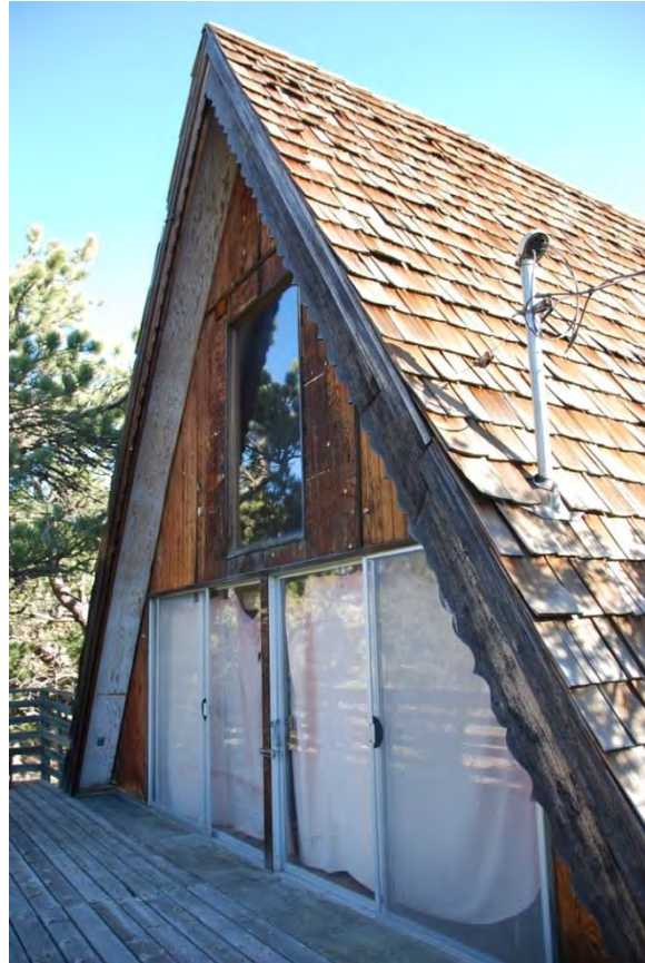
Figure 41. Front elevation of the Beal A-frame.
