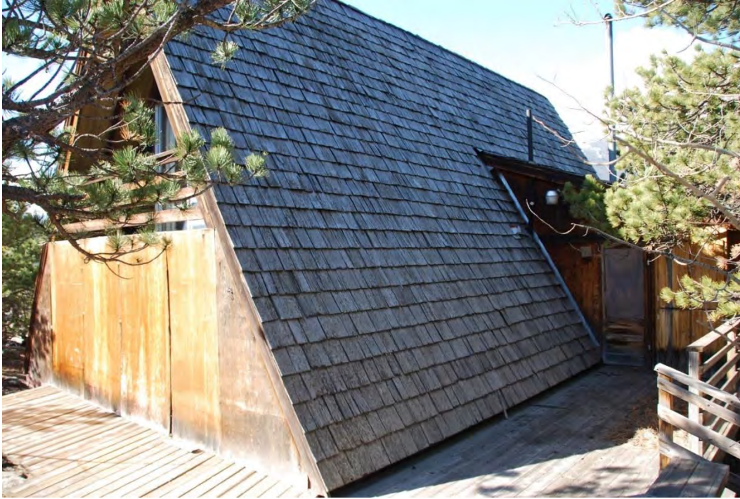
Figure 44. The Beal A-frame showing the cedar shingles utilized on roof. Note the addition to the side.
