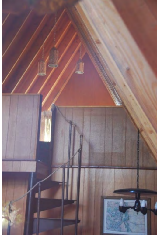
Figure 45. Interior of the Beal A-frame showing the metal spiral staircase, exposed interior rafters, and plywood paneling.
