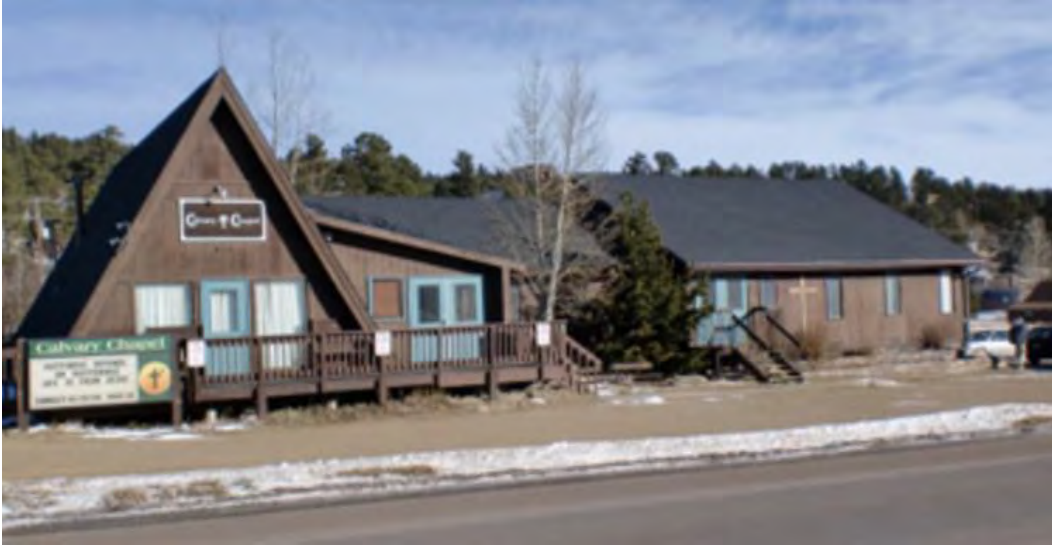
Figure 16. The Calvary Chapel Nederland appears to be a Delta A-frame on the left portion on the building, with multiple additions to the right. 103
