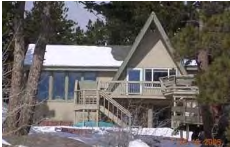
Figure 72. 101 Hickock Trail, Unincorporated. This building is considered a modified A-frame. It has wings on the side; however, these wings do not dominate the building and the A-frame form is still the focus of the building. 189
