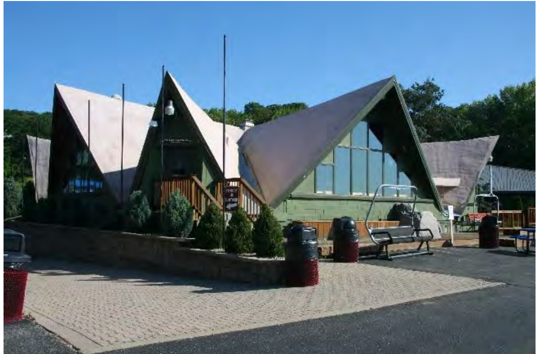
Figure 8. 1962 lodge at Cascade Mountain Ski Resort in Portage, Wisconsin. Note the multiple gables.
