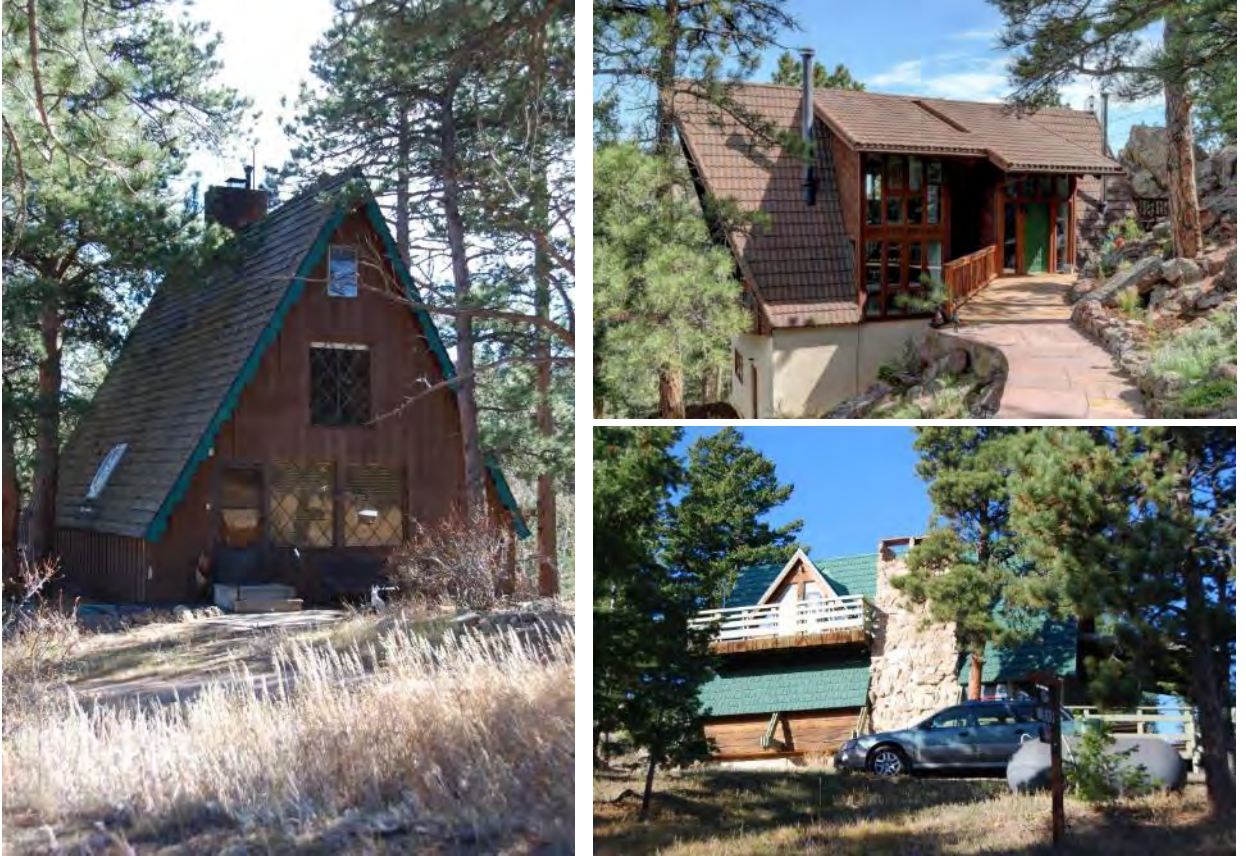
Figures 82 through 84. The addition of stylistic elements is a common variation to the standard A-frame. Left: Scalloped barge board and diamond pattern glazing details on 393 Ski Road East, Unincorporated. Upper right: Asian-inspired details on 213 High View Drive, Unincorporated (note the carved front door). Lower right: Rustic details on 98 Mine Lane, Unincorporated. 194
