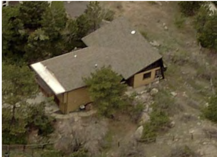
Figure 73. 177 Deer Valley Road, Boulder. Note the steeply pitched roof on the right side of the building, creating a “half A-frame” effect. This is not considered an A-frame as it does not employ the symmetrical, triangular A-frame truss structure. 190
