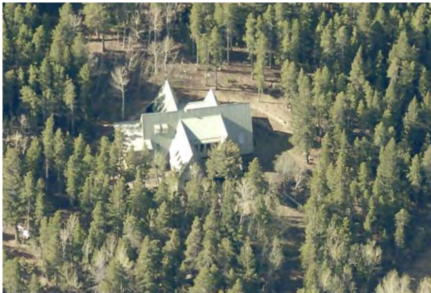
Figure 70. 78 Evergreen Way, Unincorporated. This property is not considered an A-frame. The A-frame form is visible in the center of the building, but multiple intersecting additions have been added on both sides, perpendicular to the A-frame. 187
