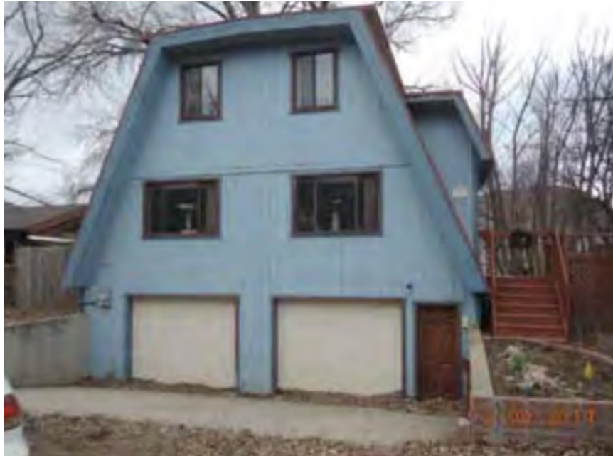
Figure 68. 115 Park Street, Lyons. This building is an example of a flat-top or clipped A-frame. 185
