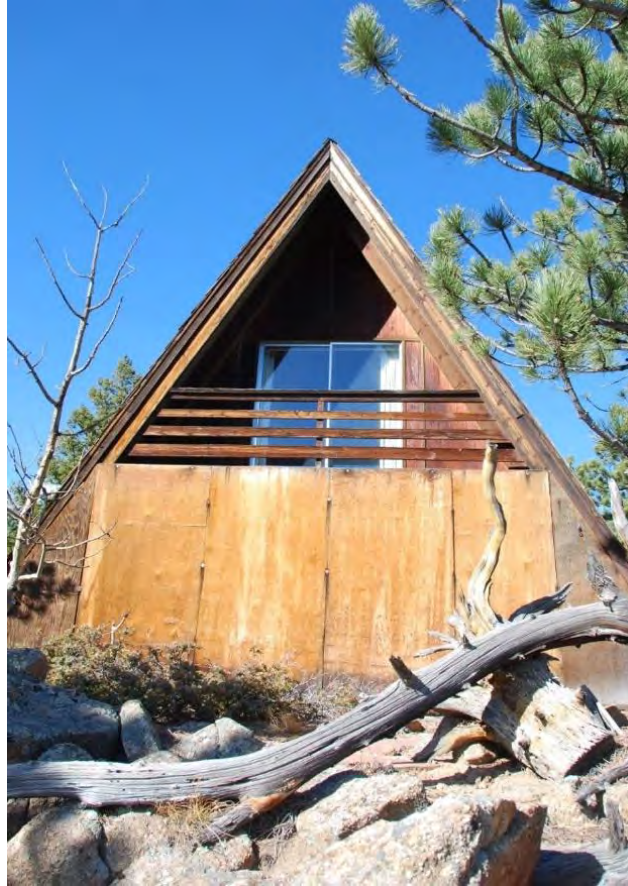
Figure 46. Rear of the Beal A-frame showing bracing on the rear gable. The plywood and horizontal header beams above were later modifications to strengthen the building from the wind gusts experienced at the top of the rock promontory.
