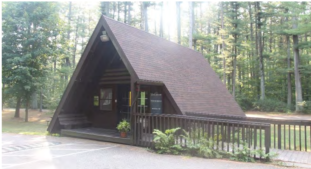
Figure 6. c.1960 Rocky Arbor State Park office near Wisconsin Dells, Wisconsin.
