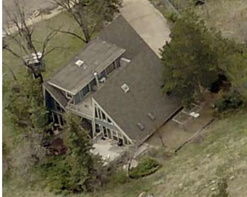
Figure 71. 1845 Kohler Drive, Boulder. This represents a high-style, architect-designed example of experimentation with the A-frame form. While multiple additions and alterations were made to the residence over the years, the A-frame form is still visible on the far left of the building. The basic A-frame form is still retained as the main massing of the building, with a smaller, mirror A-frame located parallel to the main A-frame. This building is considered a high-style example of an A-frame. 188
