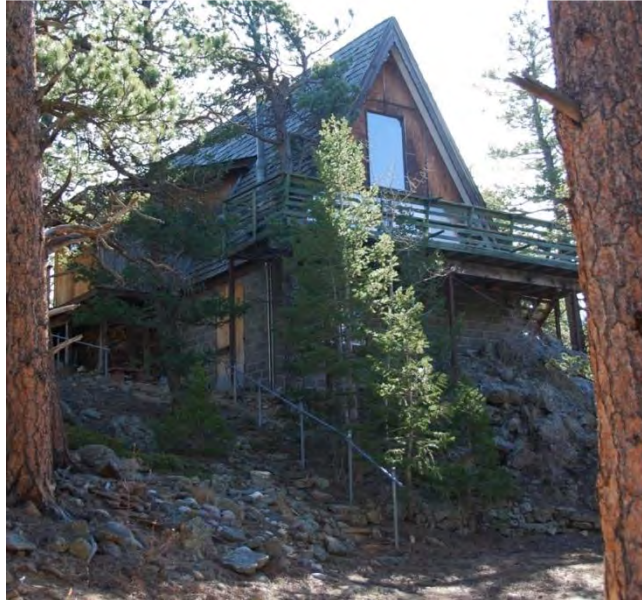
Figure 39. Exterior of the Beal A-frame at 128 Cabin Creek Road, Unincorporated, a Delta Vacation Home. This is likely a Chateau model based on the four sliding glass doors on the first floor, spiral staircase, and number of bedrooms. Note the unique setting of the house built atop a rock outcrop, and the angled deck railing.
