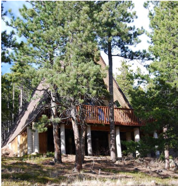
Figure 58. 520 Rudi Lane, Unincorporated. Note the piers supporting the deck and roofline.
