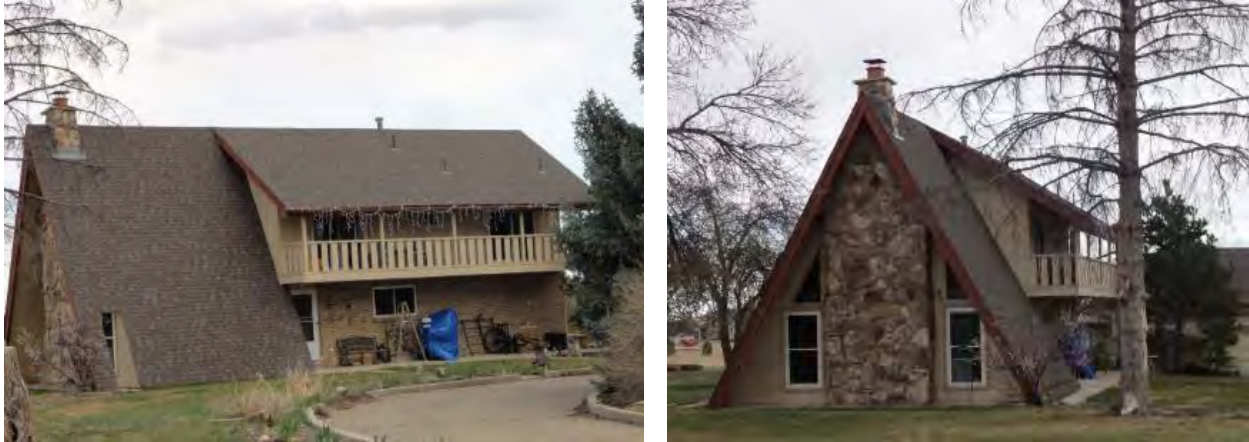
Figures 89 and 90. Additional exterior variations include notched roofs/walls to accommodate recessed window and door openings and the placement of large Ranch-style chimneys in the gable end such as at 12738 Sheramdi Street, Unincorporated. 196
