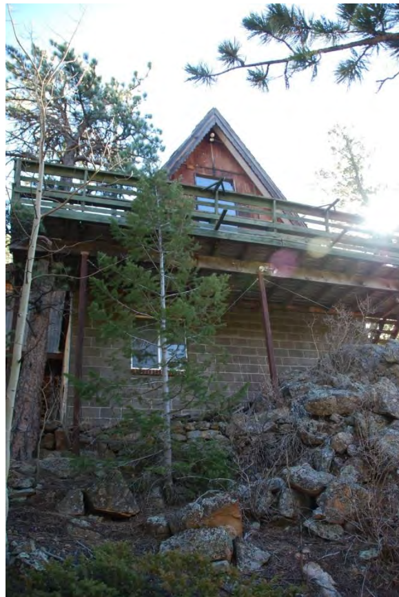
Figure 40. Siting of the Beal A-frame atop a steep rock promontory. Note the concrete block foundation constructed atop the rock promontory.
