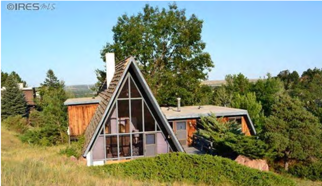
Figure 64. 1905 Kohler Drive, before demolition. 181
