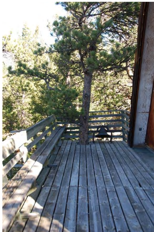
Figure 36. Deck on Delta Vacation Home A-frame with signature angled railing and integrated bench. 128 Cabin Creek Road, Unincorporated.
