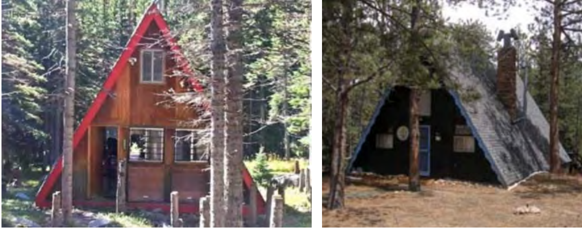
Figures 75 and 76. Examples of standard A-frames. Left: 3653 Fourth of July Road, Unincorporated. Right: 847 Hemlock Road, Unincorporated. 192
