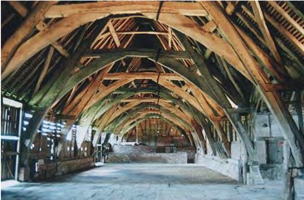
Figure 1. Cruck framing as seen in the Leigh Court Tithe Barn in Worcester, England. Note how the cruck beams are A-shaped timbers that extend short foundation walls. 5
