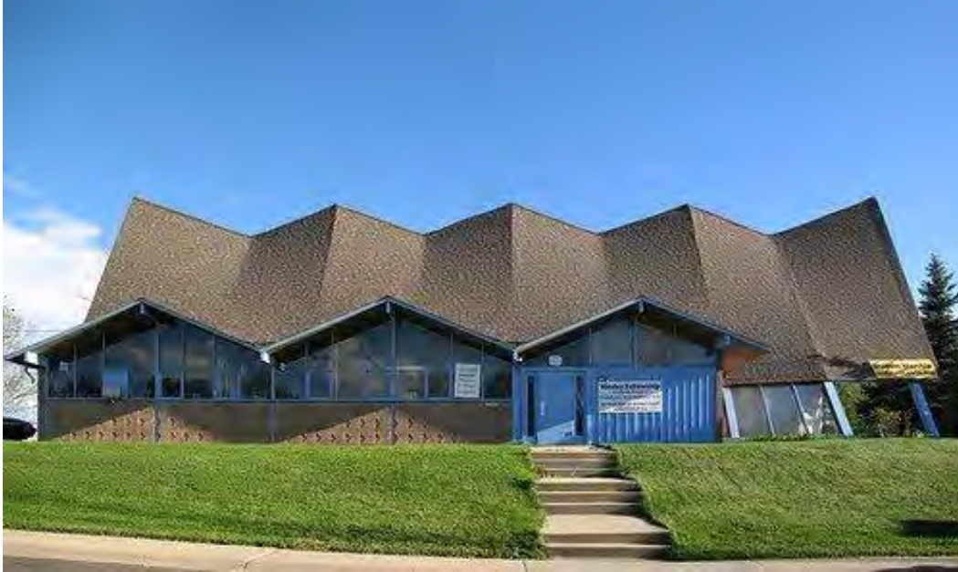
Figure 23. The north side of Methodist Student Center, 1290 Folsom Street. 120
