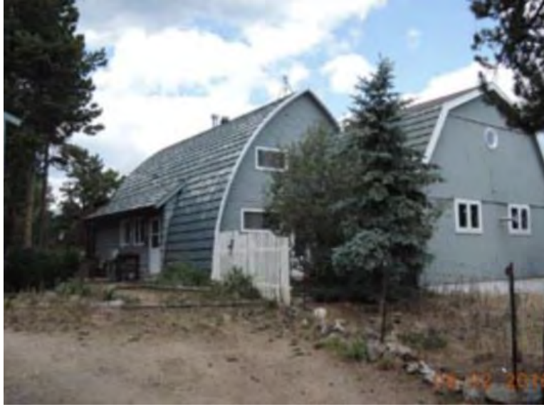
Figure 99. Example of Arched (Gothic) A-frame at 83 Alpine Drive, Nederland. 199
