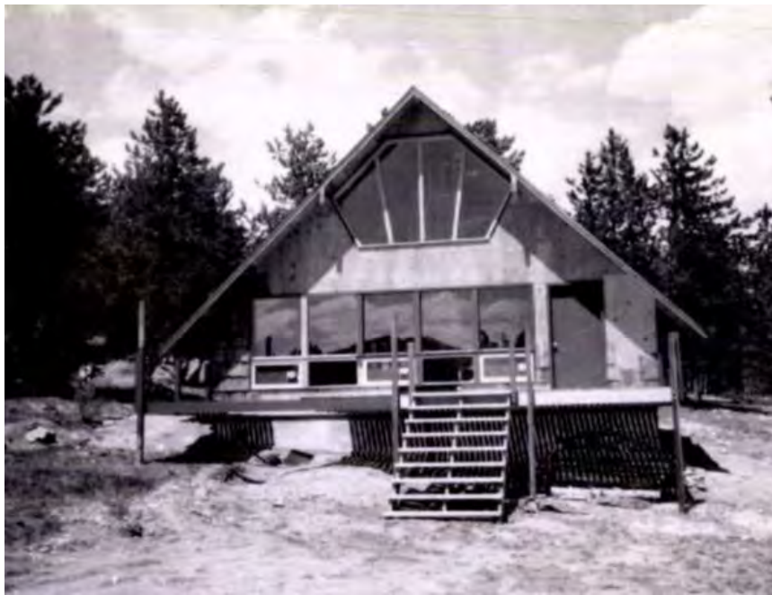
Figure 67. 118 Grizzly Drive, Unincorporated. This building is considered an A-frame. Although it has knee walls preventing the roofline from reaching the ground, the knee walls do not constitute more than two-thirds the height of the full main floor. In addition, early assessor's notes of the interior show an open first floor with a loft, typical of A-frame designs. 184
