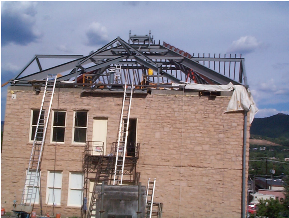
HP8. 8. The Animas City School/ Animas Museum in 2006 during the reconstruction of the hip-style roof. Camera looking east
