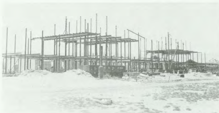
The artist's depiction of the Grand Junction factory became a reality as construction began in 1899. Thirty rail cars of structural steel supported the three-story high building. Note the beet storage sheds in the background (below).
