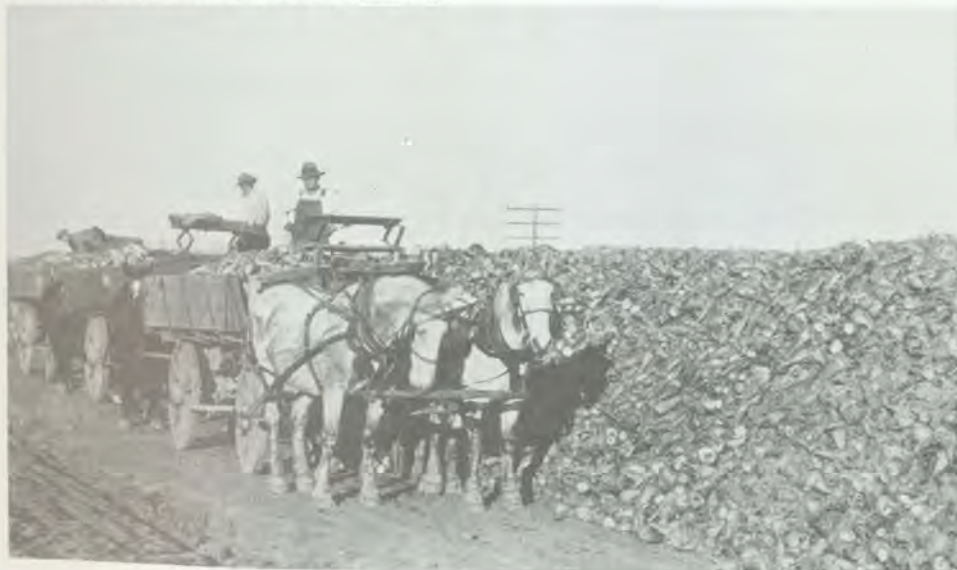
Unloading sugar beets at the railroad siding.
