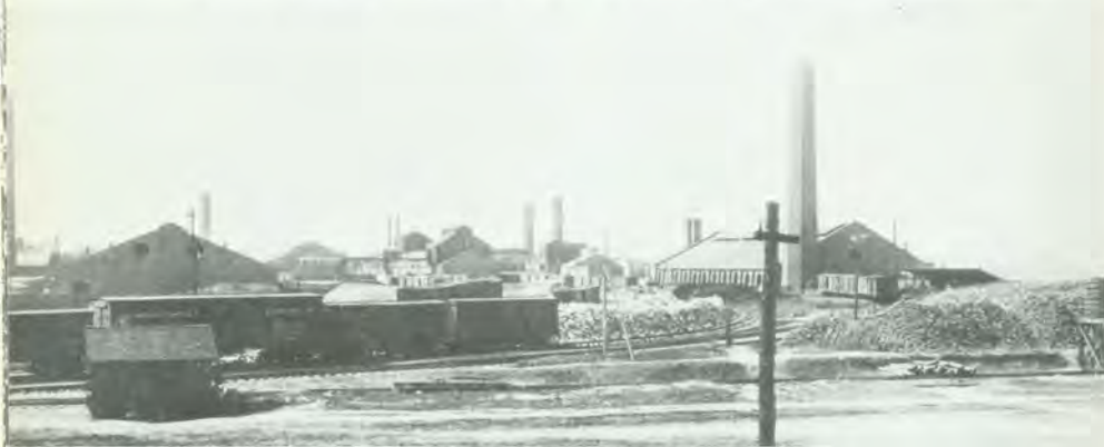
The Grant Smelter, built in 1883 on the South Platte River in north Denver.
