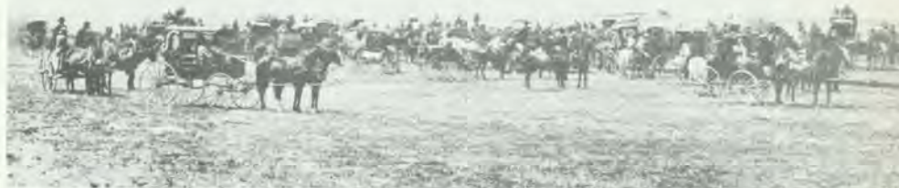
Breaking ground on the Denver Pacific, May 18, 1868, near what was the junction of the Denver Pacific and the Kansas Pacific railroads.
