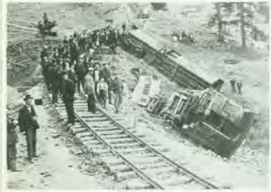
On Oil Creek, 6.4 miles north of Canon City via Field Ave. Bronze
