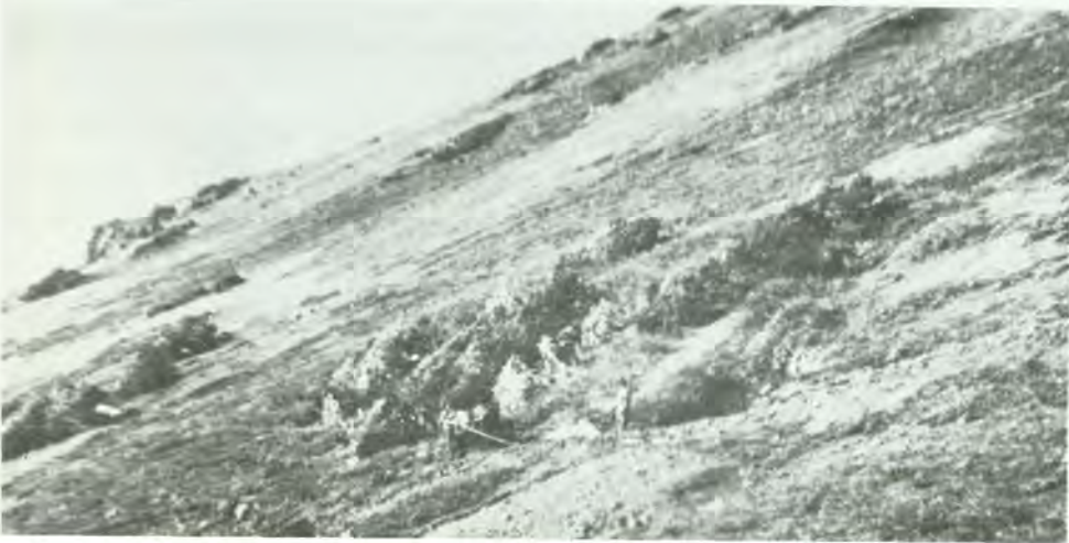
Grading on the east side of Tin Cup Pass.
