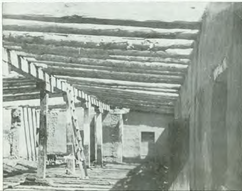
View of one of the Fort Garland structures taken during restoration.
