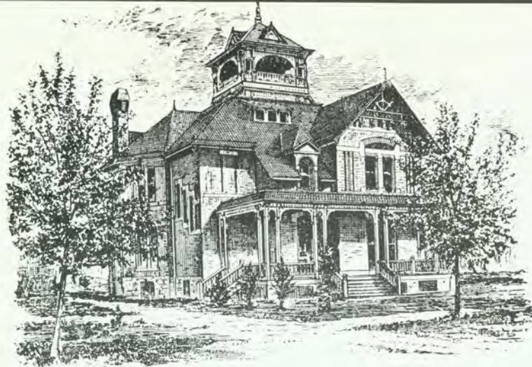
Eaton home at Madison Avenue and Linden Street (805 12th Street), Greeley.
