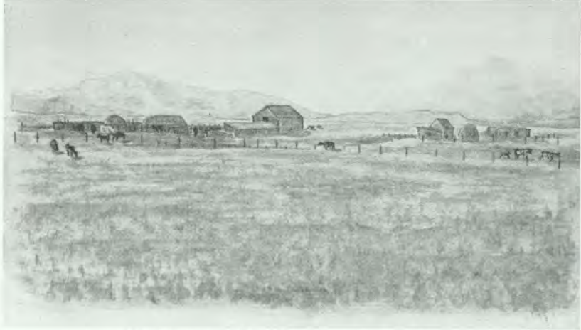
Buildings at the ZA Ranch; note barn in center and ranch house at far right.
