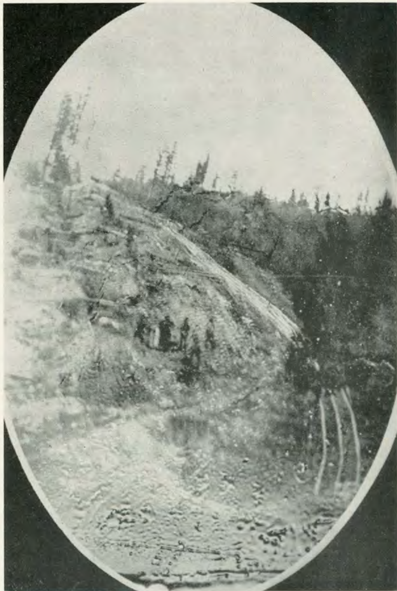
"LOG SLIDE IN WHICH WE BROUGHT THE ORE FROM THE GOLD MINE TWO HUNDRED FEET ABOVE DOWN TO THE WATER SLUICE. THE ORE BEING TIED IN BUFFALO SKINS." REMARKS ON BACK OF ORIGINAL PHOTOGRAPH.
