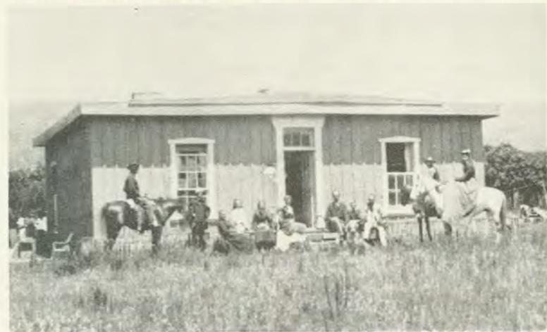
FIRST FRAME HOUSE BUILT IN COLFAX COUNTY, NEW MEXICO, 30 MILES FROM TRINIDAD
