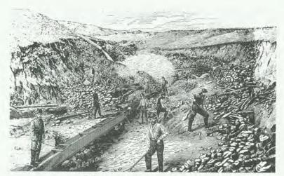
Prior to using heavy equipment for underground mining, prospectors separated ore from rocks and pebbles by running water over the gravel in a sluice.
