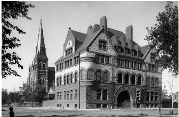
The Denver Club, at 17th Street and Glenarm Place in Denver, shows Richardsonian Romanesque design influences in its large arched doorway, arcade windows, contrasting rusticated stone trim, and dormers. In this ca. 1890 view, the First Congregational Church stands behind the club building on Glenarm Place. Source: William Henry Jackson Collection of the Colorado Historical Society.
