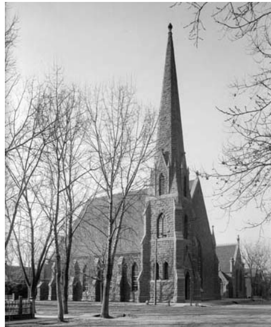
The Grace Methodist Episcopal Church at 13 th and Bannock in Denver was attributed to Varian and Sterner. Ca. 1890 photograph. Source: Colorado Historical Society.
