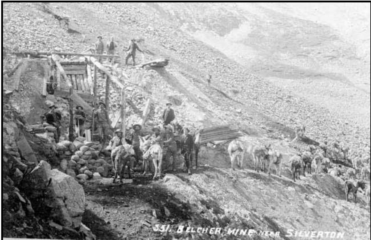
Figure F 2: By the early 1880s, the Belcher Mine recently joined the county's ore producers. In its primitive state, however, the mine resembled a deep prospect in many ways. The operation was small and simple, the underground workings were shallow, and the waste rock dump therefore small. In addition, the surface improvements were minimal, the structures few and crude, and access provided only by a packtrail. Although no buildings are evident, a blacksmith shop was probably nearby. Source: Denver Public Library, Western History Collection, C-77.
