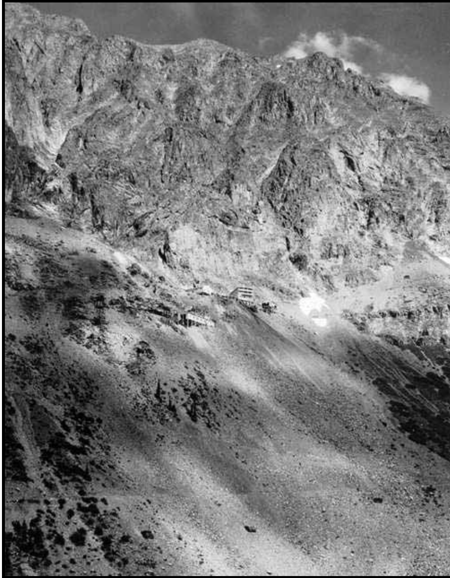
Figure E 38: The Mayflower Mine, at the base of the cliff at center, was the leading mine in San Juan County from the late 1920s until closure in 1954. The surface facilities included a five-story boardinghouse, the upper terminal for a tramway, and shops. The tramway carried ore down to the Mayflower Mill on the Animas River. The operation was the county's economic cornerstone and largest employer. Source: Denver Public Library, Western History Collection, X 62245.
