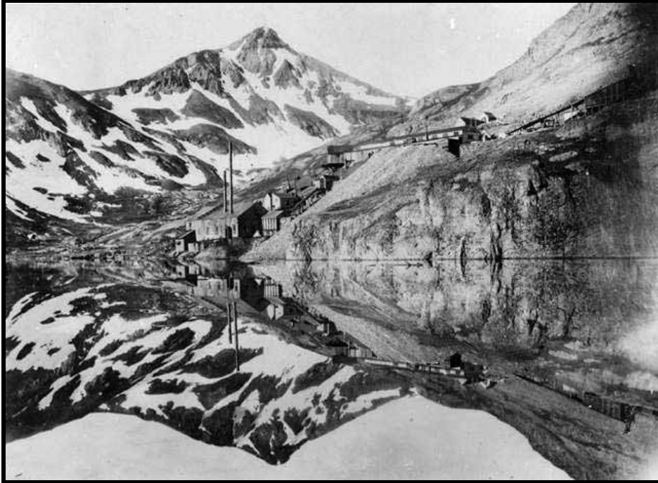
Figure E 27: The south view depicts the Iowa Mine in 1898 during a rare calm day in Silver Lake Basin. At this time, the Iowa ranked among the county's most important mines. The buildings at left were a compressor house and tram terminal, and the long structure at the upper right enclosed shops and the portal of the Iowa Tunnel. Source: Denver Public Library, Western History Collection, X 62274.
