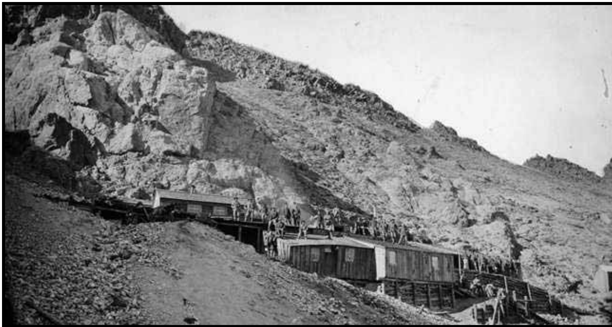
Figure E 17: Although this north view of the North Star Mine's tunnel house was taken around 1900, the building changed little from when engineer Eben Olcott erected it in 1881. The building housed the mine's tunnel portal, blacksmith shop, ore sorting station, and living quarters under one cramped and drafty roof. Source: Denver Public Library, Western History Collection, X 62714.
