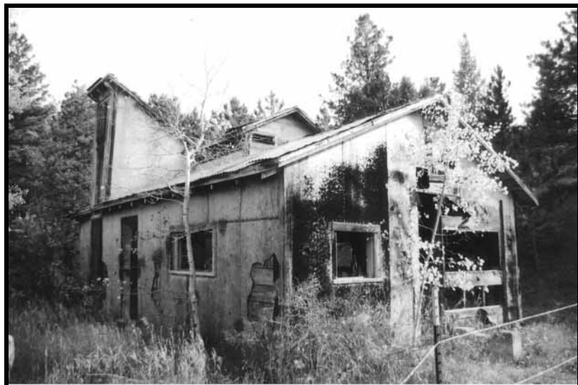
Figure E 76: Shaft houses enclosed the shaft collar, headframe, hoist, power system, and usually the blacksmith shop. The shaft house in the profile also features a Cornish pump and steam engine, rarely used in San Juan County. Source: International Textbook Company, 1899, A43:3.
