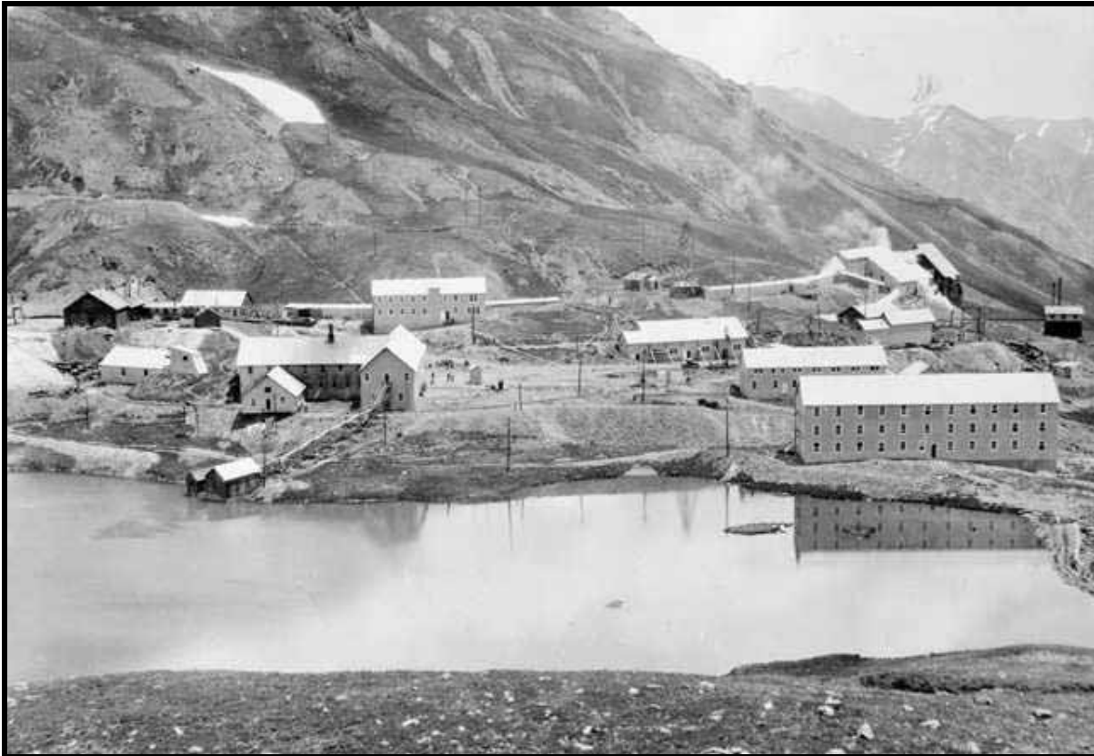
Figure F 4: The Sunnyside Mine, pictured in 1917, exemplifies the scale that some large mines attained in San Juan County. The mine, located above treeline on Lake Emma, had several tunnels, a complex surface plant, and massive boardinghouses for the crew. The surface plant included support facilities, machinery, a mill in the right background, and pump station on the lake. Although the plant evolved organically over time in response to need, it appears that the company engineer formally designed the buildings. Source: Denver Public Library, Western History Collection, X-62224.
