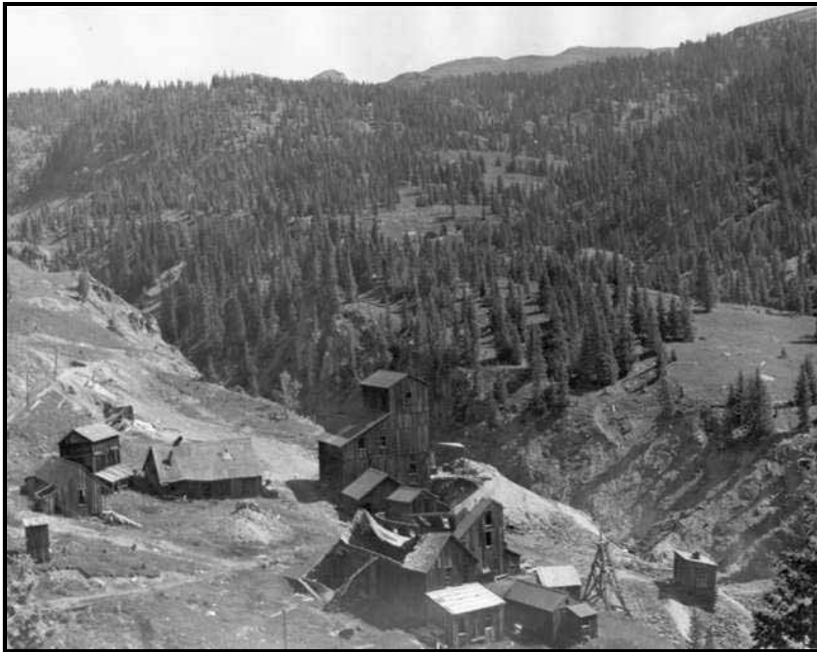
Figure F 5: Although the Silver Ledge Mine, above Chattanooga, was idle and dilapidated by 1920, it represents a well-developed shaft operation. The surface plant consists of multiple buildings added over time, and they are vernacular in design and construction. A shaft house stands at center, a shop is to its left, and the partially collapsed building may be a tram terminal. Source: Denver Public Library, Western History Collection, X-62196.
