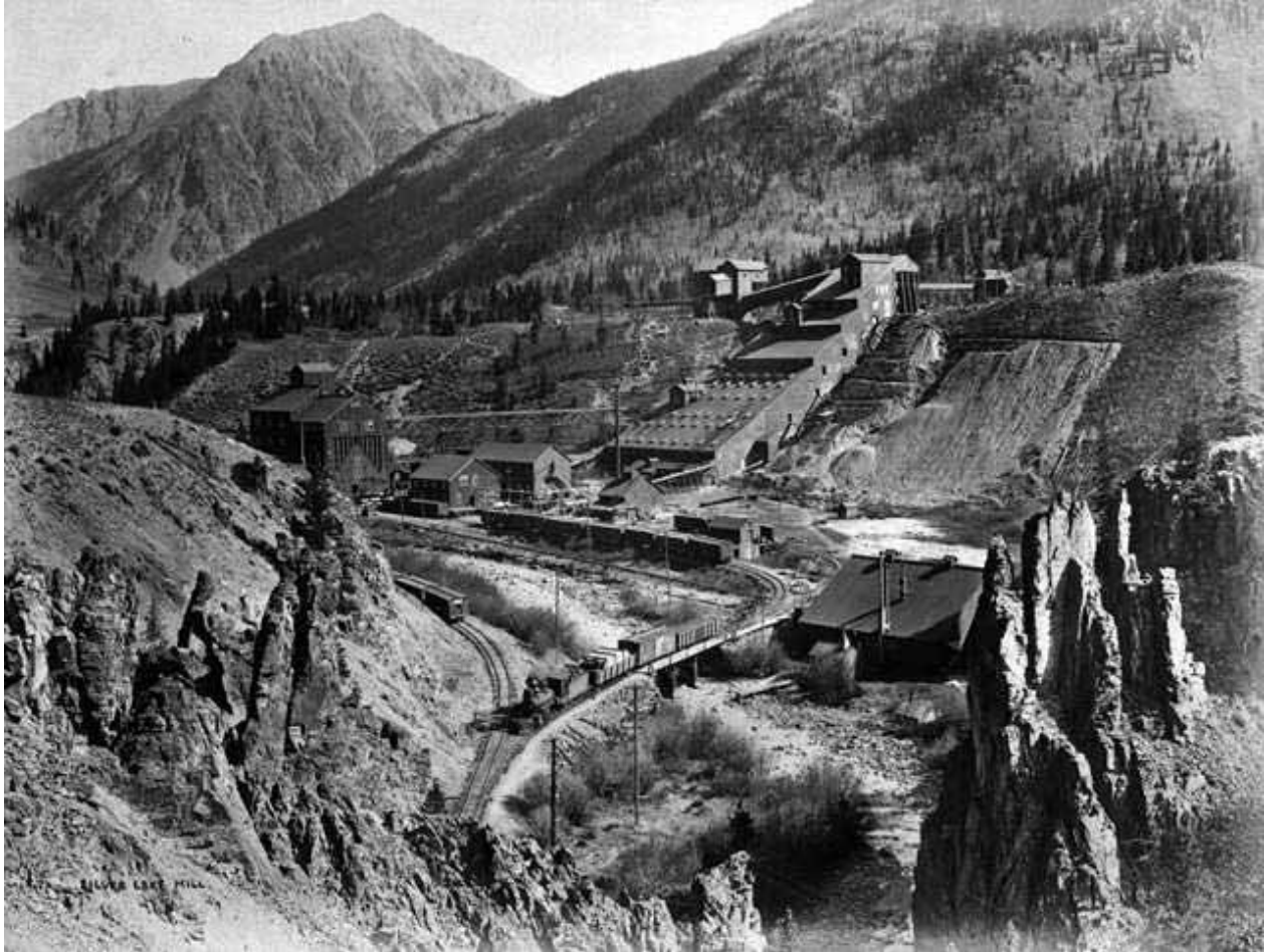
Figure E 30: Edward Stoiber designed the sprawling Silver Lake Mill, built on the Animas River in 1900. Because Stoiber was one of Otto Mears' best customers and invested in Mears' Silverton Northern Railroad, Mears provided the mill with direct rail service. At far left stands the ore bins and tram terminal of a loading station erected during the 1890s, prior to the mill. The small building with tall smokestack at photo-center was an electrical powerhouse, and the complex building to the left of the mill's head was a new tram terminal that received and crushed ore. Note how the mill building fans out to accommodate the increased number of concentration machines for each processing stage. The facility had a capacity of 1,000 tons of ore per day and ranked among the state's largest. In later years, the mill played an important role in the county because it accepted custom ores from independent mines. Source: Denver Public Library, Western History Collection, X 62275.
