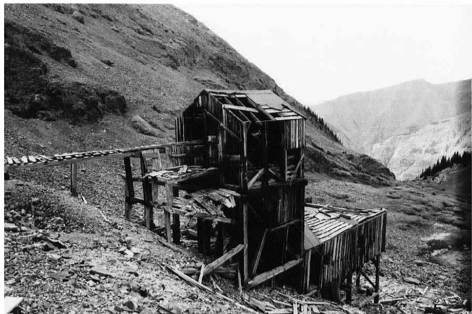
Figure E 36: Peter Orella's tram terminal at the Big Giant Mine still stands. Miners input payrock into the structure from the trestle at left. A second tramway carried North Star Mill tailings down from Little Giant Basin and entered the double doorway in the cupola. The tram mechanism was located in the large room at the structure's bottom. Source: Author.
