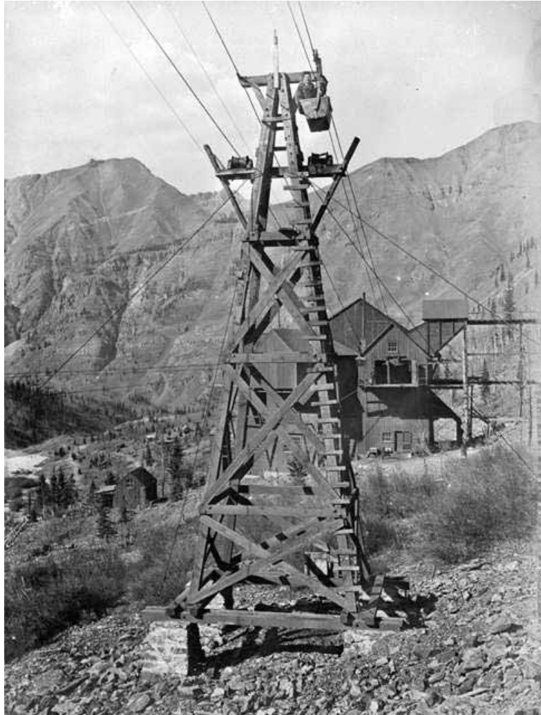
Figure E 78: Aerial tramways played a significant role in the success of mining in San Juan County. They allowed many companies to overcome difficult terrain and ship high volumes of ore from remote locations. Without tramways, transportation costs would have been too high. The photo illustrates the Bleichert system that descended from the Iowa Mine to the mill, background. In the Bleichert system, the buckets coasted over a stationary track cable fixed to the tower top, and were pulled by a second, lower traction cable. Note the cross-member and rollers for the traction cable. The tower is a pyramid type, the most common in the county. Source: Denver Public Library, Western History Collection, X-62249
