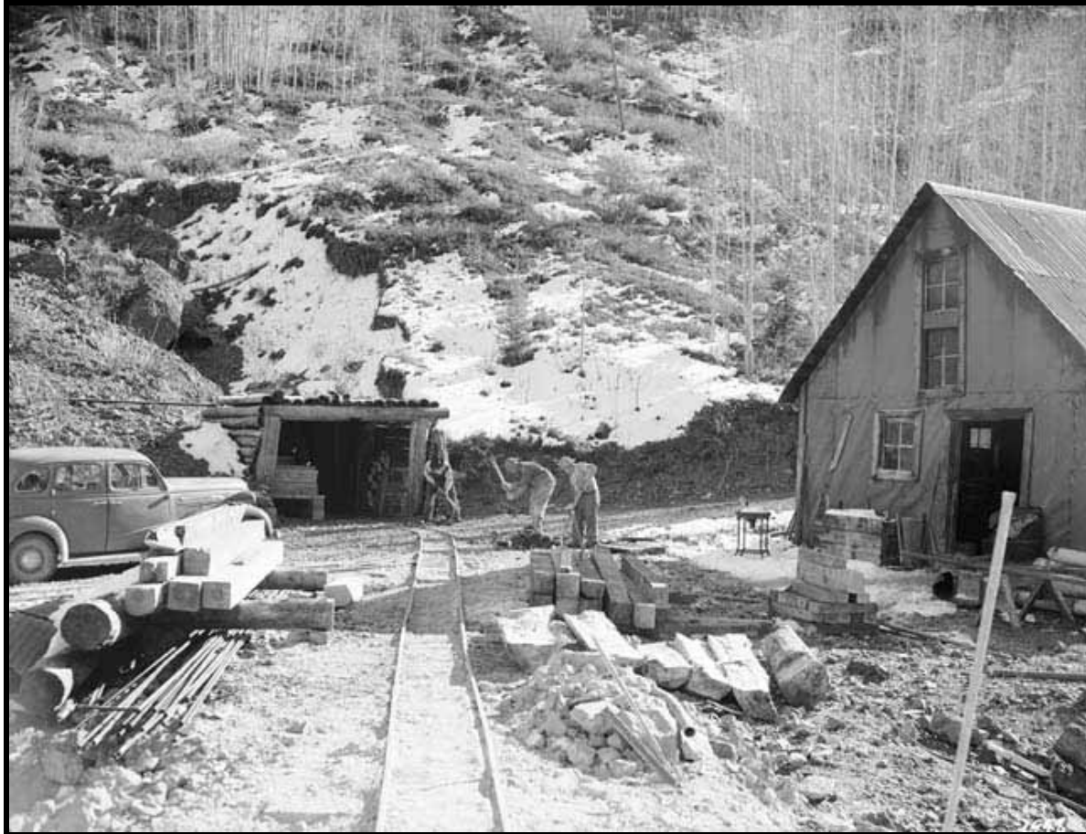
Figure F 3: The unidentified 1930s operation in Cunningham Gulch illustrates a small, tunnel mine. The tunnel is well-developed, and the miners cached timbers and supplies on both sides of a rail line. The building at right is a blacksmith shop and probably houses an air compressor. The building, battered and clad with tarpaper, is characteristic of 1930s vernacular architecture at mines. Source: Denver Public Library, Western History Collection, X6195.
