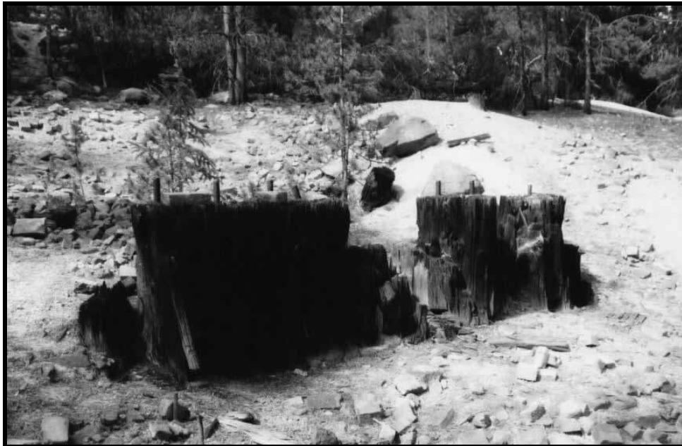
Figure E 88: When a stamp battery was dismantled, the pedestals for the cast iron battery boxes were often left in place. The pedestals consist of timbers on-end and feature anchor bolts on top, and each is around 2 feet wide, 3 feet high, and 5 feet long. Source: Eric Twitty.
