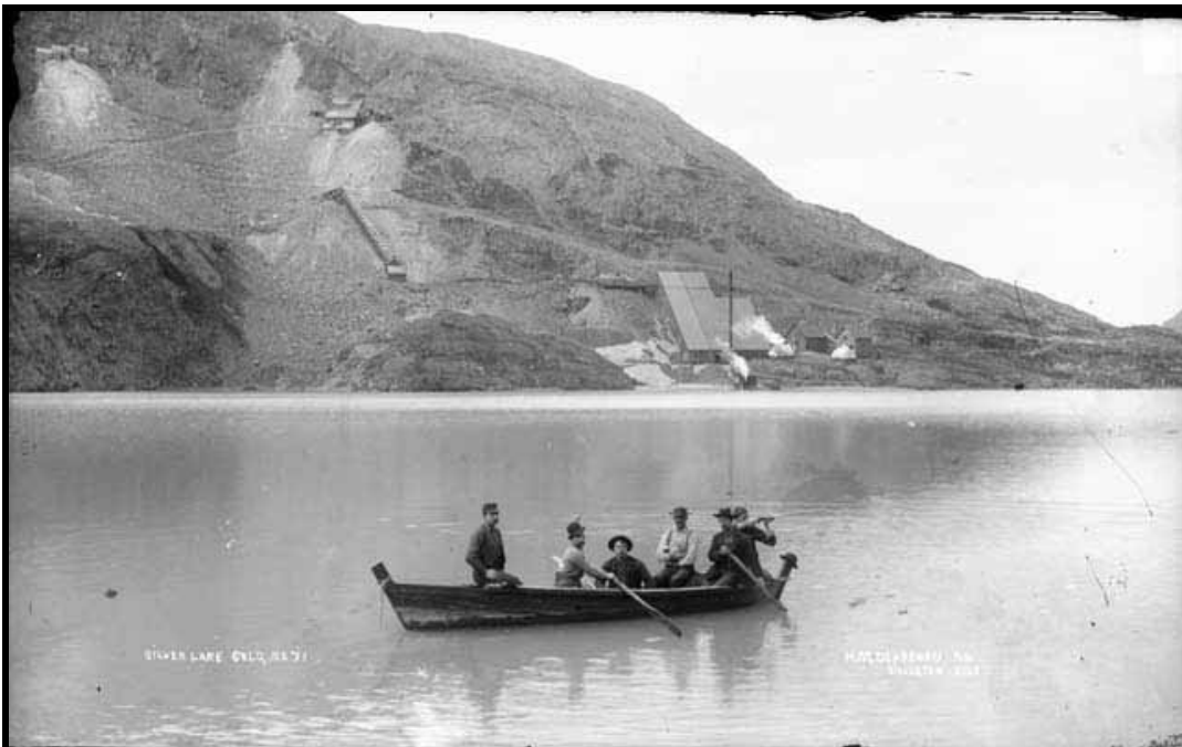
Figure E 23: This northwest view depicts Edward Stoiber's Silver Lake Mine in 1890 or 1891. Stoiber recently finished the mill, center, a boardinghouse adjacent and right, and two shaft houses at upper left. The long chute at left delivered ore from a mid-level tunnel. The skiff floats on Silver Lake, which was a glacial tarn in an austere basin above treeline. The man on the bow is probably Edward Stoiber, and he is accompanied by engineers. Source: Colorado Historical Society, CHS X 7880.
