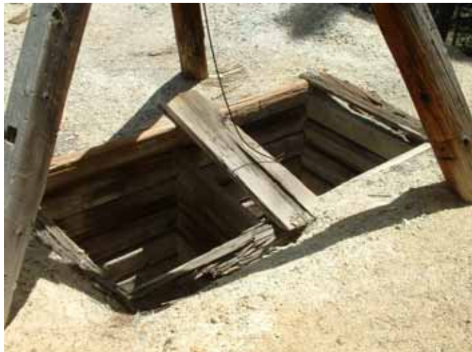
Figure E 44: When intact, shafts often are divided into several compartments for hoisting and egress. The collars are usually timbered to retain loose material, and are flush with the surrounding ground. Intact examples are rare and important engineering resources. Source: Eric Twitty.
