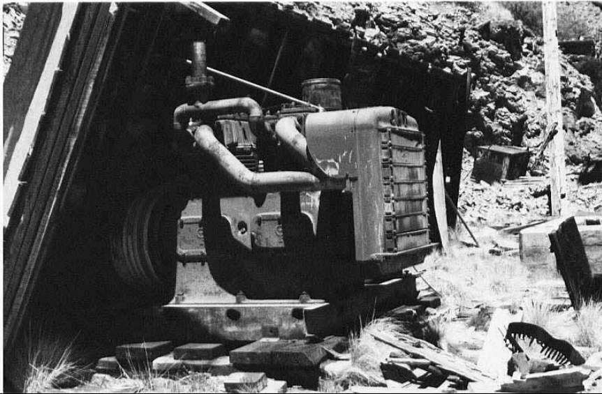
Figure E 72: The V-cylinder compressor, similar to a large engine, became one of the most popular compressor types during the 1930s. Note the foundation. Source: Eric Twitty.
