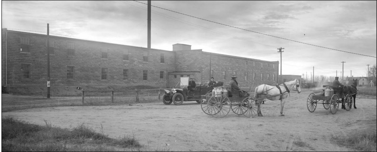
Figure 3. This 22 January 1910 view southeast shows the west wall of the original complex, with the warehouse section to the left, the factory to its right, and the one-story detached office beyond. Based on Sanborn map measurements, the factory was about 115' in length and the warehouse 95'. Courtesy of Western History and Genealogy Department, Denver Public Library, Denver, Colorado, L.C. McClure photograph MCC-3446, 22 January 1910.
