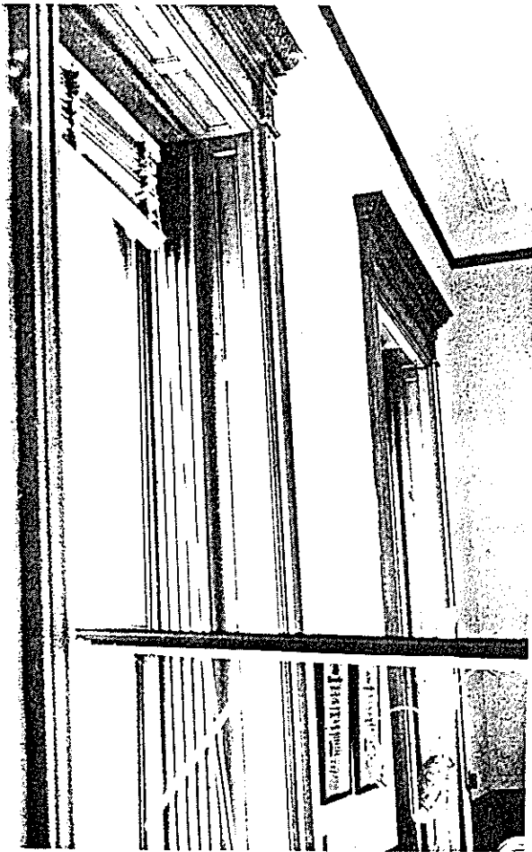
Figure 5. The interior storm window was designed to fit within the existing wooden jamb. The large size of the windows necessitated the use of operable storm panels, intersecting at the historic meeting rail. Here the lower storm panel is in an opened position for cleaning. Photo: Charles E. Fisher
