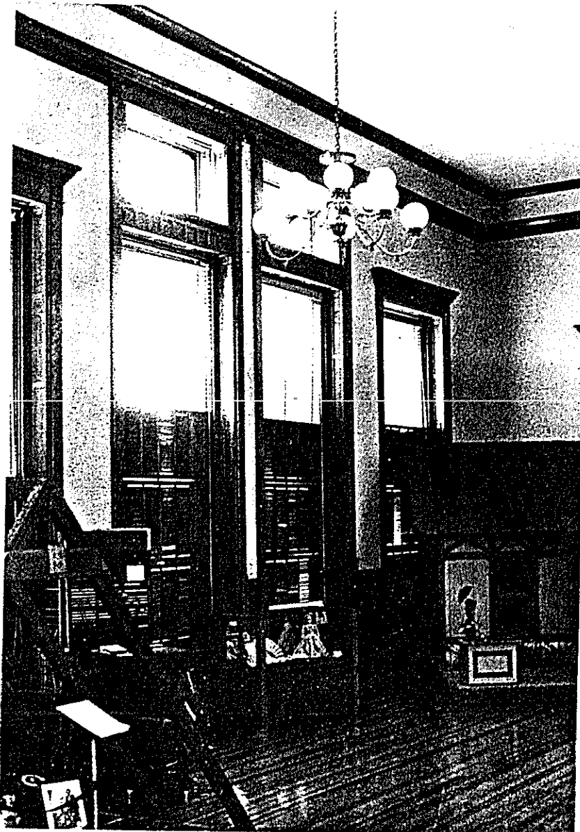
Figure 1. The monumental windows are elegantly detailed on the interior and contribute to the grandeur of the spacious banking rooms. The original interior shutters are still being used for comfort and light control. Photo: Charles E. Fisher
