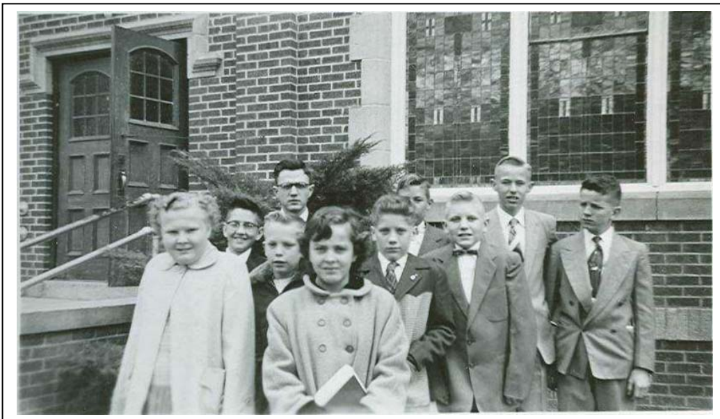
Note original doors on main entrance- windows remain, though the doors have been covered with large metal panels. Wood panels on lower portion are visible on inside. Image courtesy of the Eaton United Methodist Church
